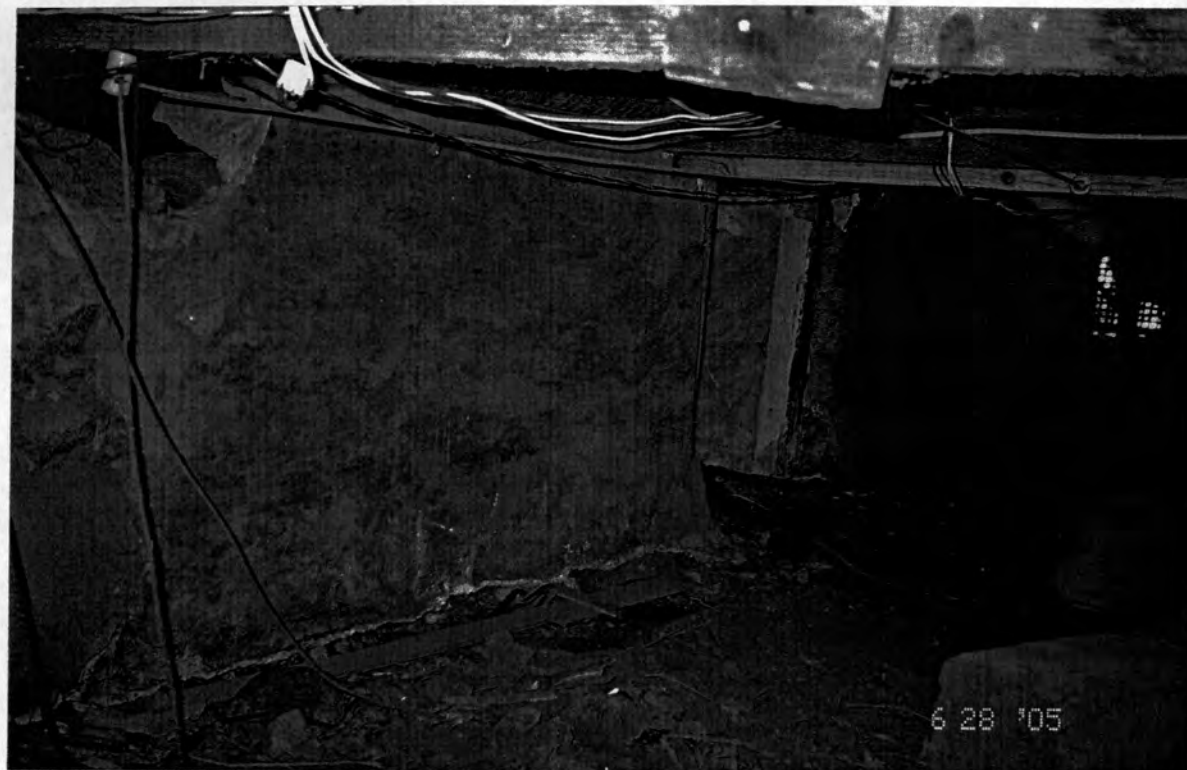
THICK LIME CEMENTED STONE FOUNDATIONS
