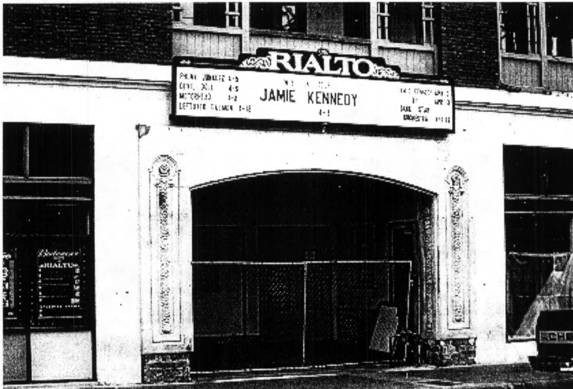
PHOTO #1: Theater entrance on Congress Street, looking south
