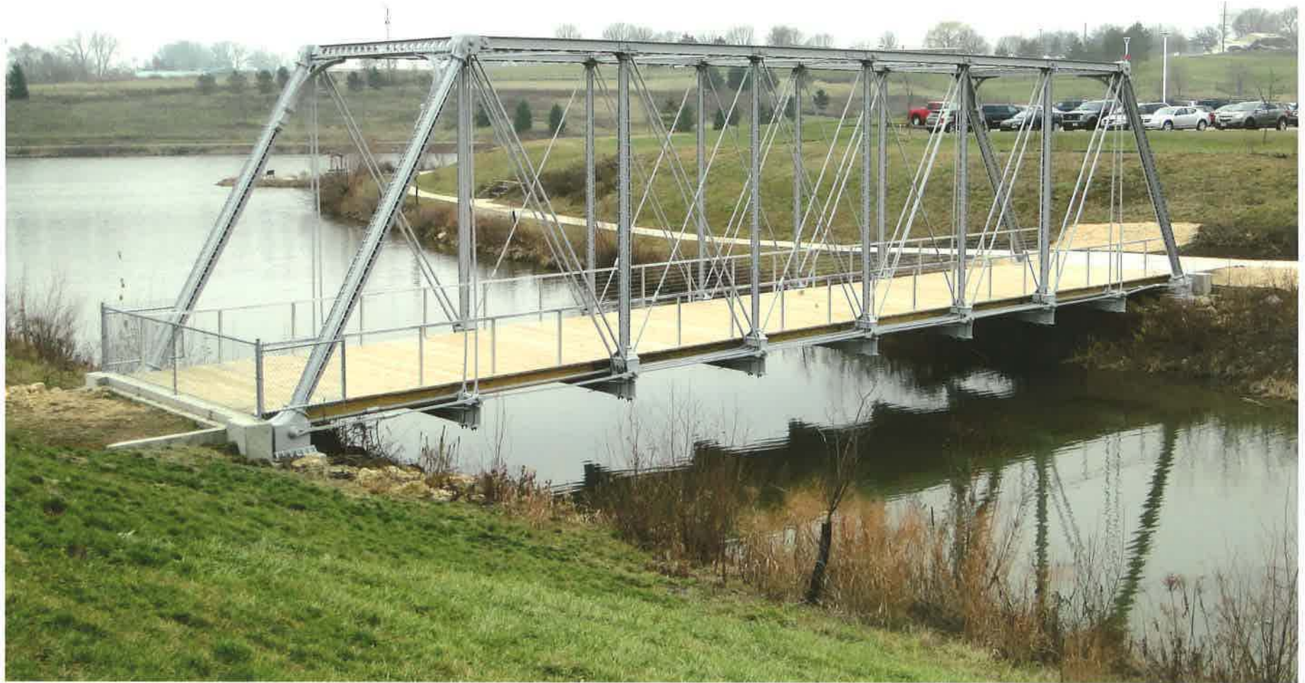
Dunleith and Dubuque Bridge (Dubuque County, IA)
