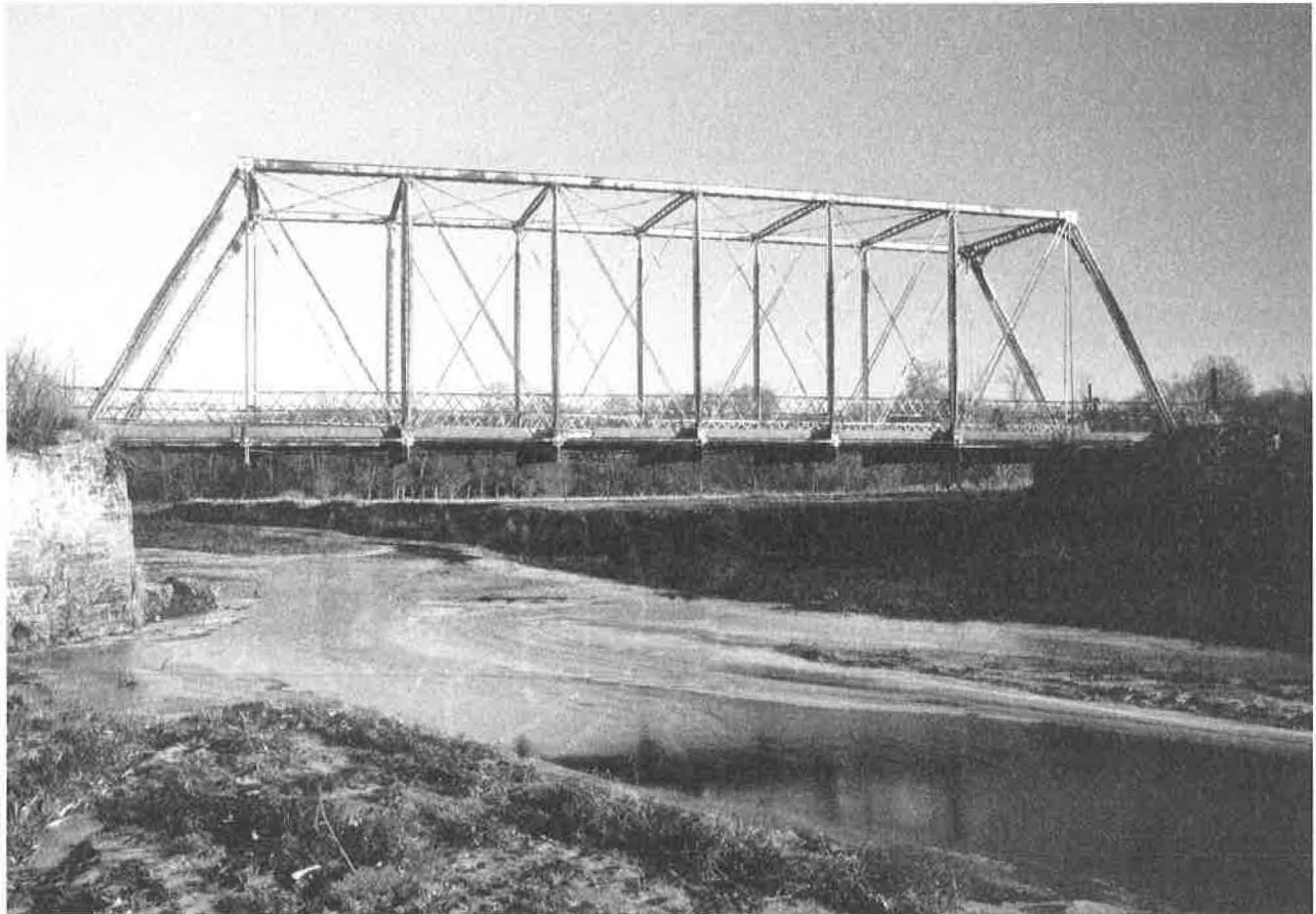
Fig. 2 White Water Creek Bridge, 1989 (from collection of the author).
