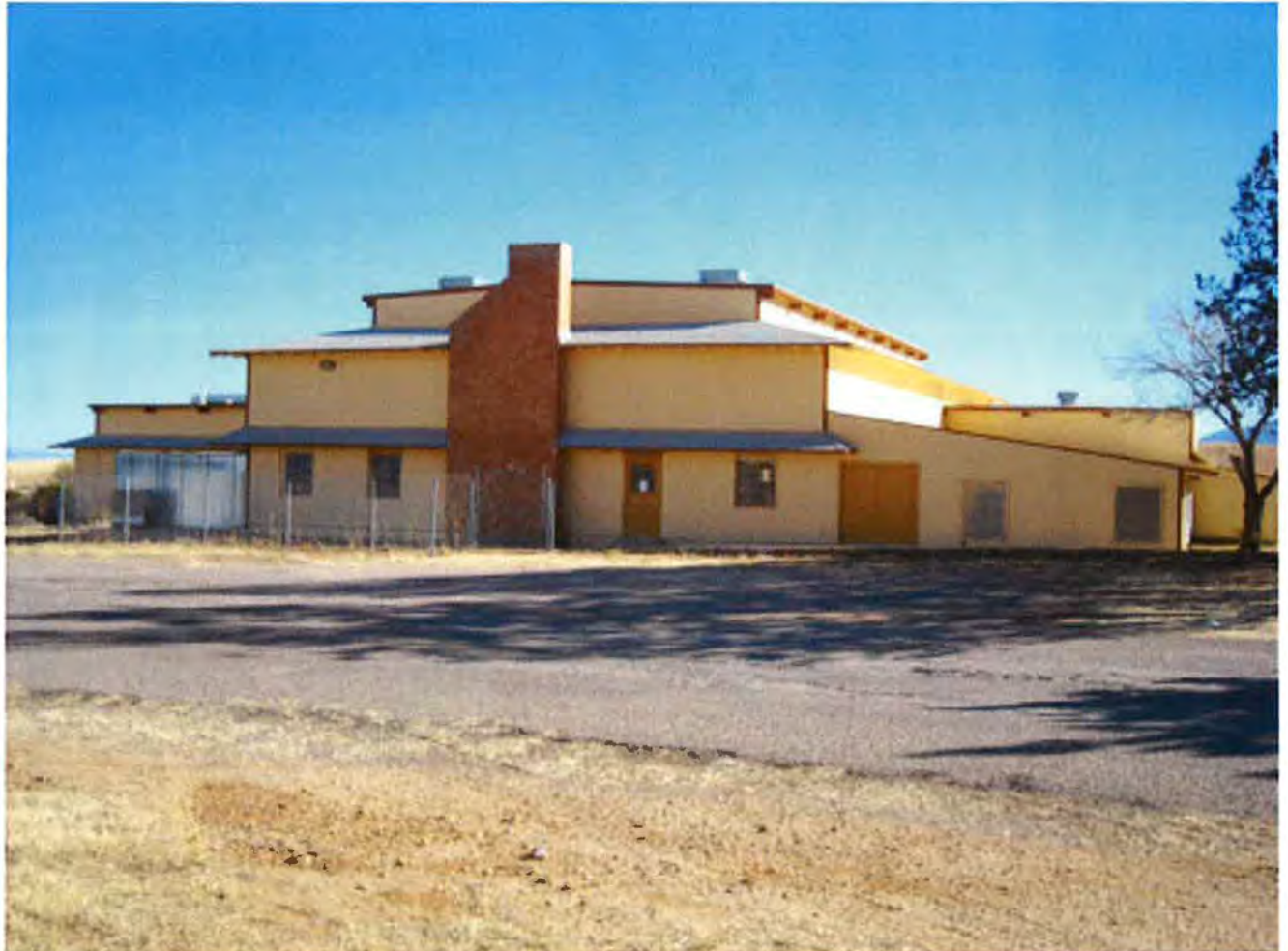
Photograph 5. North elevation of MVOC. View facing south.
