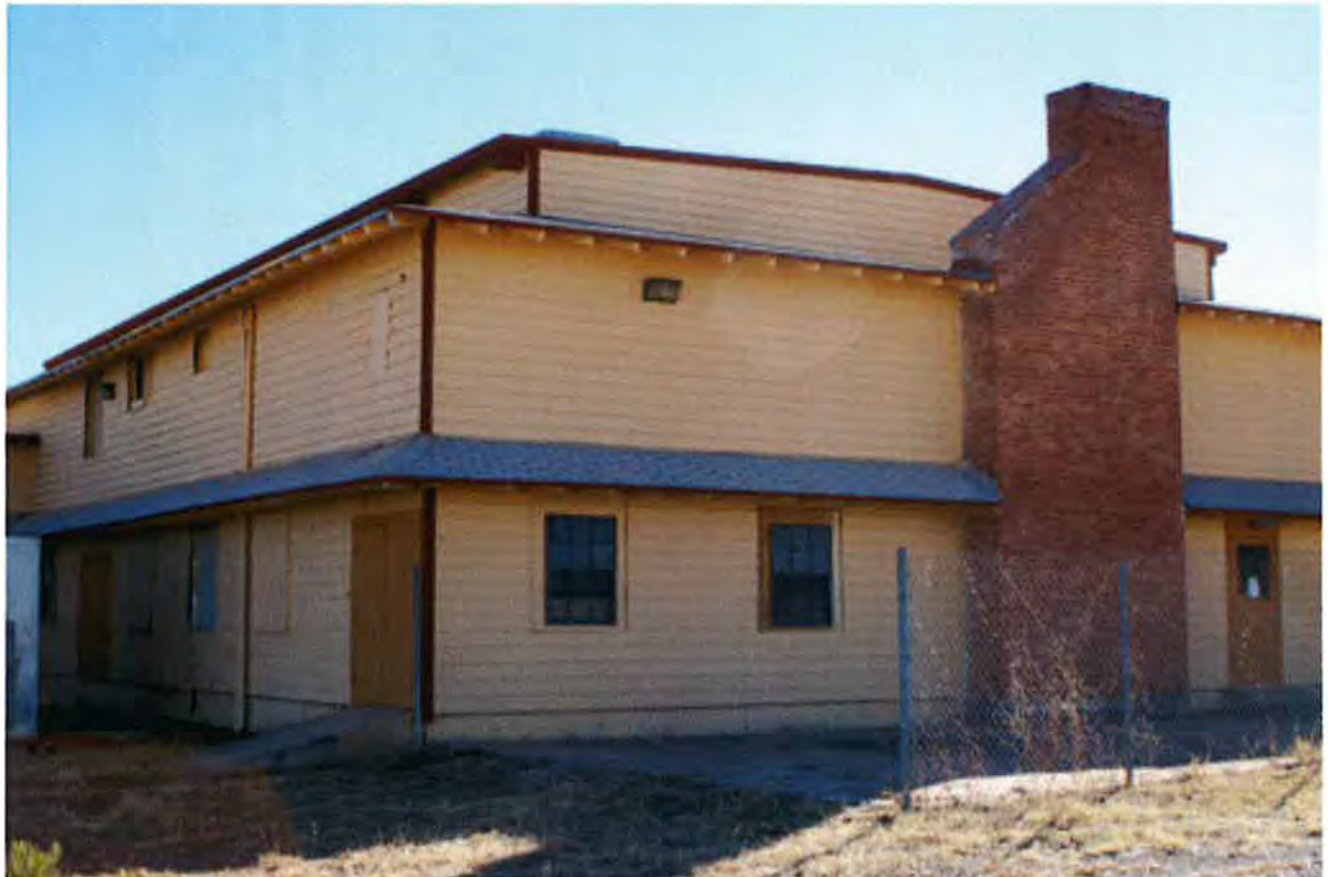
Photograph 6. Detail of north elevation. View facing southwest.
