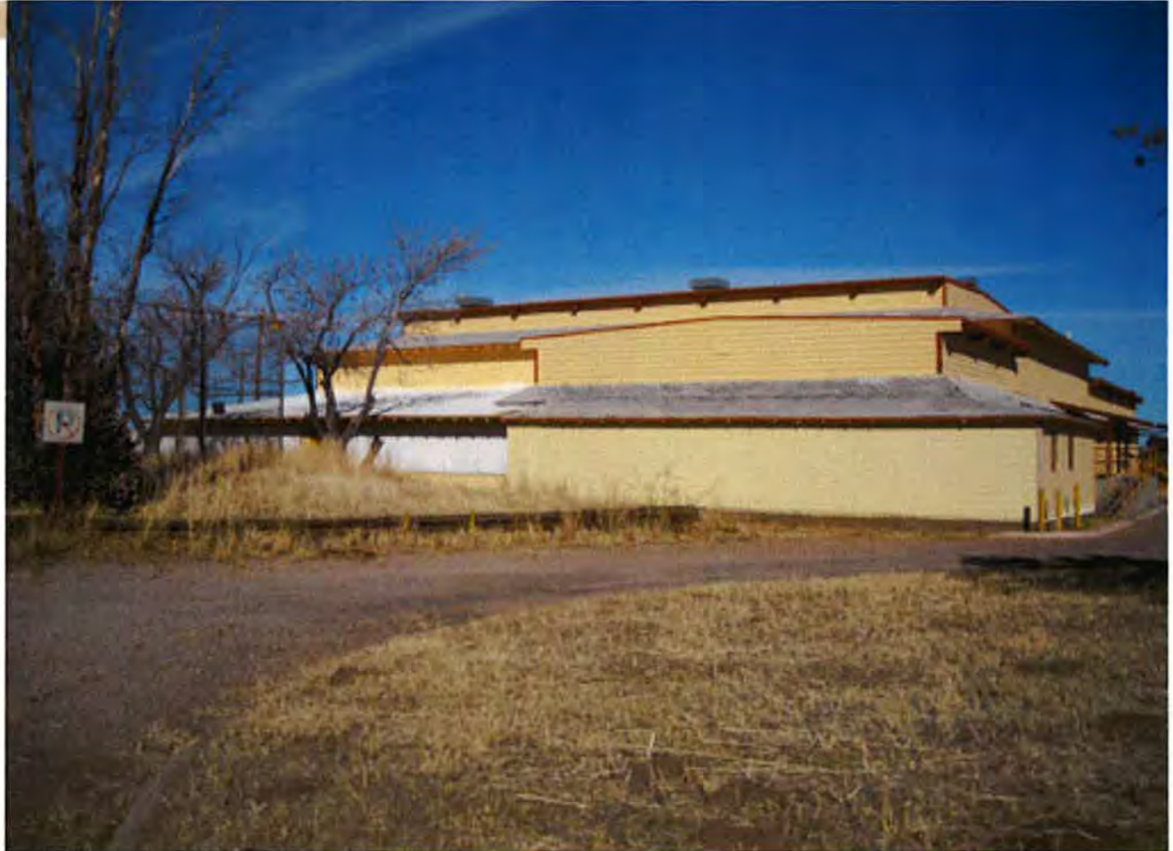
Photograph 4. West elevation of MVOC. View facing northeast.
