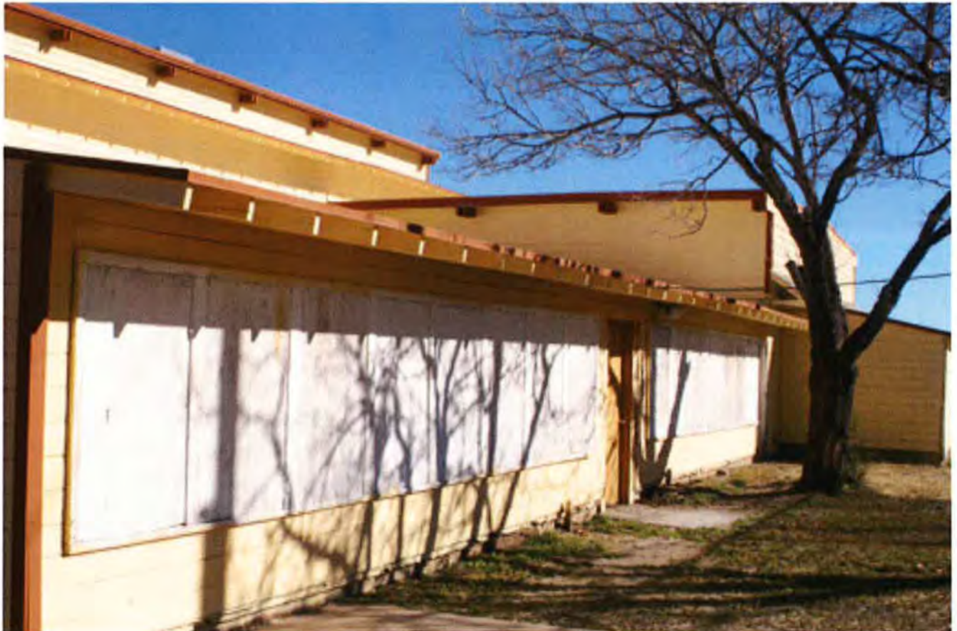
Photograph 7. Detail of west elevation. View facing south-southeast.
