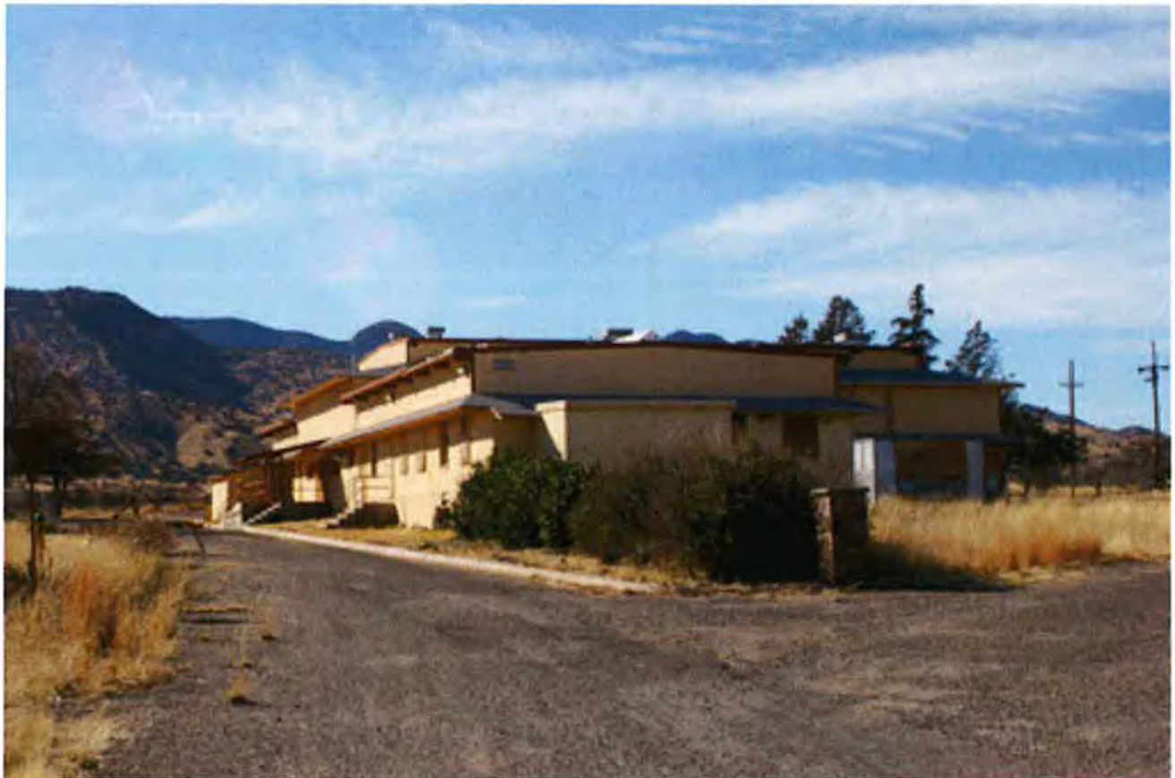
Photograph 1. Main façade (south elevation) and East elevation of MVOC. Stone pillar in foreground and driveway leading to circular drive to left. View facing northwest.
