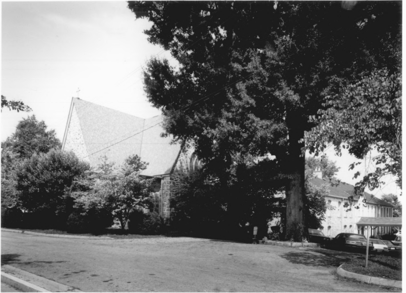
ST. GEORGE'S EPISCOPAL CHURCH GRIFFIN/SPALDING COUNTY, GEORGIA 3 OF 11
