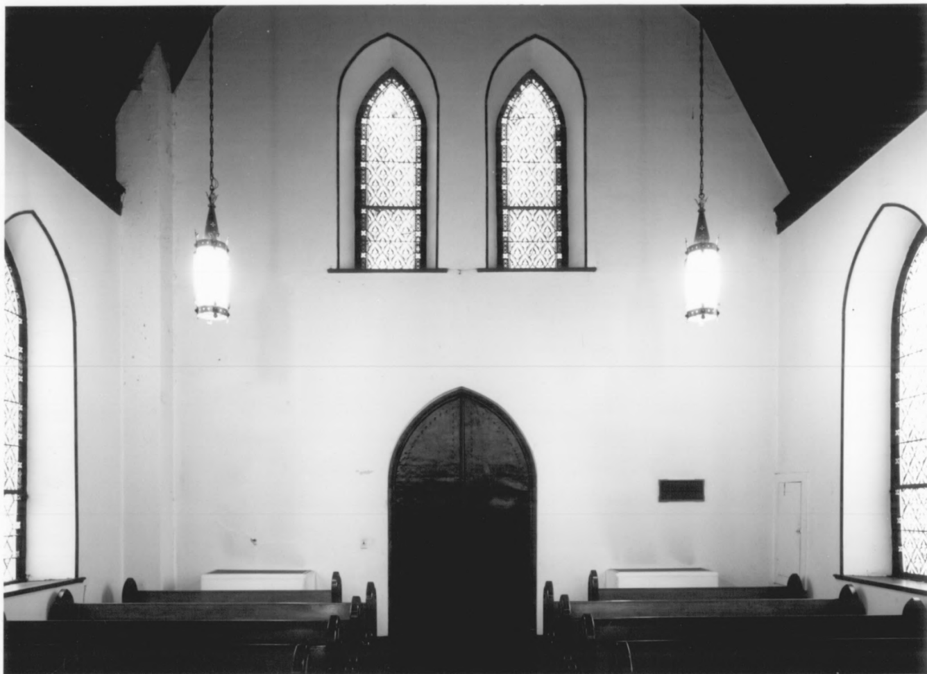
ST. GEORGES EPISCOPAL CHURCH GRIFFIN/SPALDING COUNTY, GEORGIA 7 OF 11
