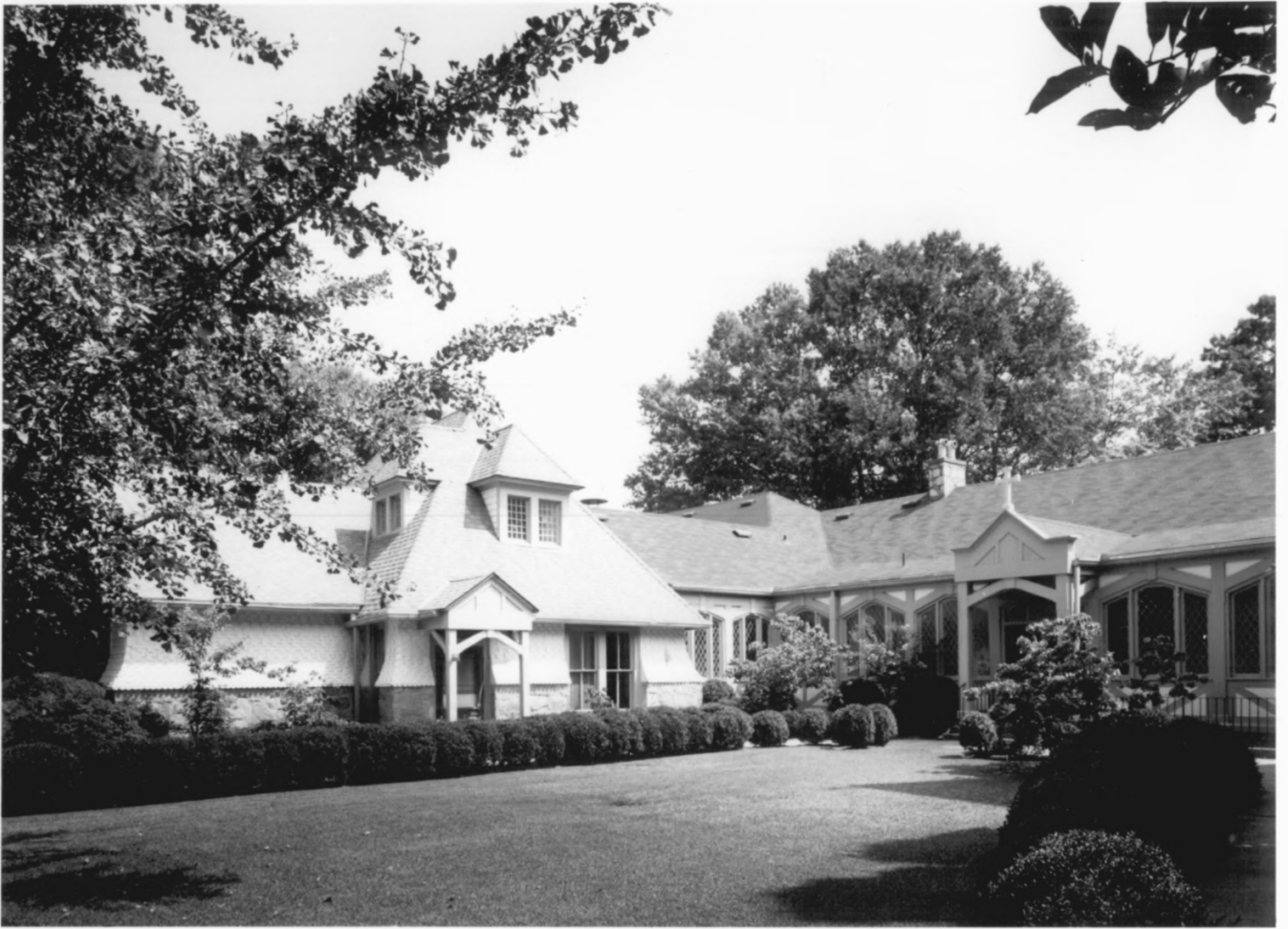
ST. GEORGE'S EPISCOPAL CHURCH GRIFFIN / SPALDING COUNTY, GEORGIA 2 OF 11
