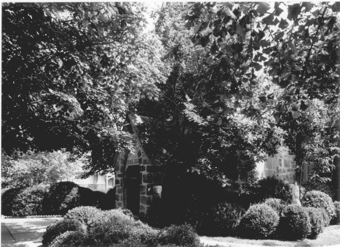
ST. GEORGE'S EPISCOPAL CHURCH GRIFFIN/SPALDING COUNTY, GEORGIA
