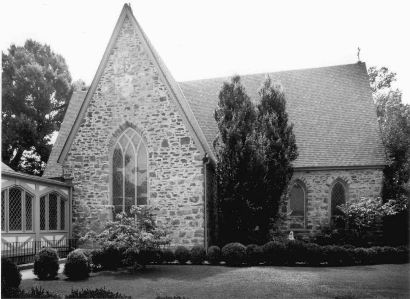
ST. GEORGE'S EPISCOPAL CHURCH GRIFFIN / SPALDING COUNTY, GEORGIA 1 OF 11
