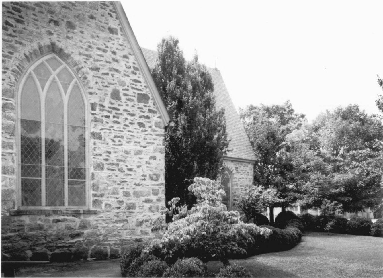
ST. GEORGE'S EPISCOPAL CHURCH GRIFFIN / SPALDING COUNTY, GEORGIA 11 of 11
