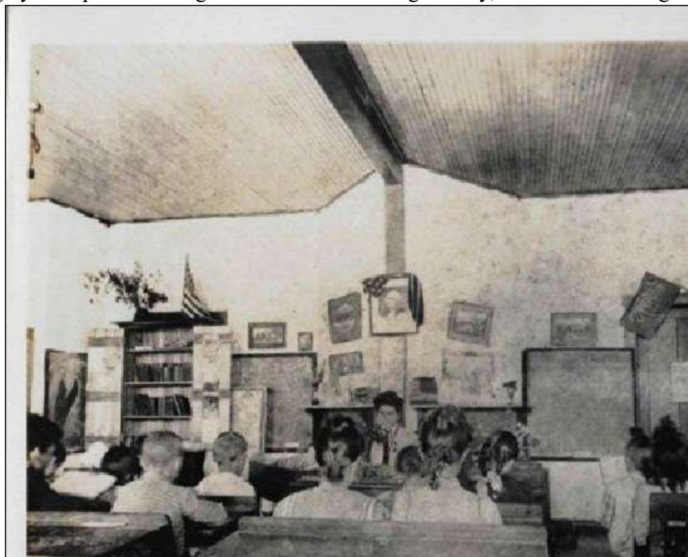
Figure 4: Olympia Mill School, first floor classroom, n.d.
