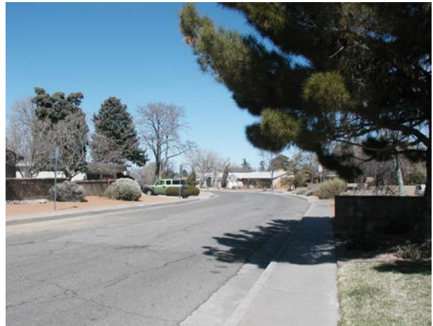
Photos 2. Stanford Drive looking north.
