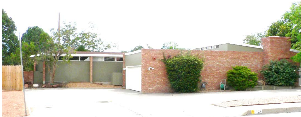
Photo 22. Contemporary-style Ranch House at 1428 Stanford Drive.
