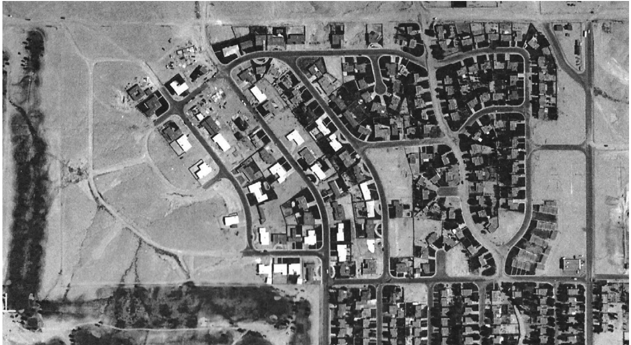
Figure 3. Vista Larga Subdivision under construction, 1955. Girard Boulevard is seen at right, with one of the neighborhood's earliest commercial buildings, Rhodes Supermarket. The Lobo Addition is located south of Hannett Avenue.
