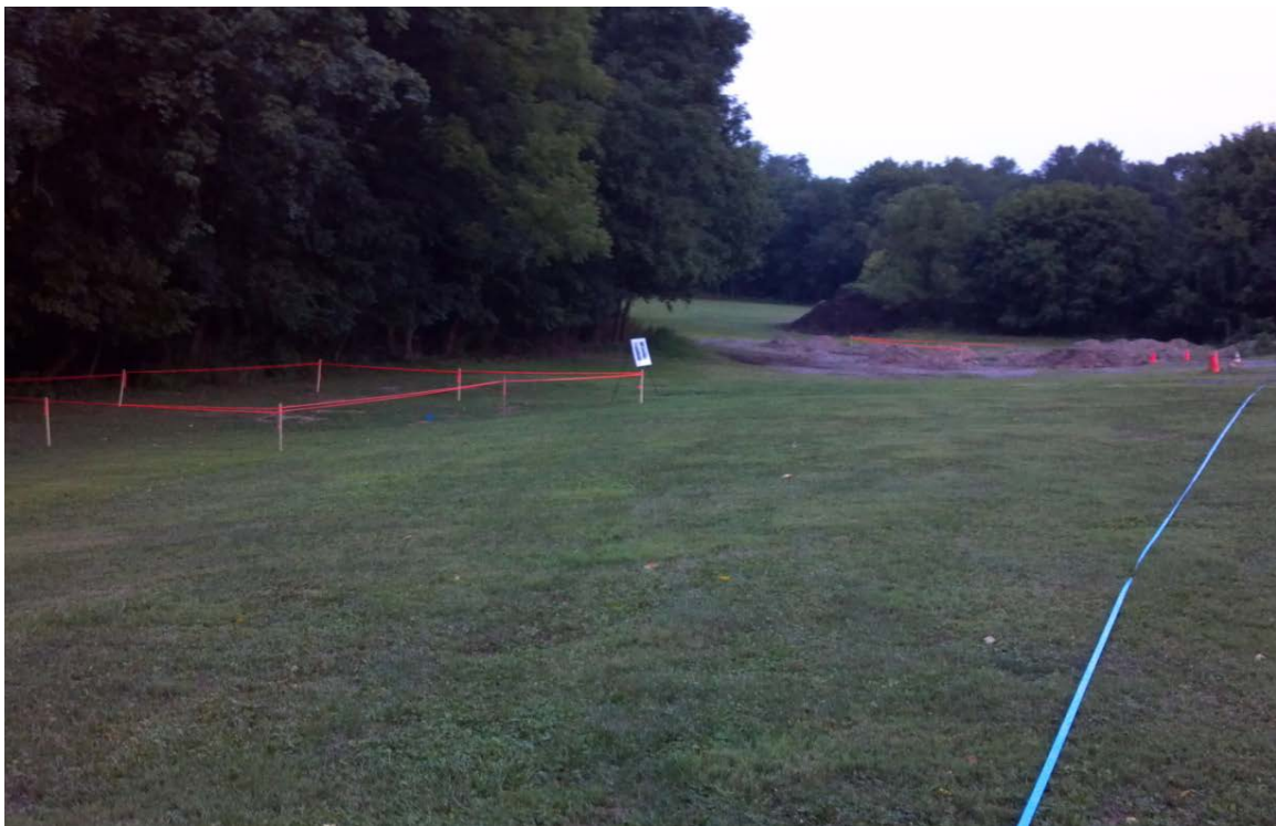
Photograph 6. View along the buried section of the raceway (blue tape) showing the locations of the graining mill site (foreground) and the stamping mill site (background), looking southeast.
