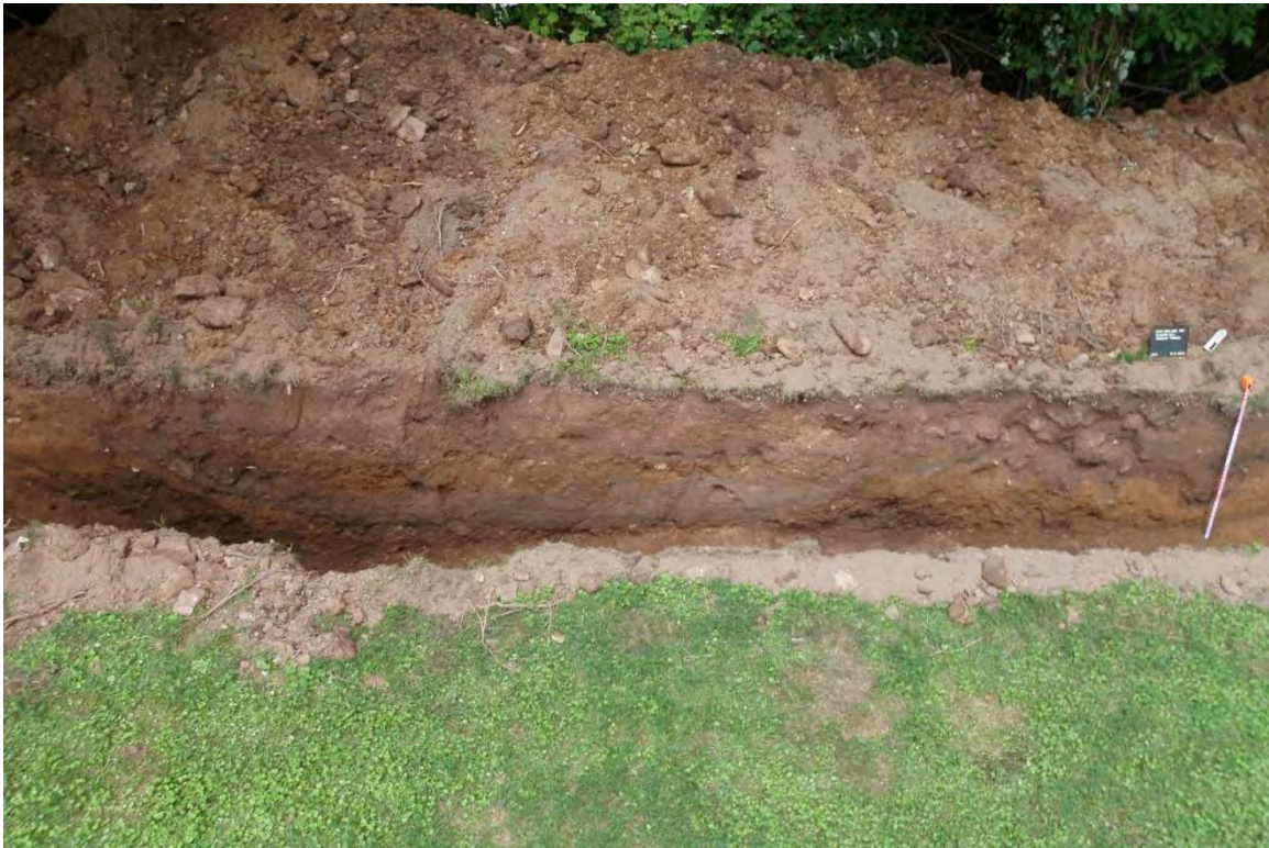
Photograph 5. View of a buried section of the raceway southeast of Rapps Dam Road as exposed in a trench cut, looking northwest.
