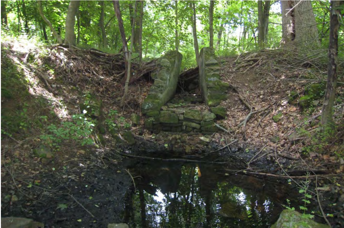
Photograph 3. View of a post-Continental Powder Mill sluice gate and possible wheel pit at the location of the ruins of Rudy's Powder Mill, looking west. A tailrace runs back to French Creek from this location. The primary raceway that runs to Rapps Dam Road is to the south.
