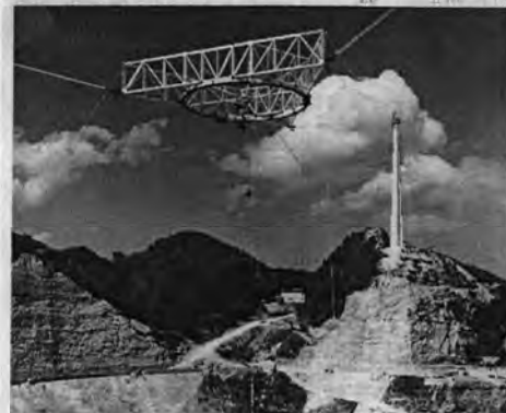
Fig. 34 Raising the triangular platform, February 21, 1963.
