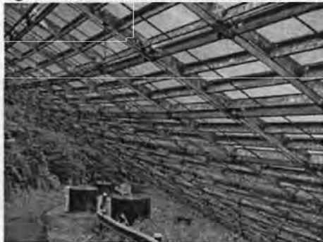
Fig. 39. Aluminum network that holds the "dish".
