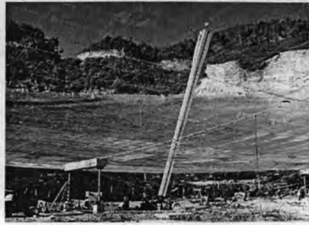
Fig. 35 August 14, 1963, the 430-MHz line feed is lifted.
