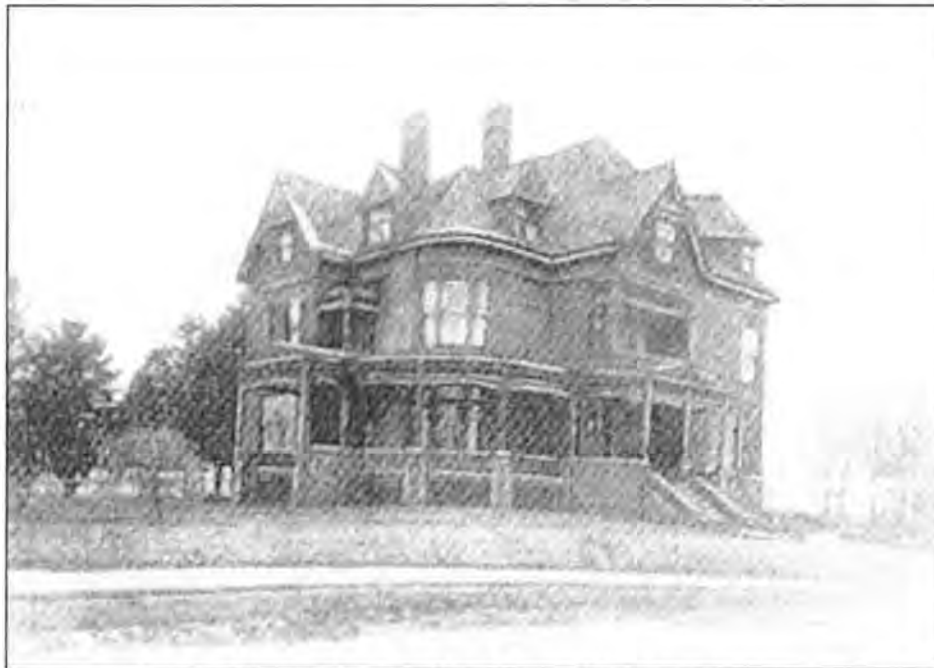
Figure 24: L. C. Bissell House, 900 3rd Street West, 1897, view southwest ( Souvenir Gems of Dubuque , 1897)
