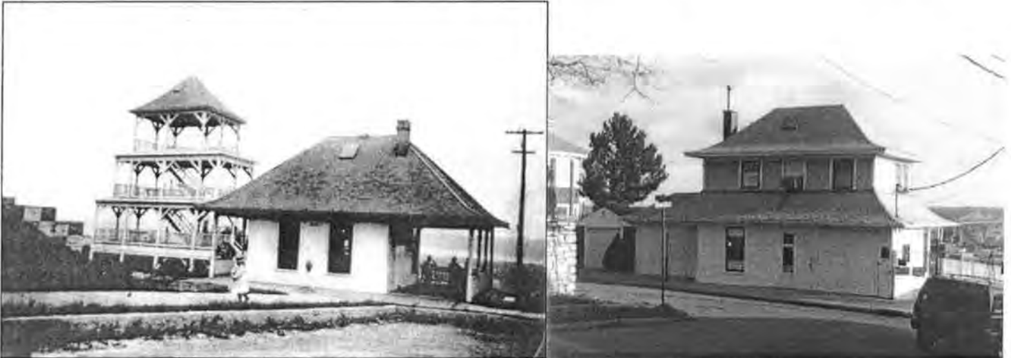
Figures 13-14: Head of elevator, c.1915 (left) and recent view (right) (Center for Dubuque History, Loras College; Photo by J. Jacobsen, April 2005)
