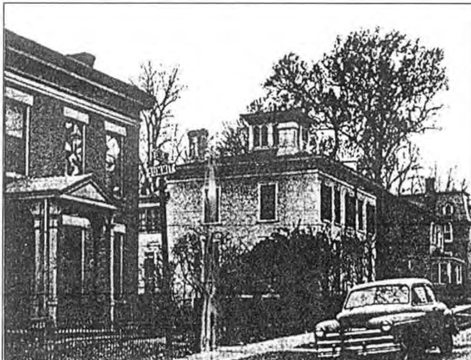
Figure 32: 710, 732, 760 and 788 Fenelon Place, view southwest (Dubuque Telegraph-Herald Staff Photo, December 15, 1957)
