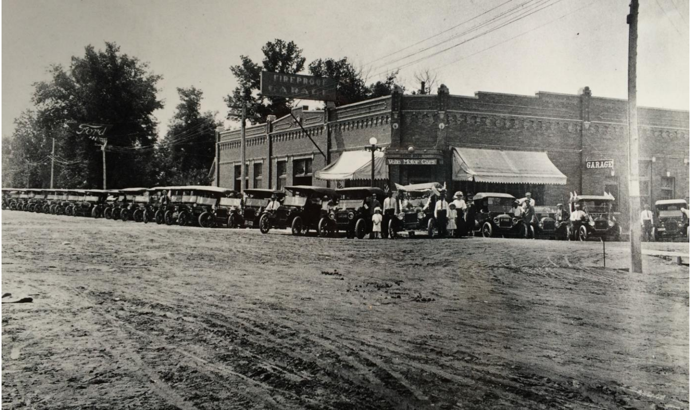
Figure 8: 124 E. 11 th Street, Kopac Garage. Source: Schuyler Museum Archives.
