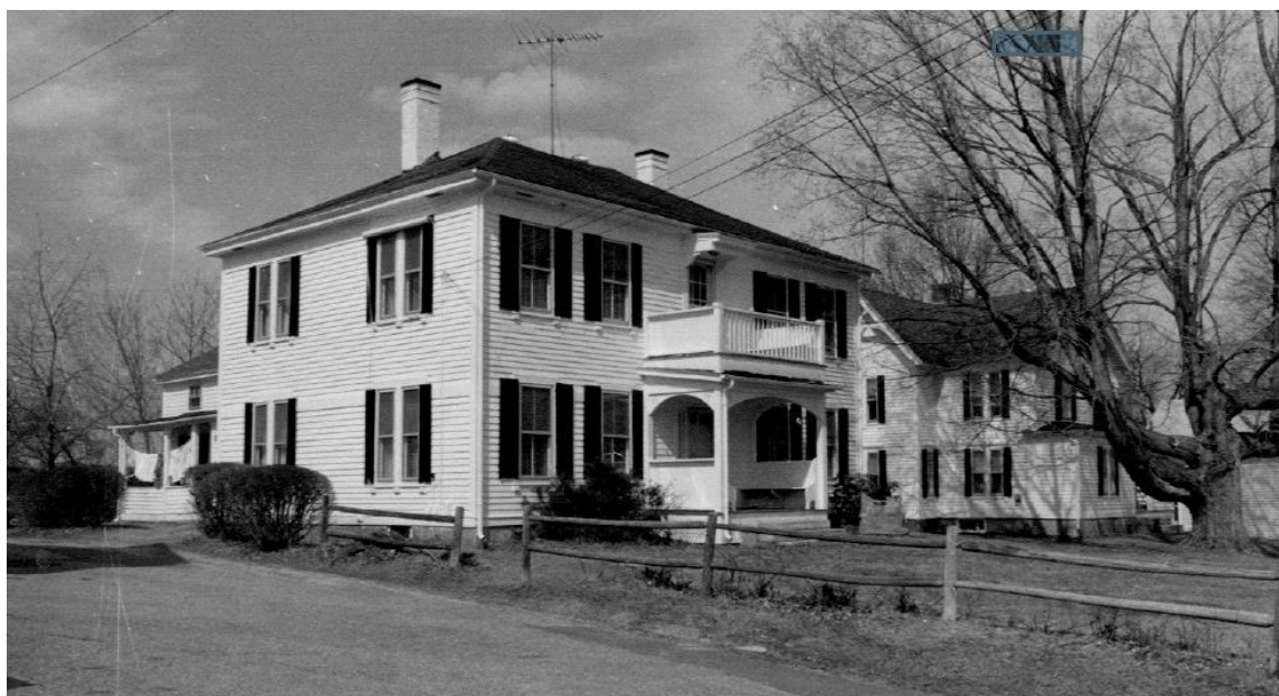
Figures 8.21 & 8.22: Moses Barnes House in the 1890s (top) and 1981 (bottom). Top photograph from the collection of the Pearl L. Crawford Memorial Library in Dudley; used with permission. Both reproduced in DUD.52 (MHC inventory form).
