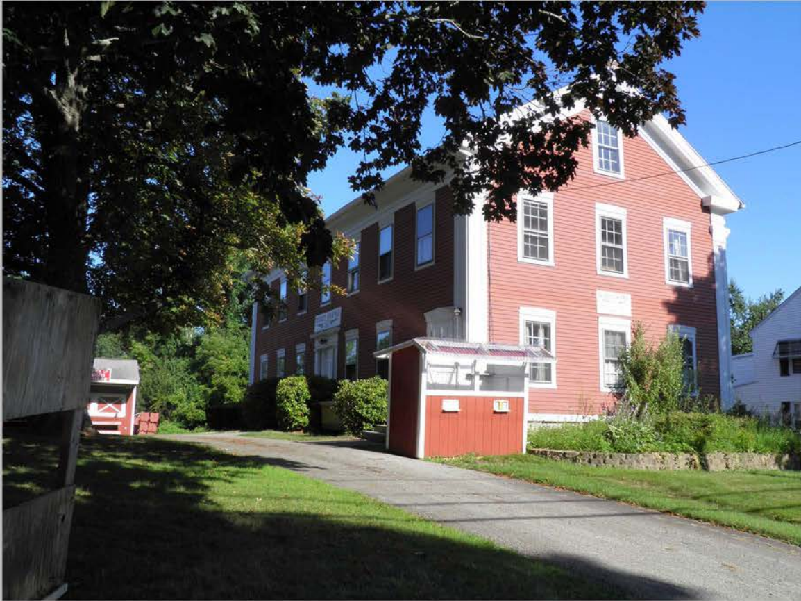
9. Center School/Washington Hall, 139 Center Road, façade and eastern end, looking northwest.
