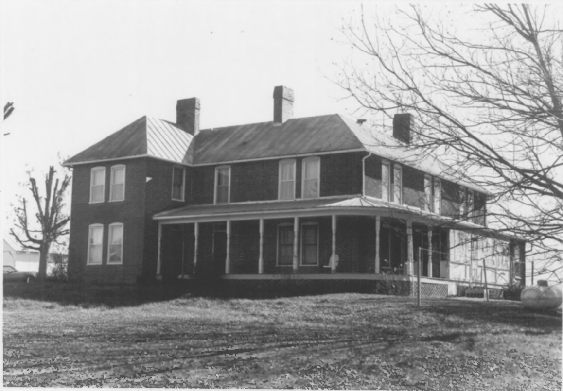
Davis, James R., House, Blount Co., TN, Photo 1 of 10
