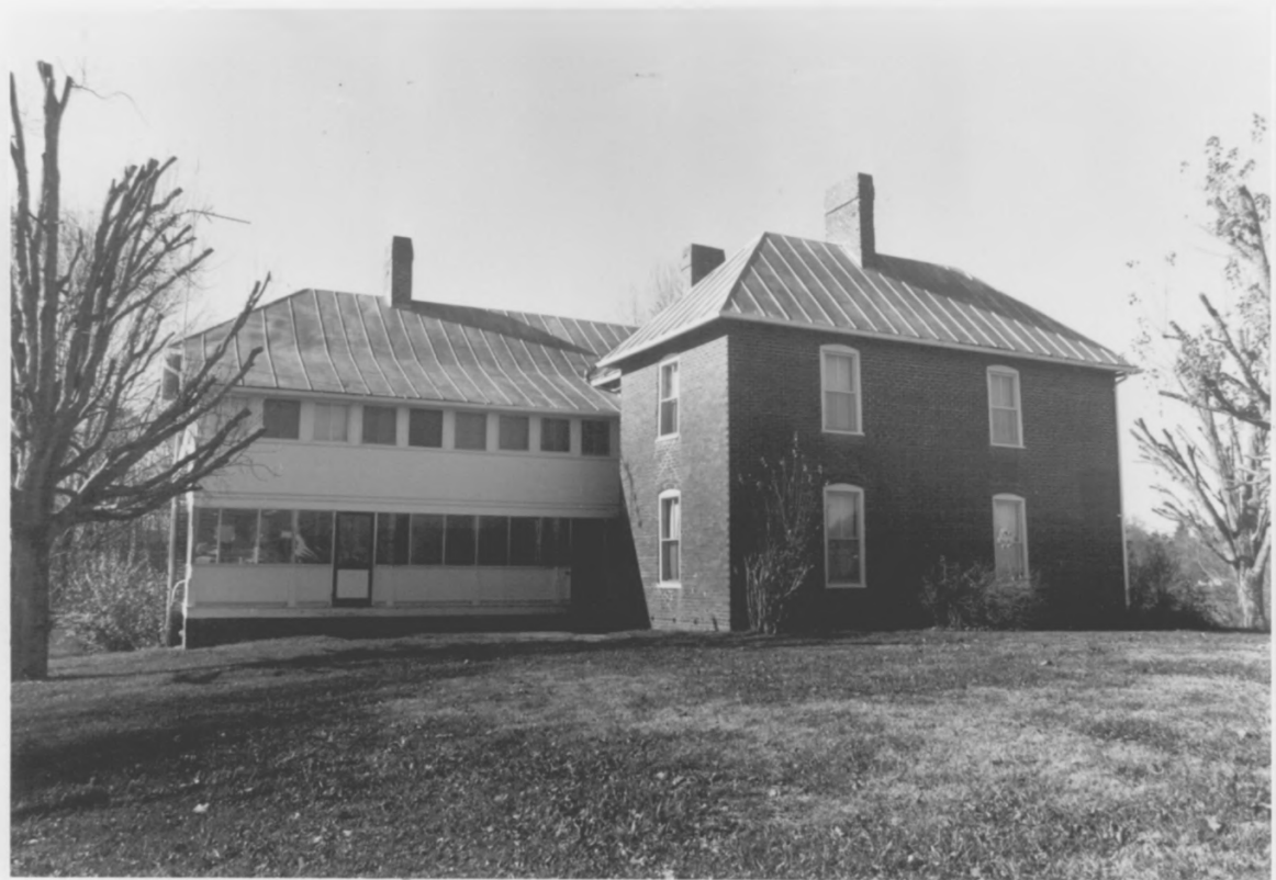
Davis, James R., House, Blount Co., TN, Photo 3 of 10
