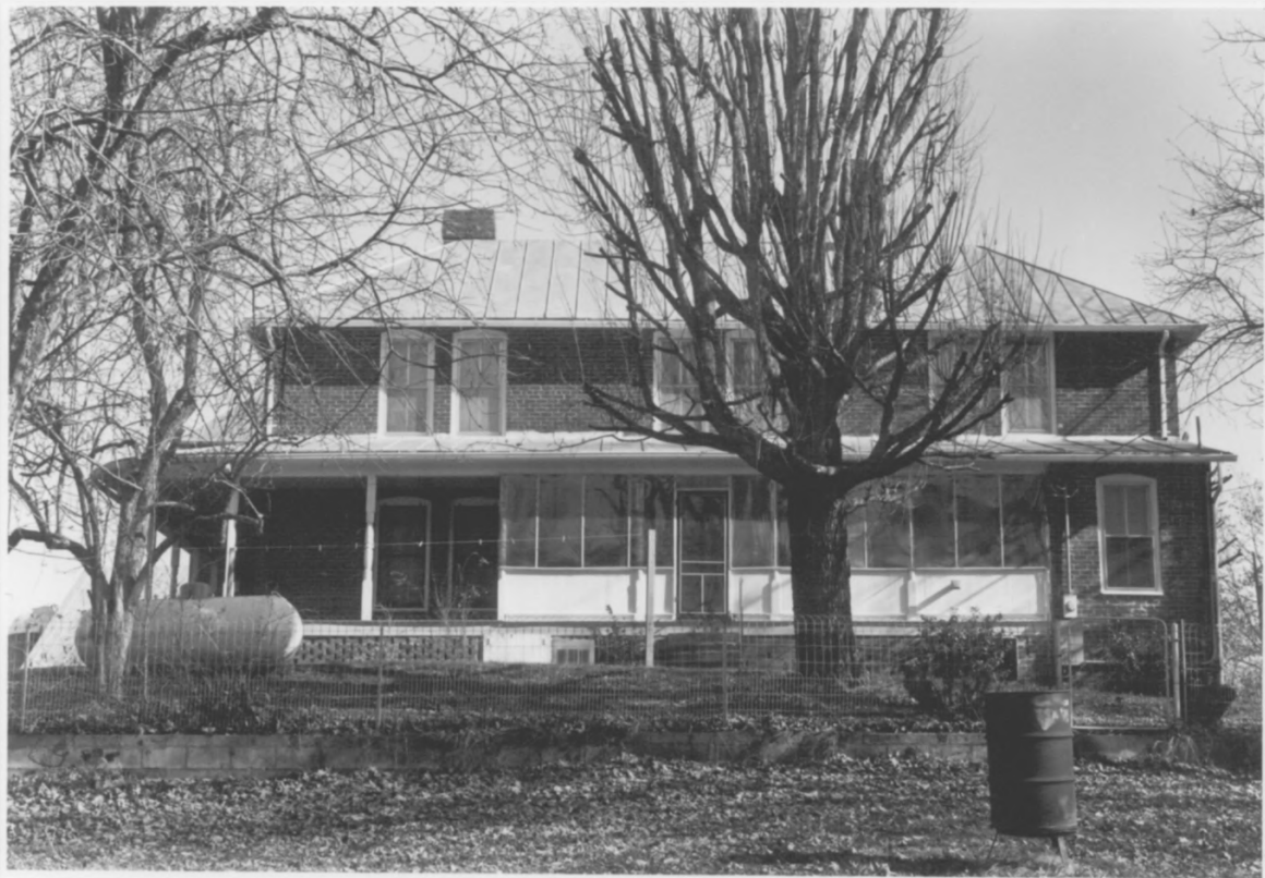
Davis, James R., House, Blount Co., TN, Photo 2 of 10
