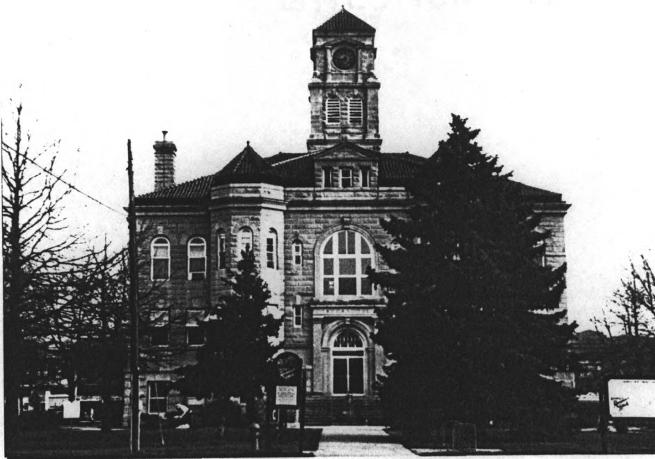
Appanoose County Courthouse (south elevation)
