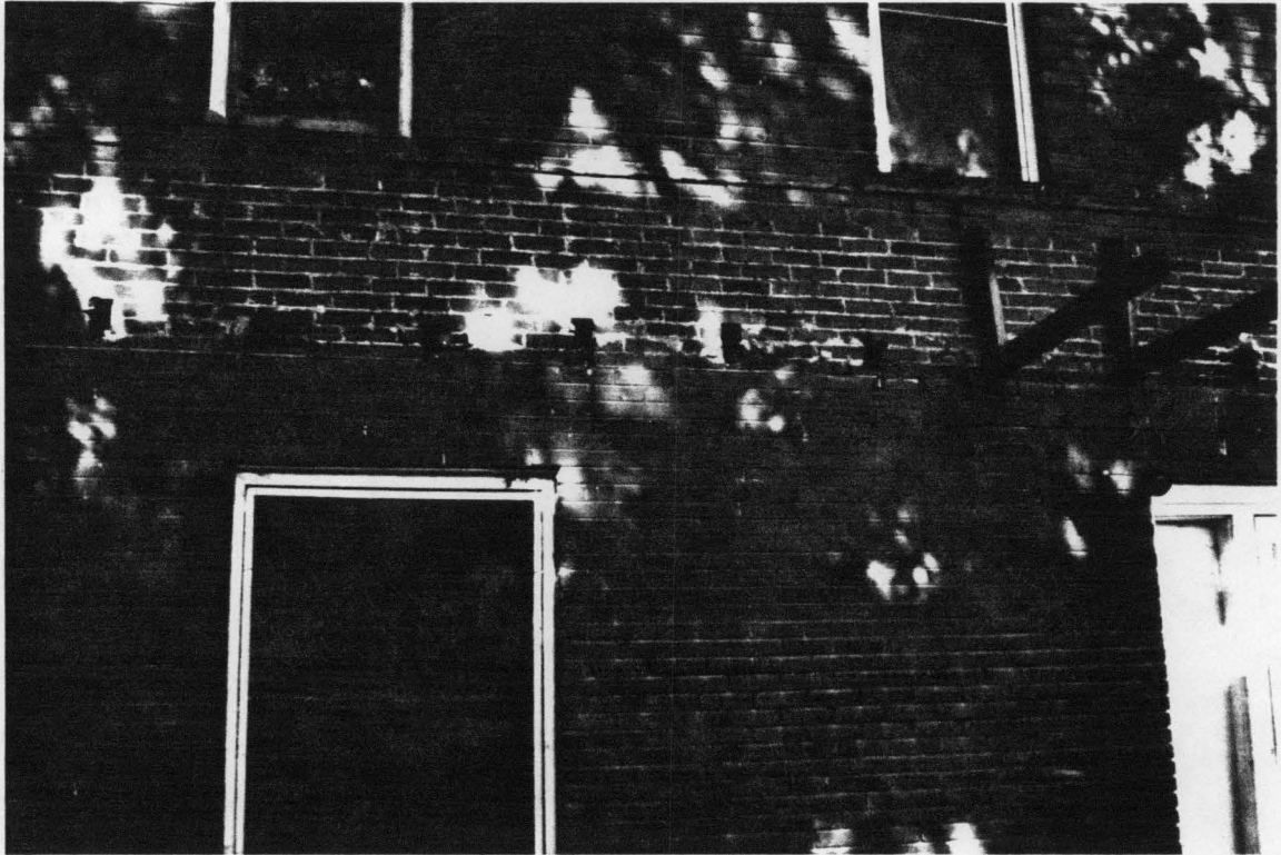
DETAIL OF REMOVED PORCH
