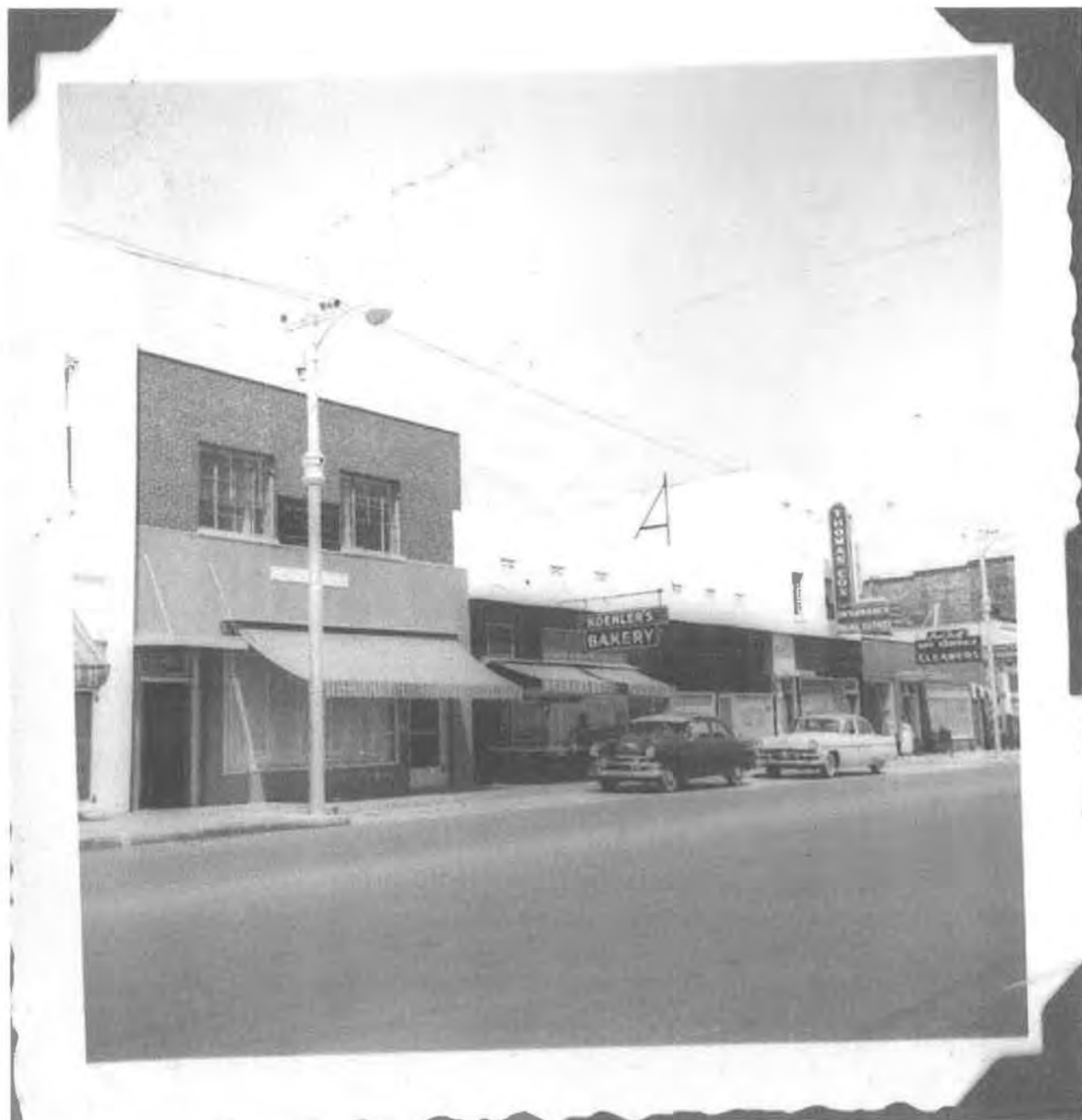
Koehler Buildings at 709, 711, and 713 Main Street, c.1955. (Photo courtesy of the North Little Rock History Commission.)
