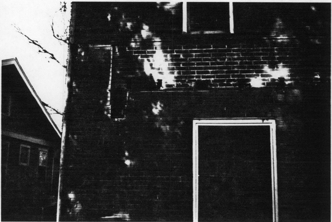
DETAIL OF REMOVED PORCH
