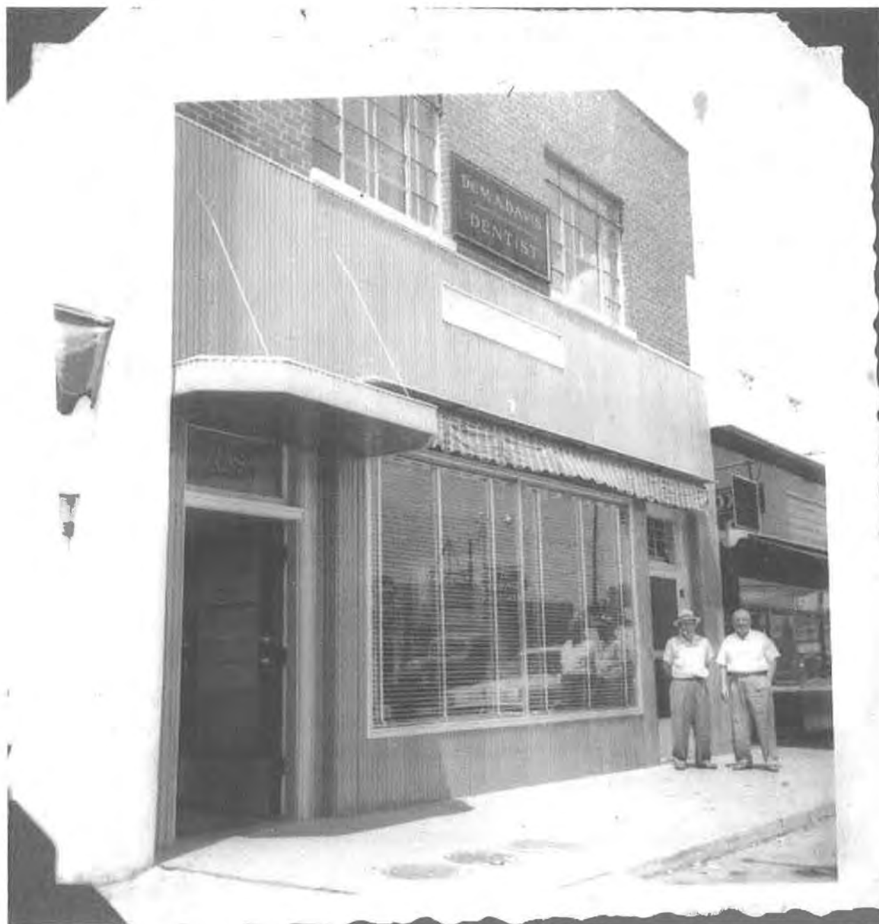
W. H. Koehler Building at 709 Main Street, c.1955. (Photo courtesy of the North Little Rock History Commission.)
