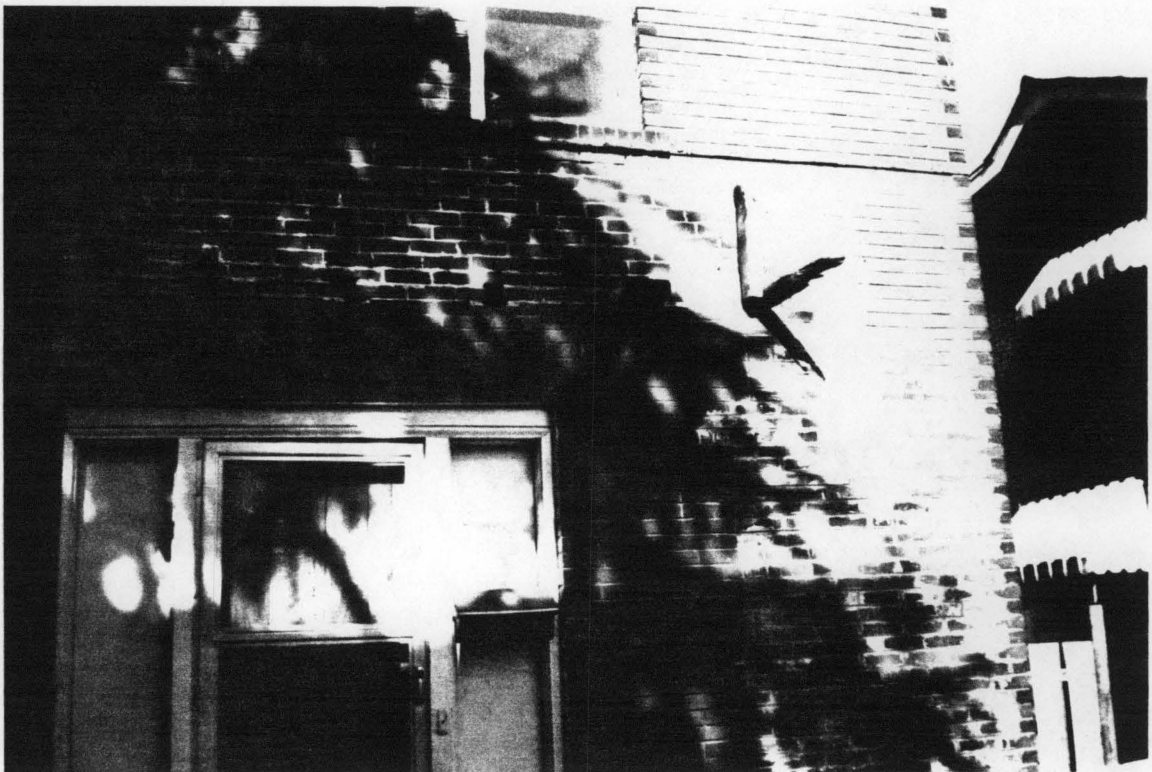
DETAIL OF REMOVED PORCH
