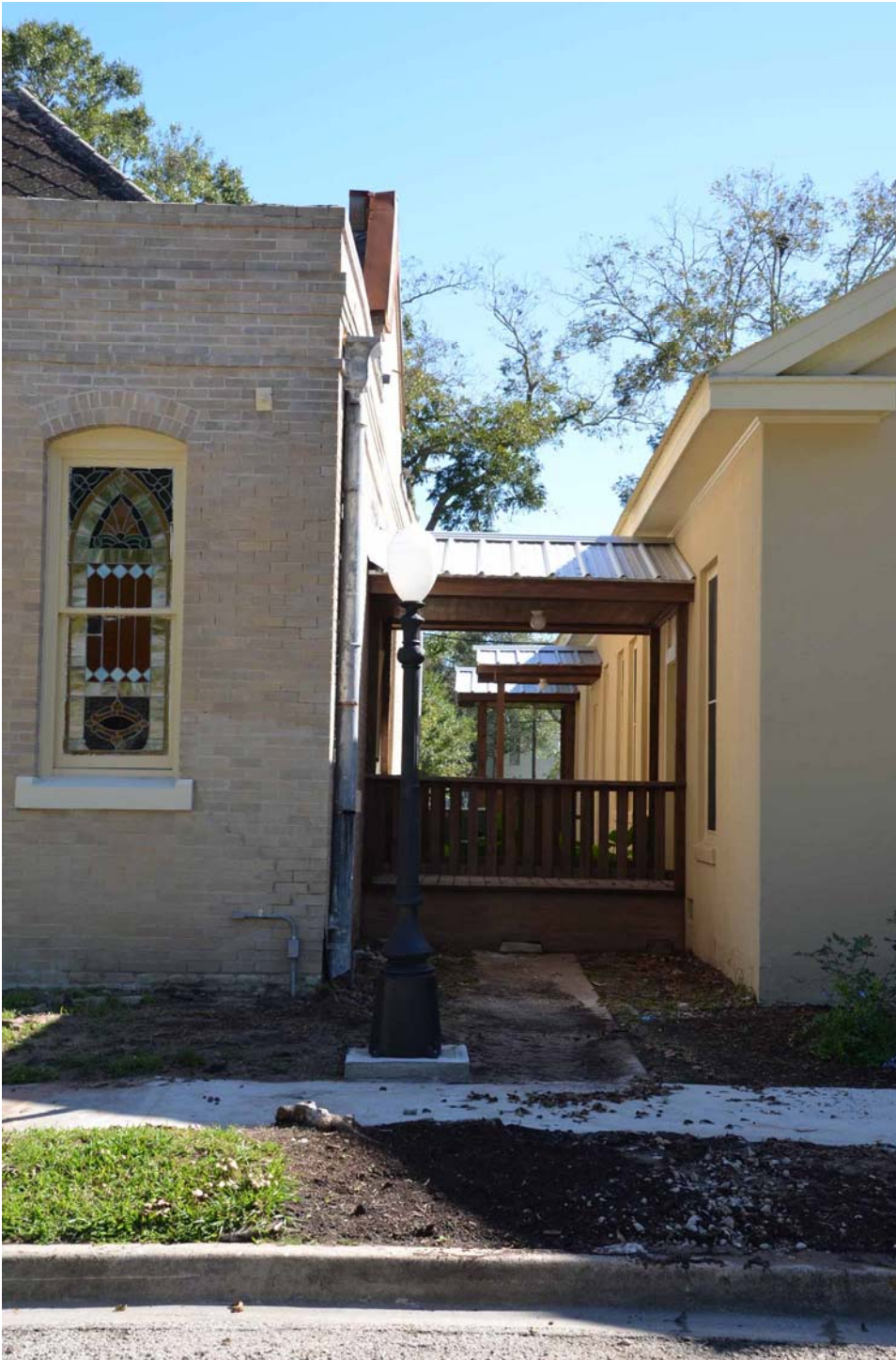
TX_Jackson County_Allen Memorial Presbyterian Church_0005.TIFF North and west elevations looking south showing connection between church and education building
