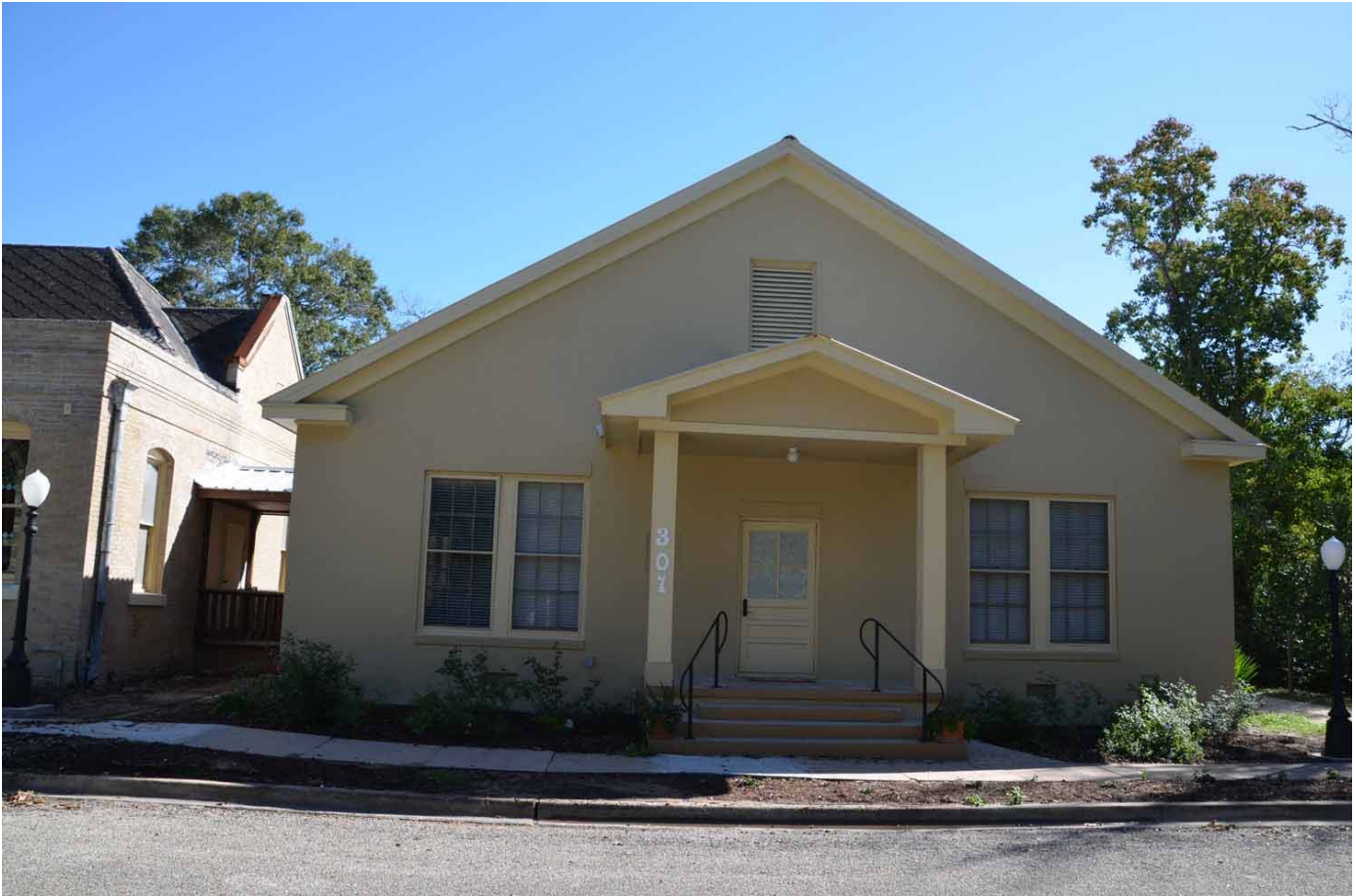
TX_Jackson County_Allen Memorial Presbyterian Church_0006.TIFF West elevation looking south (on left); north elevation of education building (on right; noncontributing)
