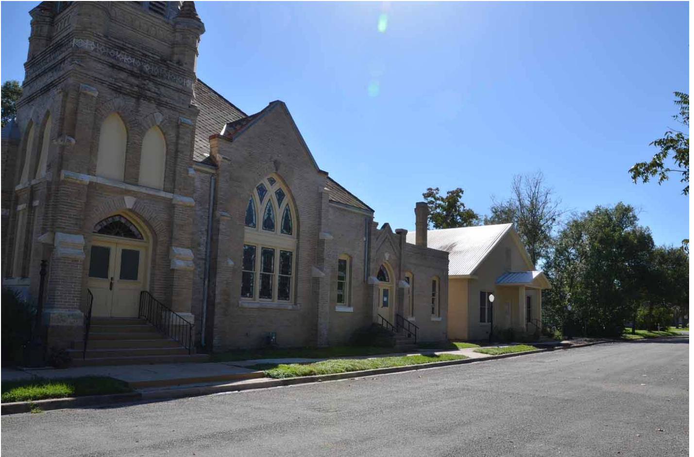
TX_Jackson County_Allen Memorial Presbyterian Church_ 0003.TIFF North elevation looking southwest
