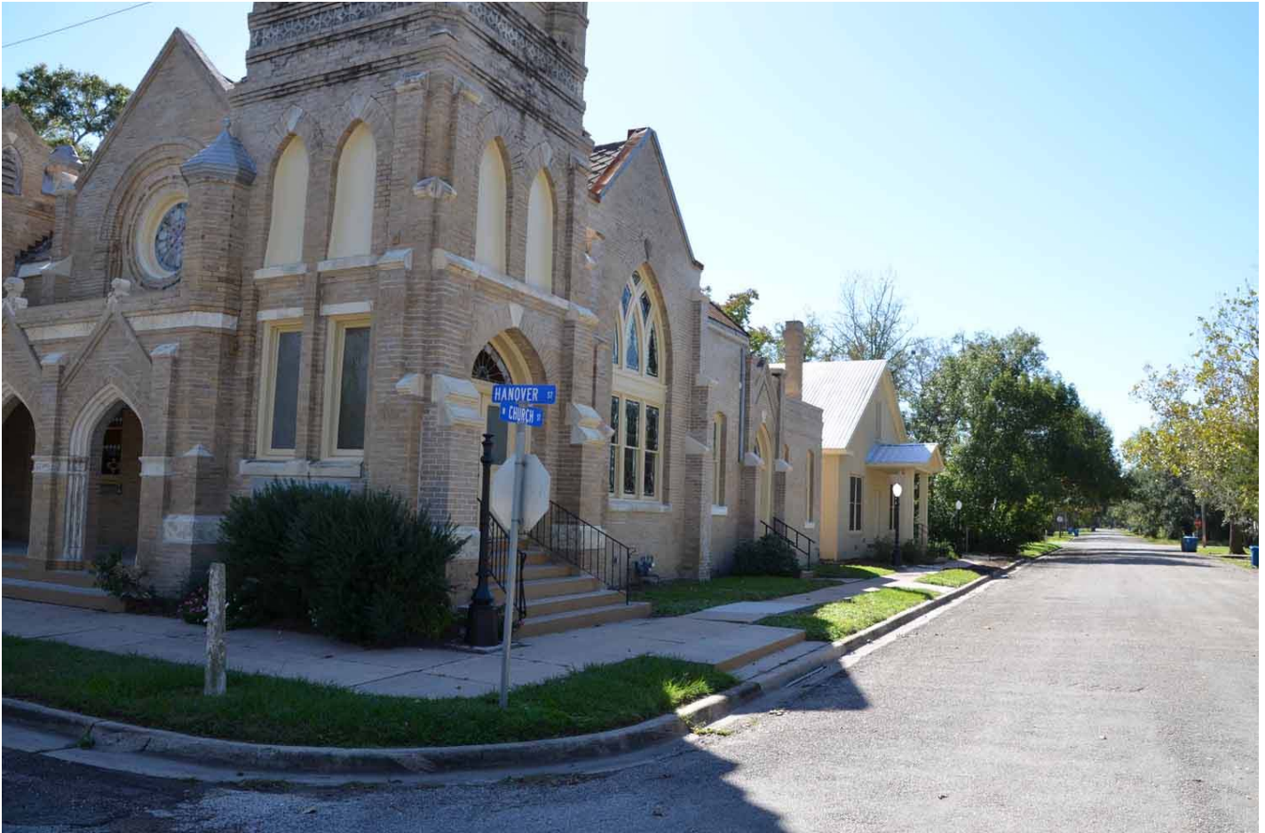
TX_Jackson County_Allen Memorial Presbyterian Church_0018.TIFF Looking west on Church Street
