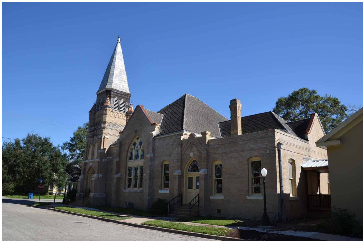
TX_Jackson County_Allen Memorial Presbyterian Church_ 0002.TIFF North elevation looking southeast
