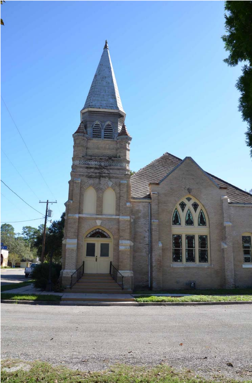
TX_Jackson County_Allen Memorial Presbyterian Church_0004.TIFF Northeast corner, north elevation looking south
