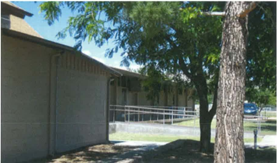
Figure 5. The 1940 (left of drain pipe) and 1966 additions.
