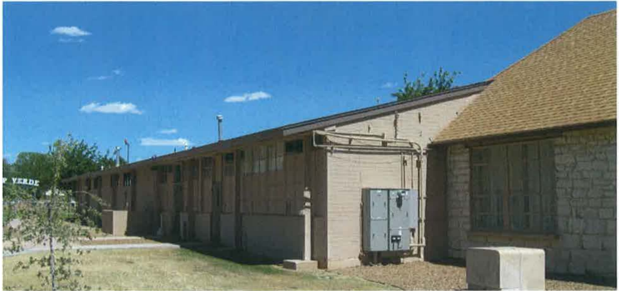
Figure 7. North façade of the 1950 addition.
