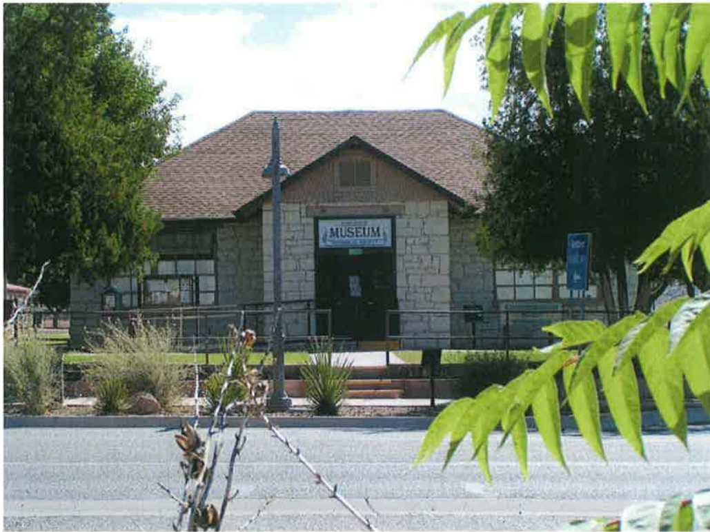
Photograph 3 of 17. Front façade, facing east.
