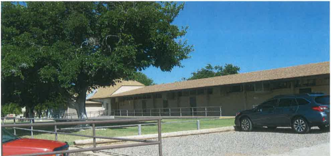
Figure 6. South facade of the 1950 addition. The rear entrance to the 1915 portion is on the far left of the addition, in the corner.
