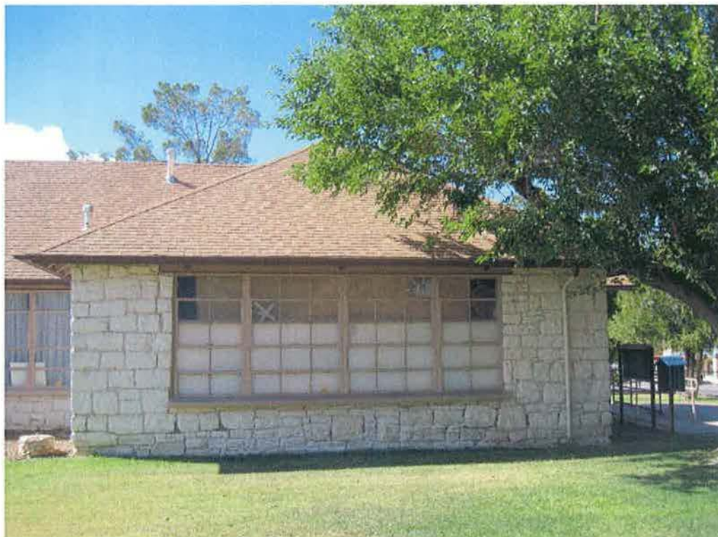
Photograph 17 of 17. Southern façade of 1915 portion.
