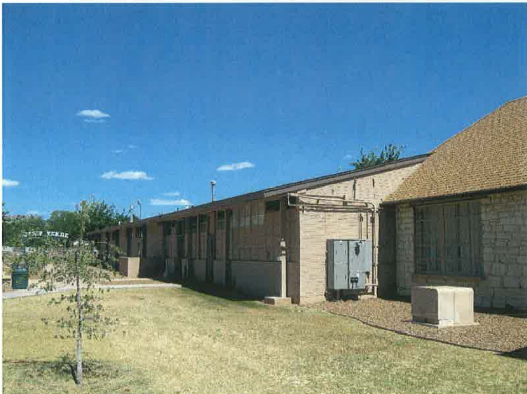
Photograph 16 of 17. Northern façade of rear addition, facing southeast.
