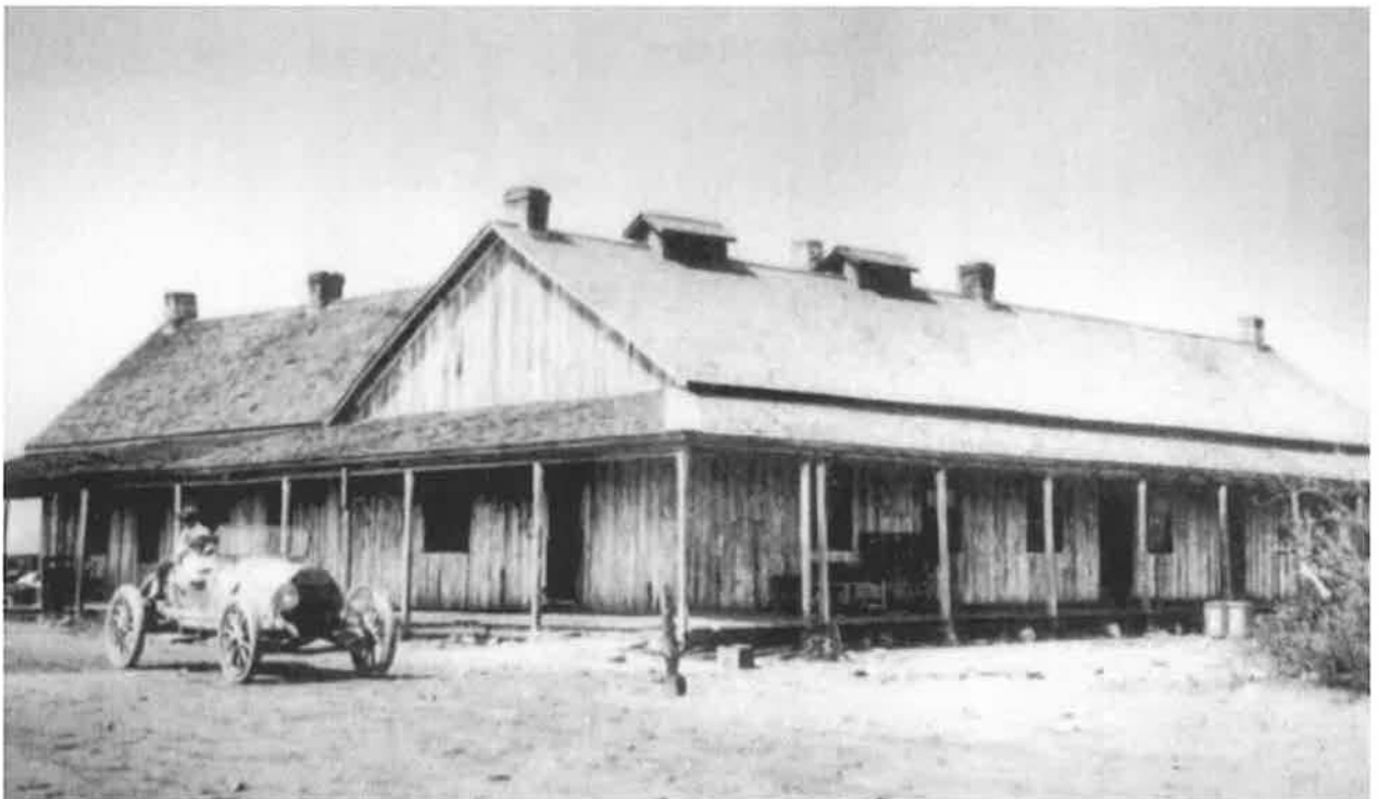
Figure 13. The Fort Verde Hospital was later used as a school. From Steve Ayers, Camp Verde .
