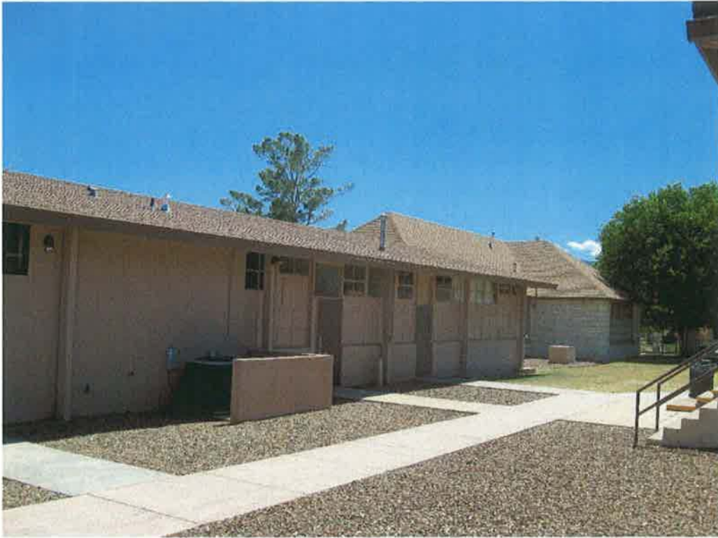
Photograph 15 of 17. Northern façade, facing southwest
