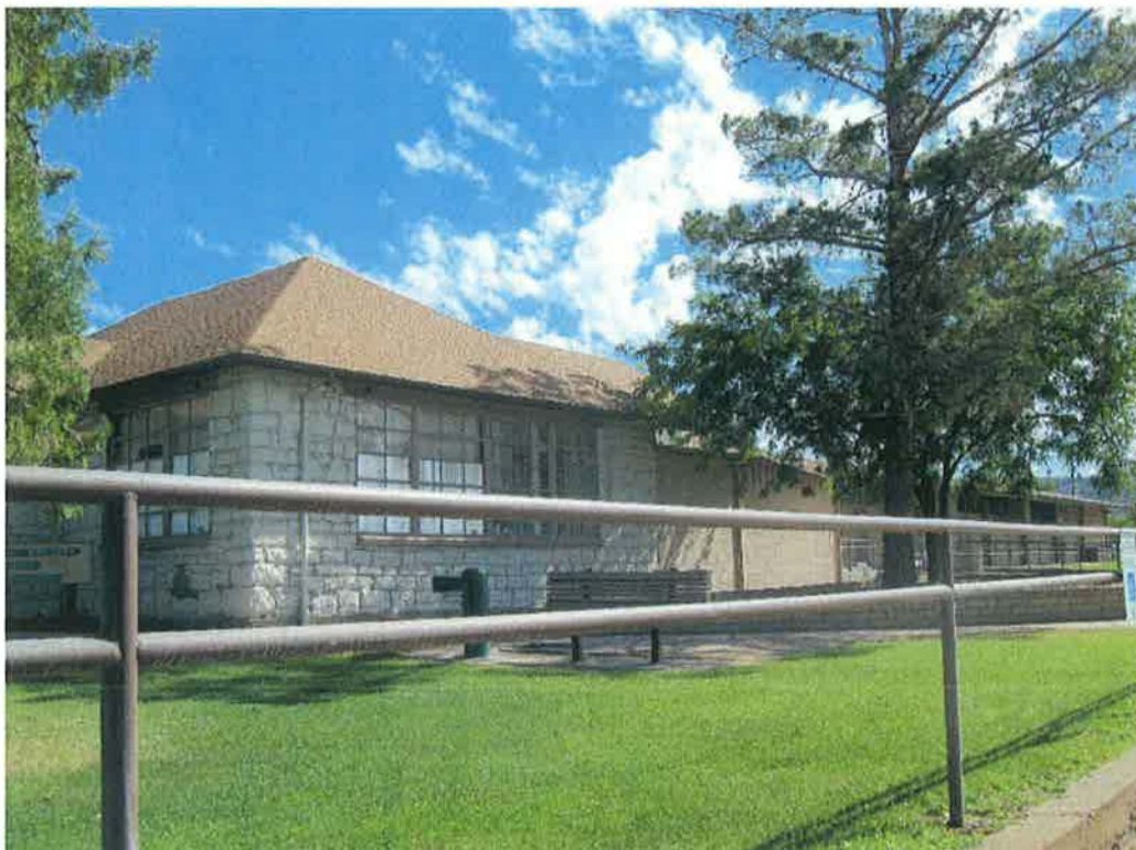
Photograph 8 of 17. South façade, facing northeast.
