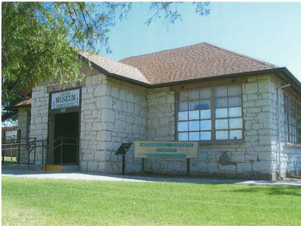
Photograph 7 of 17. Southwest corner, facing northeast.
