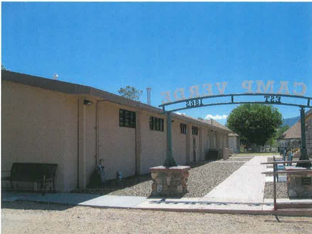
Photograph 14 of 17. Northern façade of rear addition, facing southwest.
