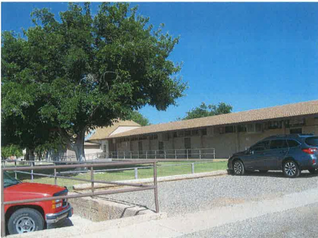
Photograph 12 of 17. Southern façade of rear addition, facing west.
