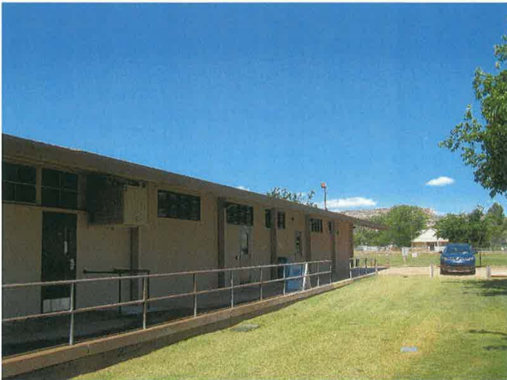
Photograph 11 of 17. Southern façade of rear addition facing east.
