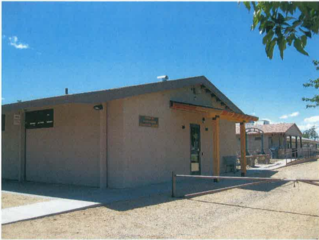
Photograph 13 of 17. Rear façade, municipal court entrance, facing northwest.
