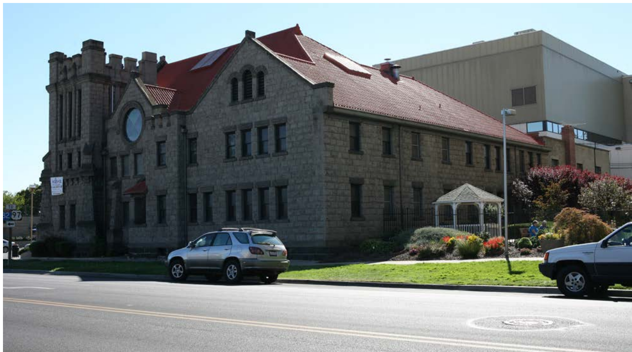
6 of 14. First Baptist Church, northeast corner showing side east (left) and rear north (right) facades.
