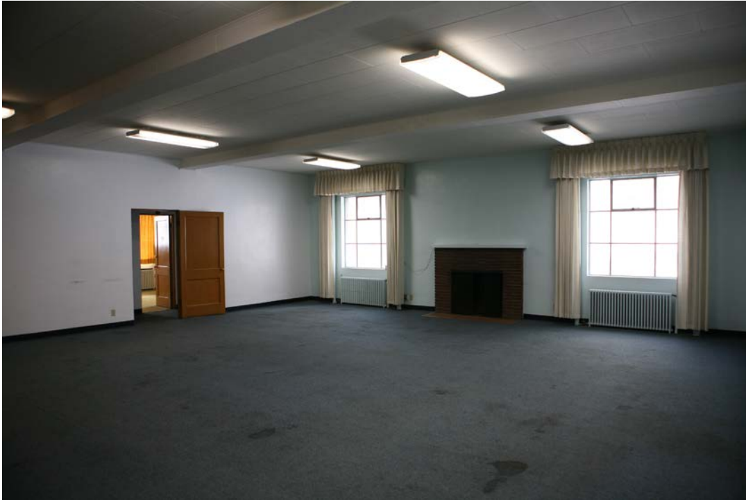
11 of 14. Interior view of church parlor in addition, camera facing northwest.
