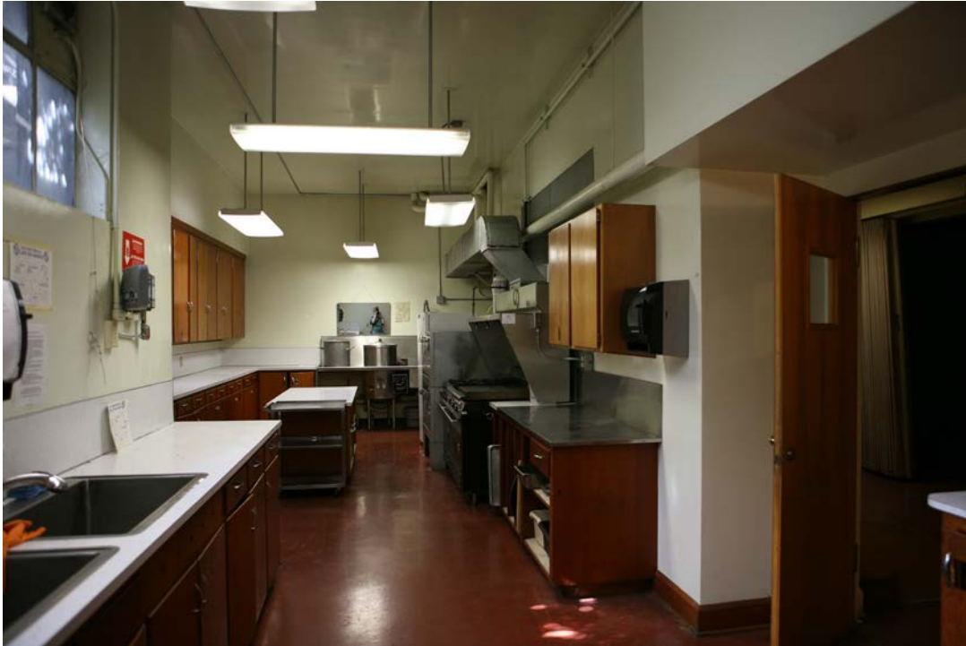
13 of 14. Interior view of main kitchen, in addition basement, camera facing west.
