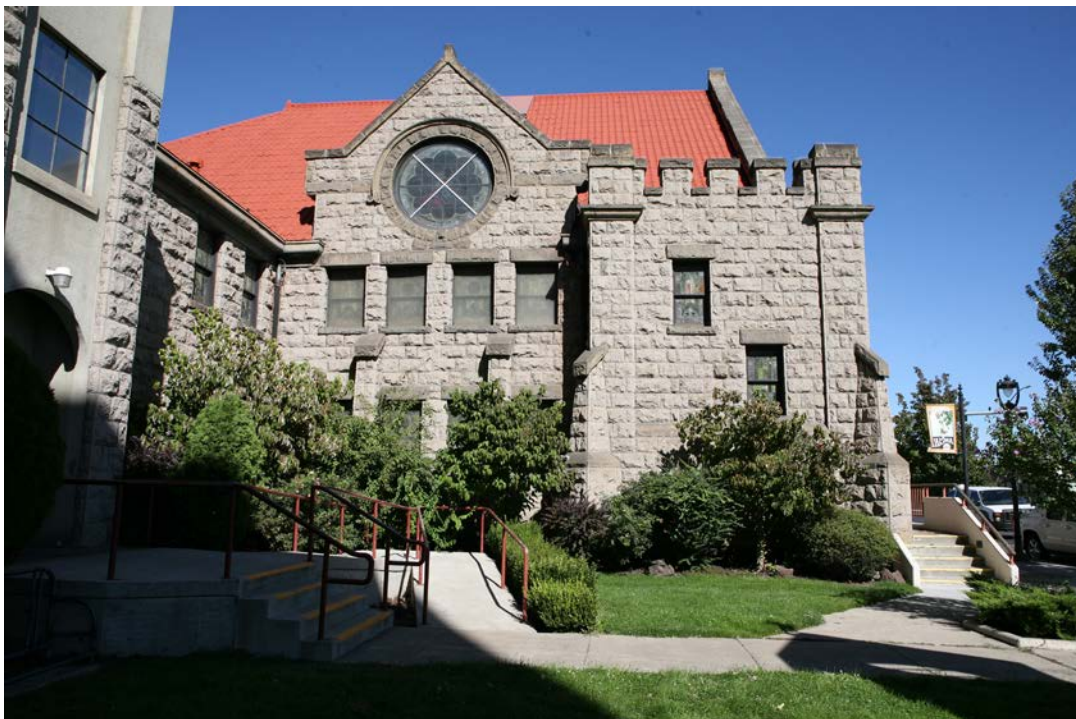
4 of 14. First Baptist Church, west facade of original building.
