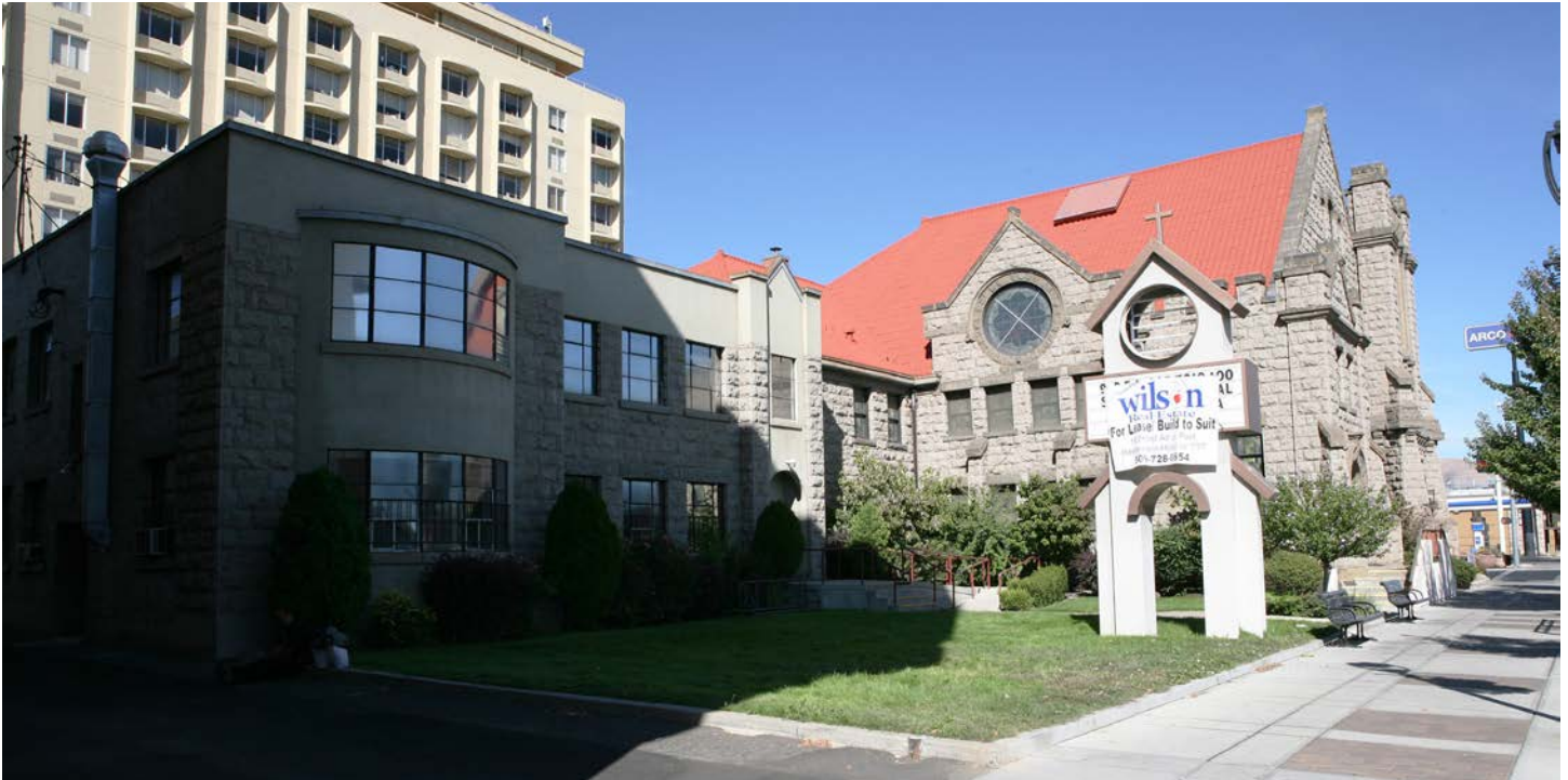
3 of 14. First Baptist Church, southwest corner showing the front south and side west facades.
