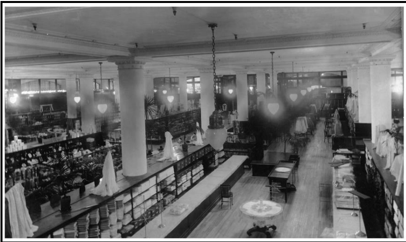
Figure 14. Interior of John A. Roberts' Department store on opening day, 1911. This photo was reproduced in the Utica Herald-Dispatch of 29 March 1911 (Collection Oneida County History Center, 2014.003.21).
