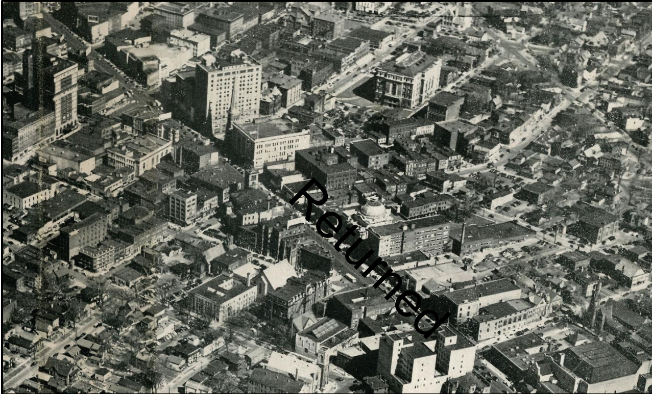
Figure 29. The Downtown Genesee Street district, seen from the south, looking east, c. 1952 (unidentified photographer).
