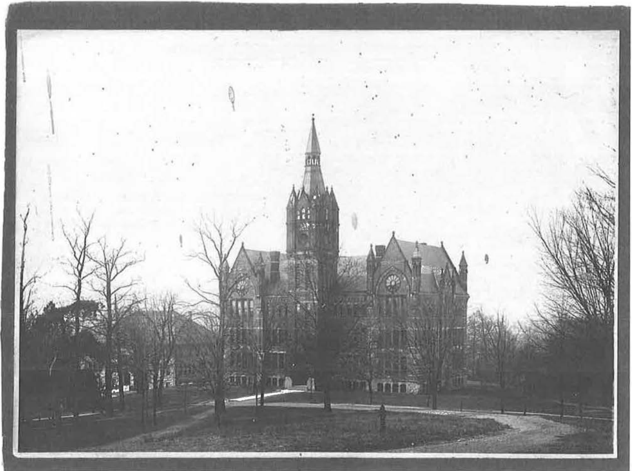
FIGURE 28 – Historic photo of Carnegie Hall and Recitation Hall; date unknown but post-1908; Wittenberg University Archives.
