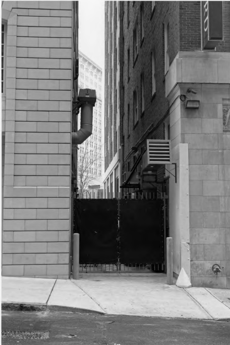
Wynne-Claughton Building Fulton County, Georgia Photograph 11 of 23
