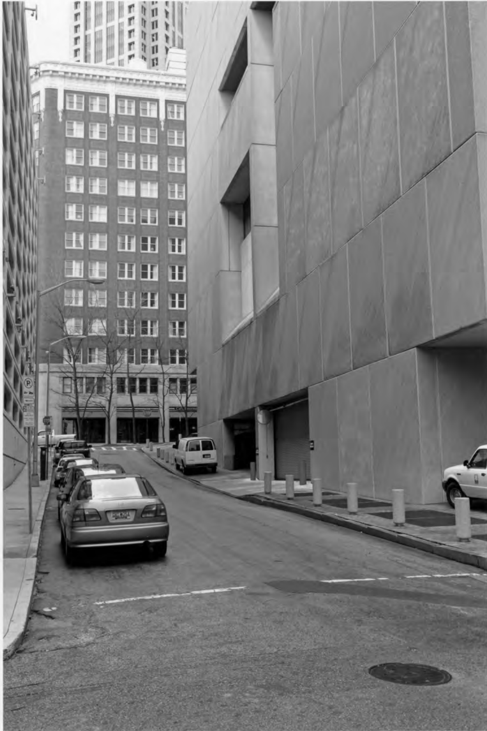
Wynne-Claughton Building Fulton County, Georgia Photograph 10 of 23
