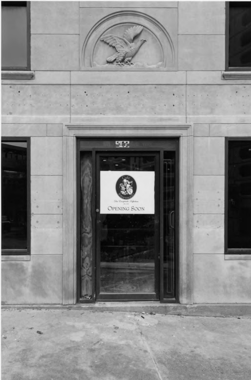
Wynne-Claughton Building Fulton County, Georgia Photograph 6 of 23
