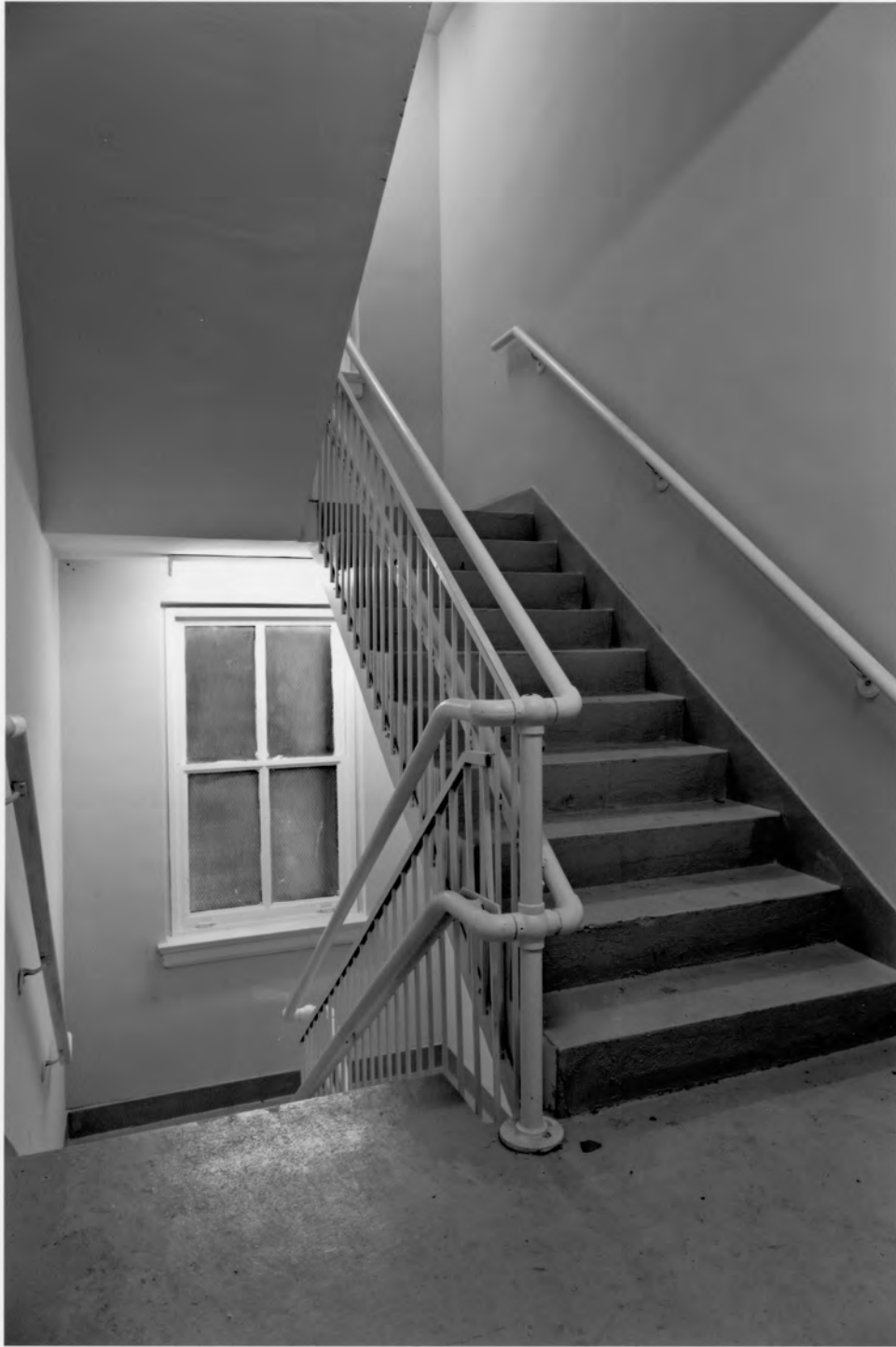
Wynne-Claughton Building Fulton County, Georgia Photograph 19 of 23
