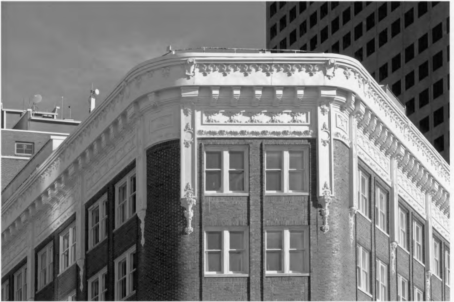
Wynne-Claughton Building Fulton County, Georgia Photograph 12 of 23
