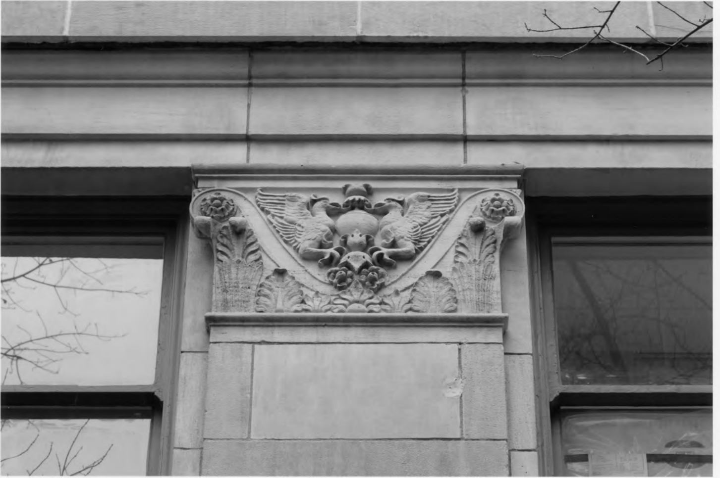
Wynne-Claughton Building Fulton County, Georgia Photograph 9 of 23
