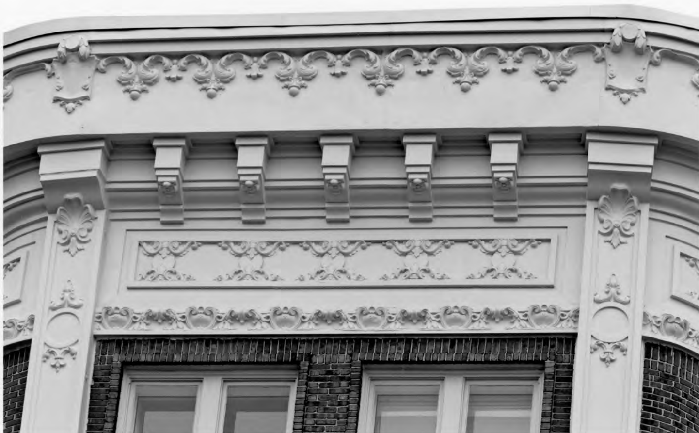
Wynne-Claughton Building Fulton County, Georgia Photograph 13 of 23
