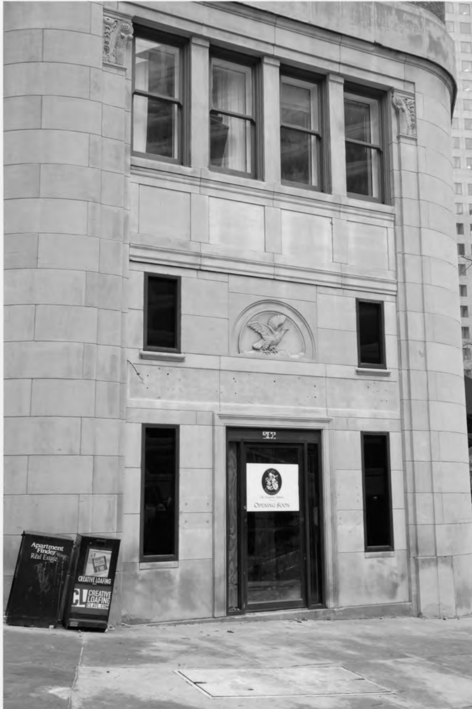
Wynne-Claughton Building Fulton County, Georgia Photograph 5 of 23
