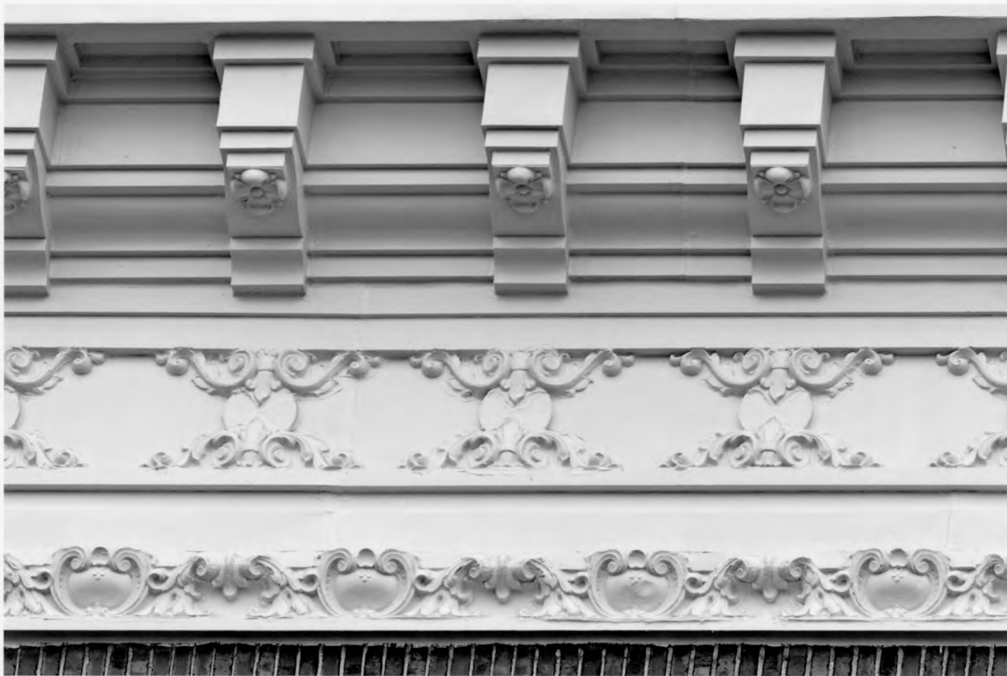
Wynne-Claughton Building Fulton County, Georgia Photograph 14 of 23
