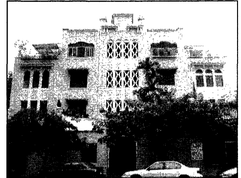
Fig. 3 Edificio Victory Garden. South facade.
