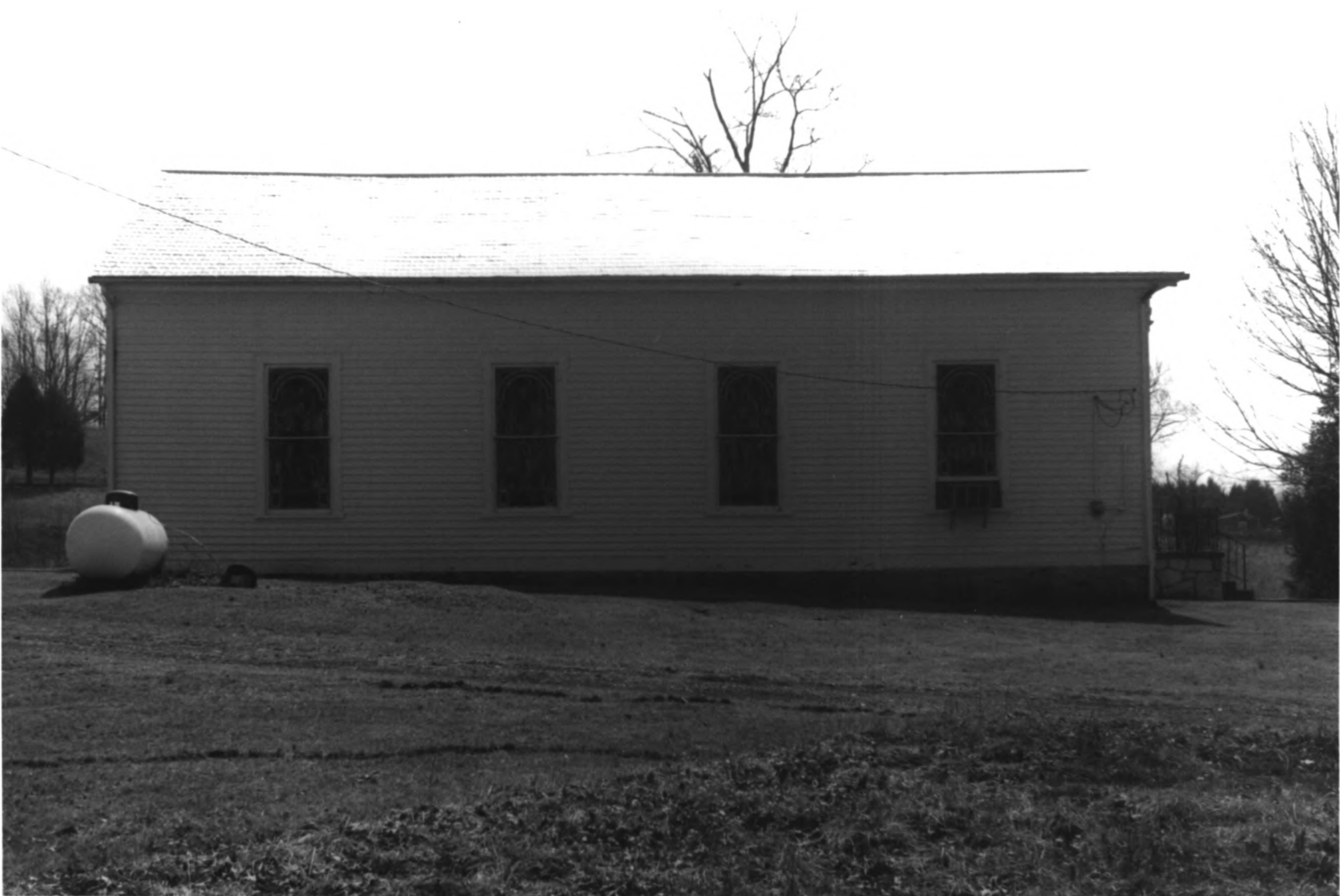
Bethany Presbyterian Church Complex Giles County TN
