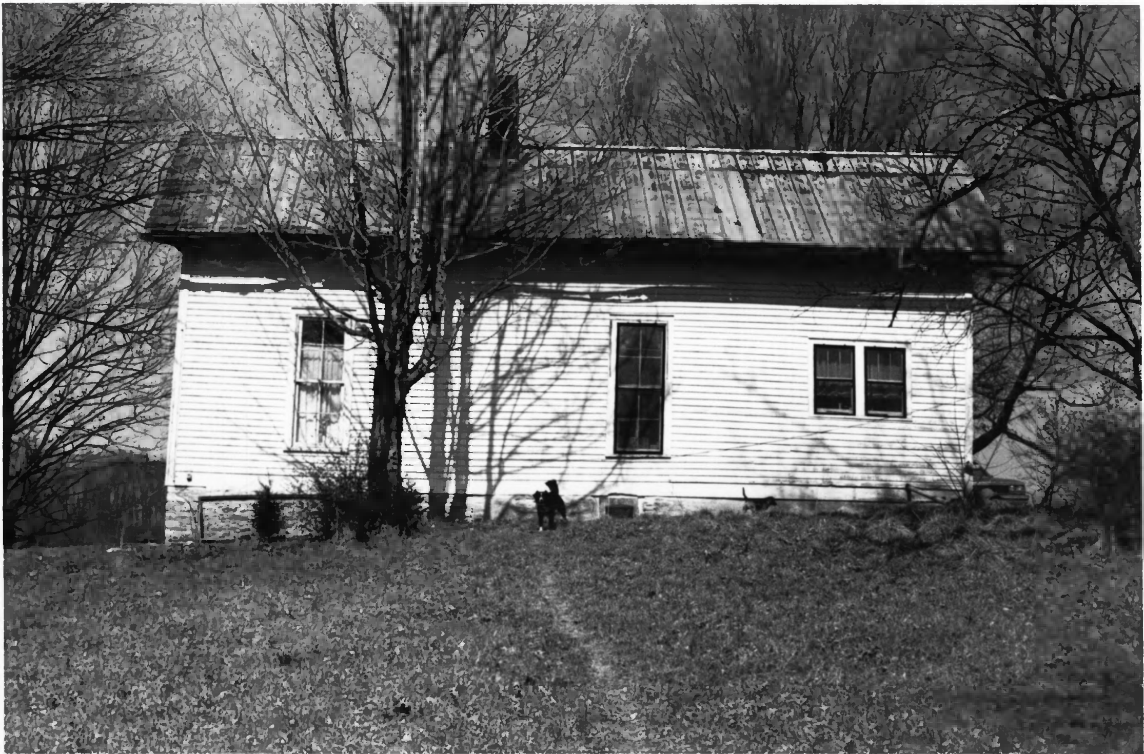
Bethany Presbyterian Church Complex Giles County TN
