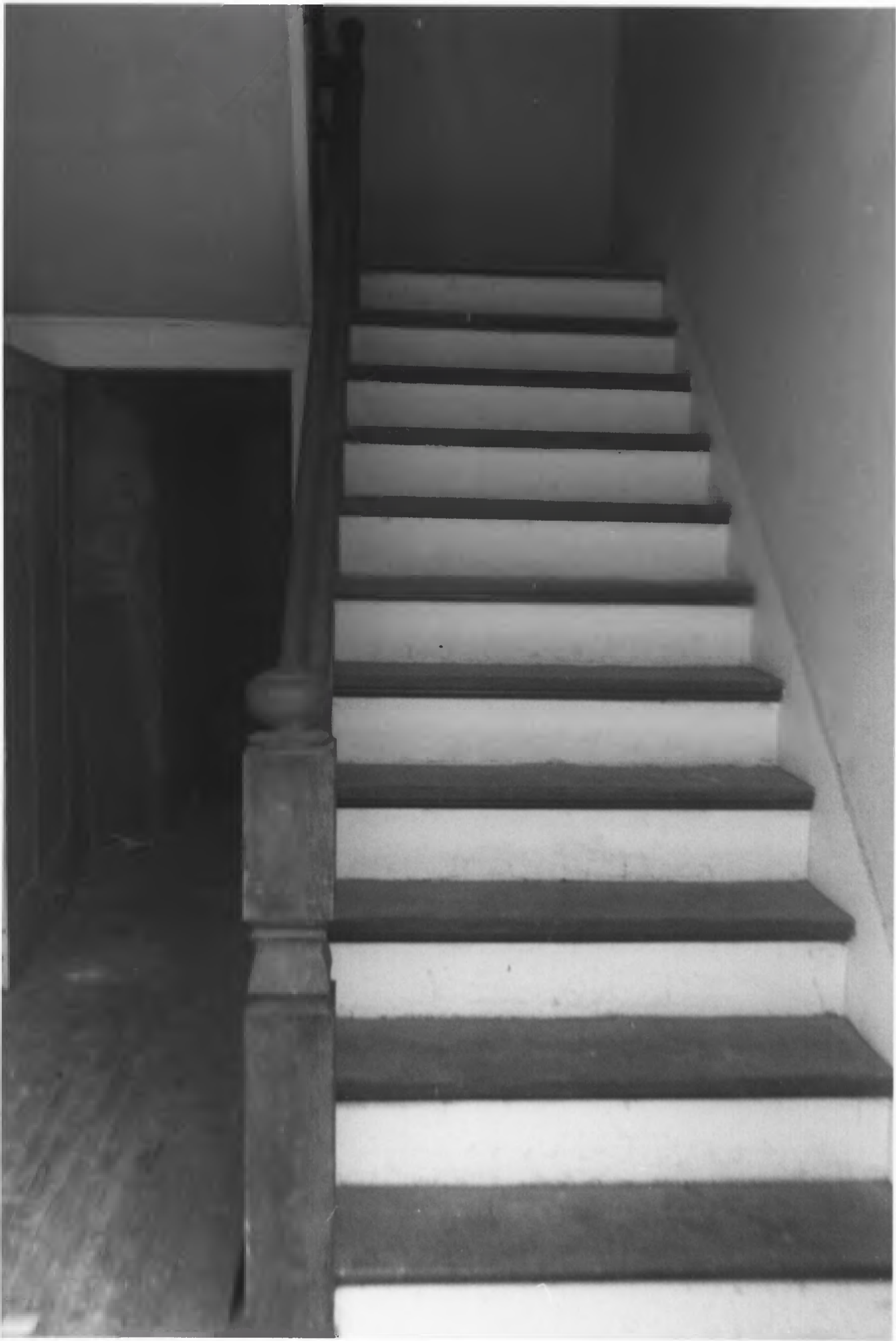
Bethany Presbyterian Church Complex Giles County TN
