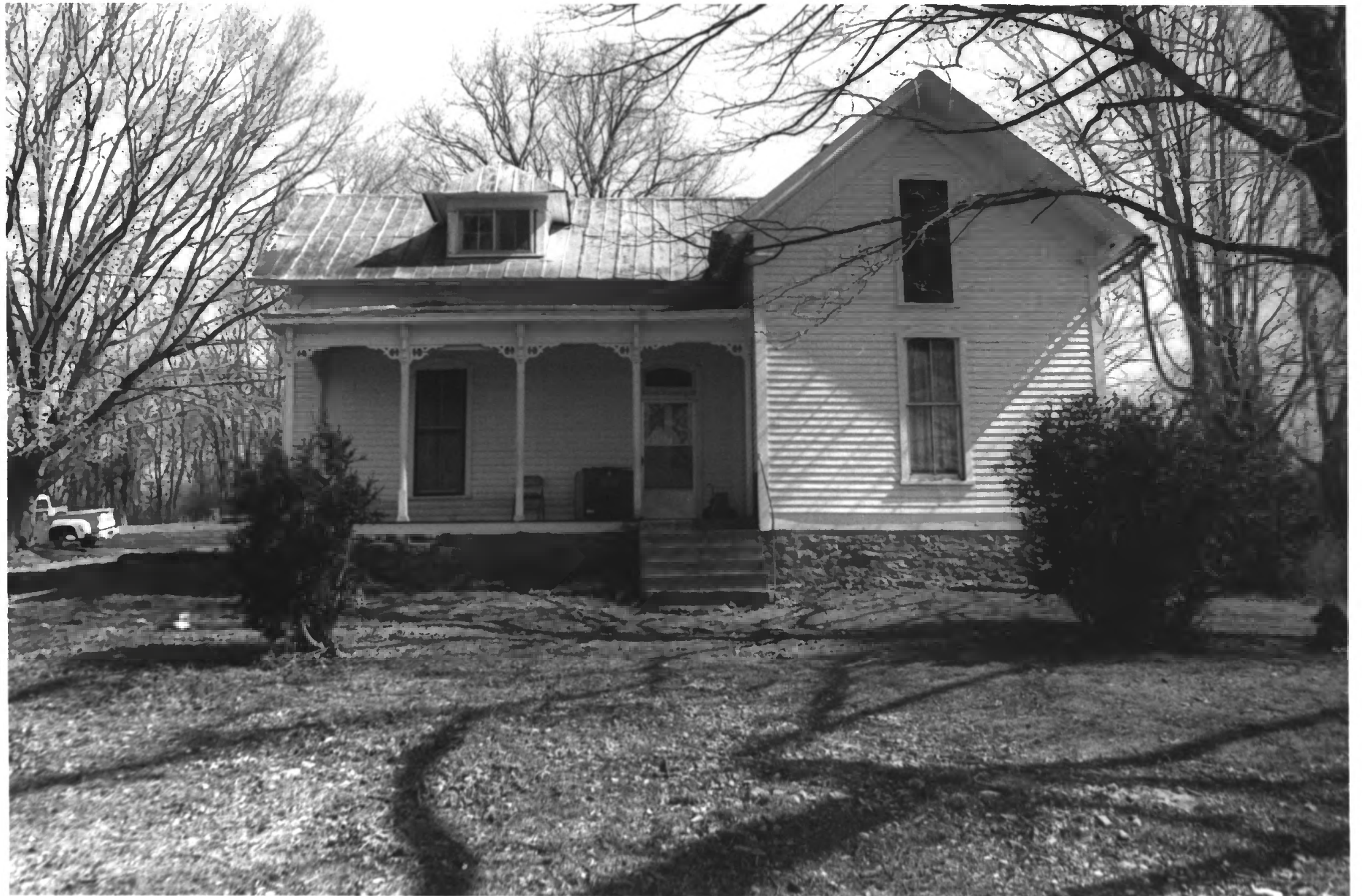
Bethany Presbyterian Church Complex Giles County TN
