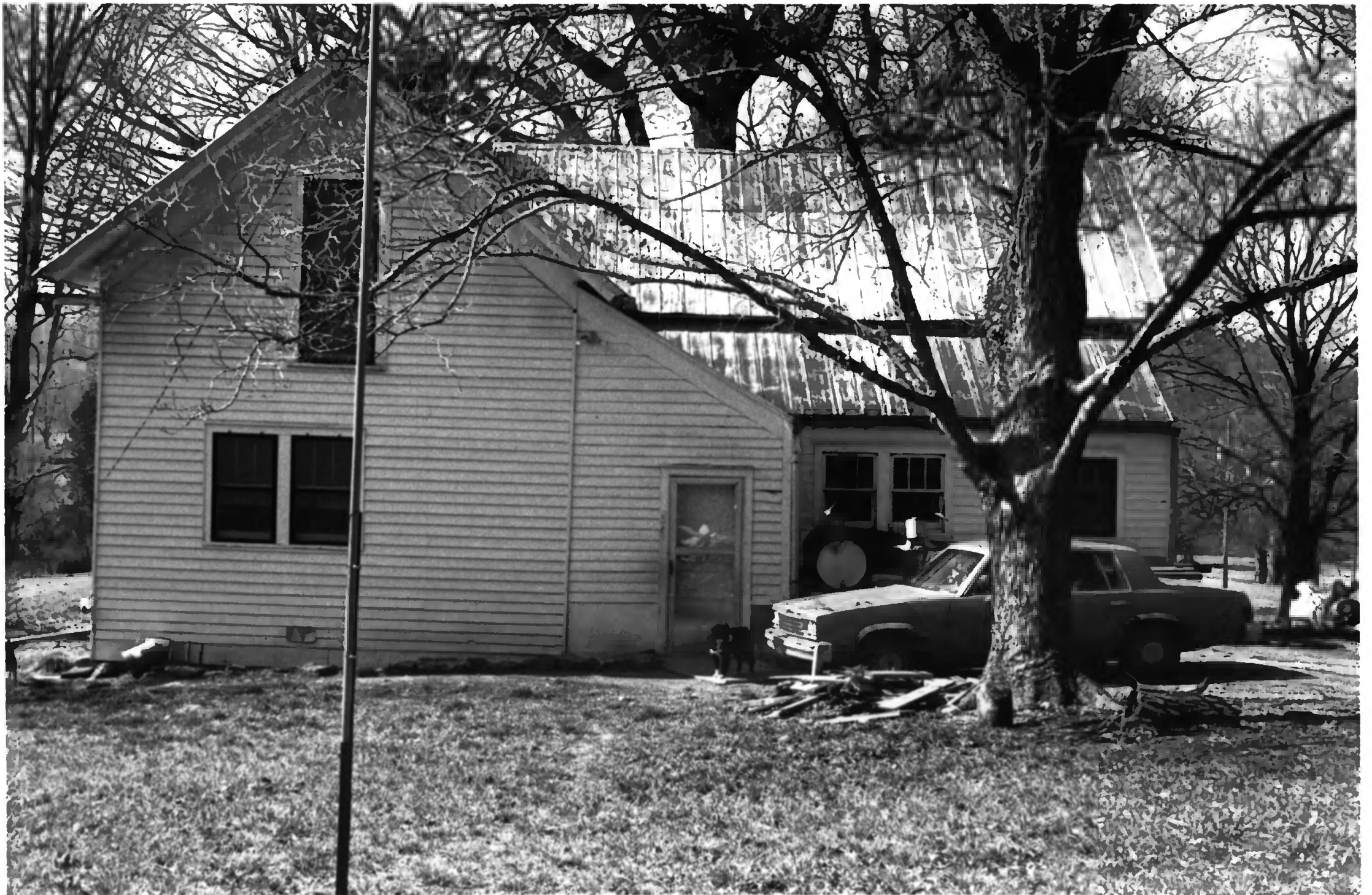
Bethany Presbyterian Church Complex Giles County TN
