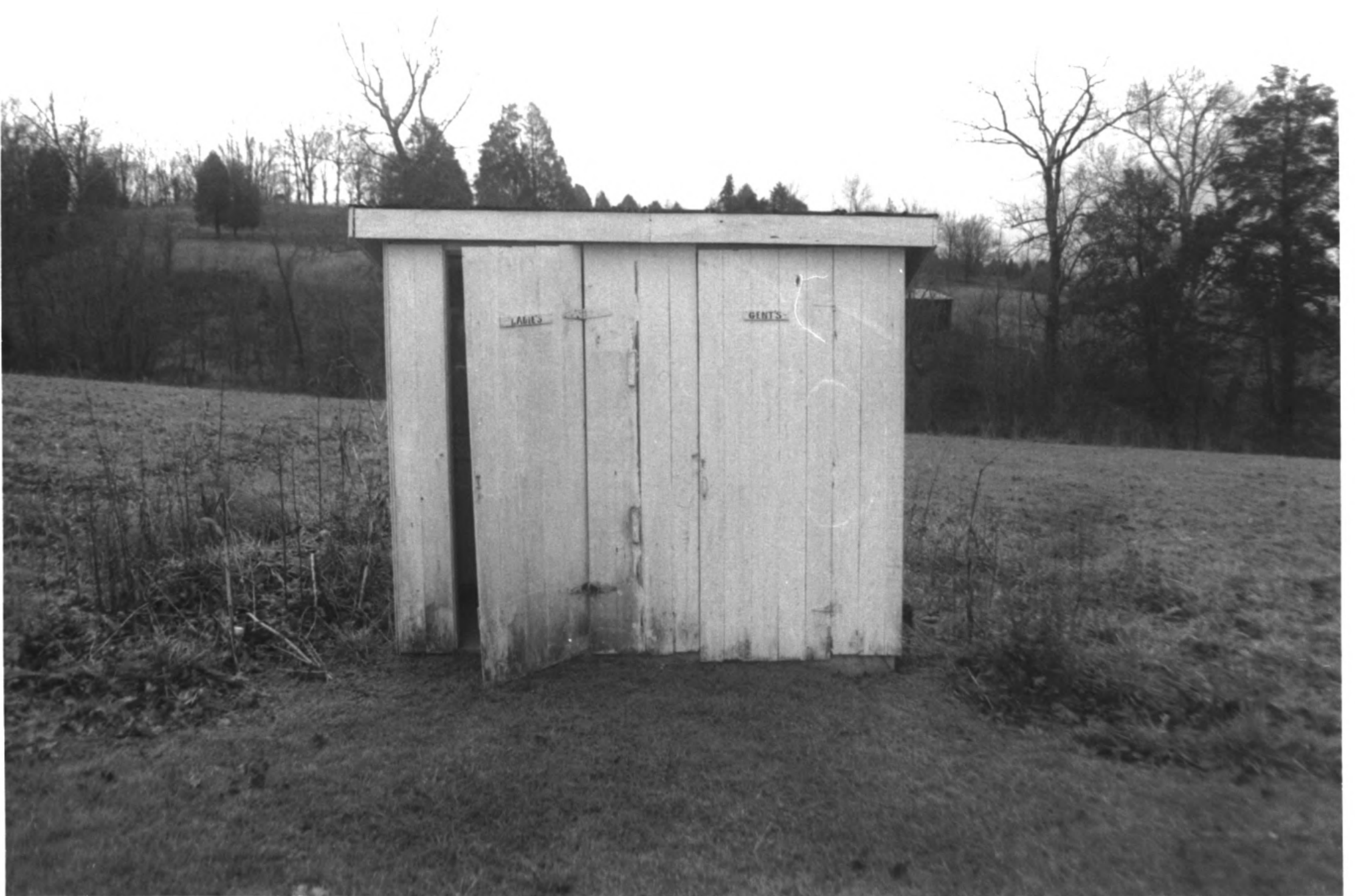
Bethany Presbyterian Church Complex Giles County TN
