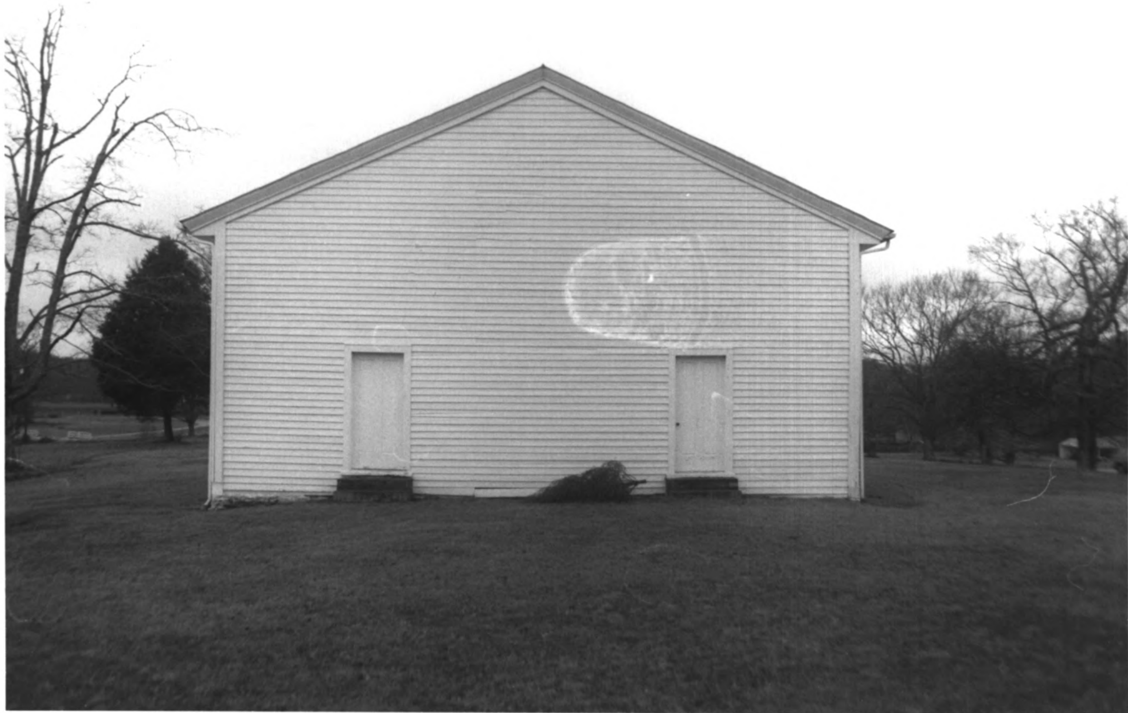
Bethany Presbyterian Church Complex Giles County TN
