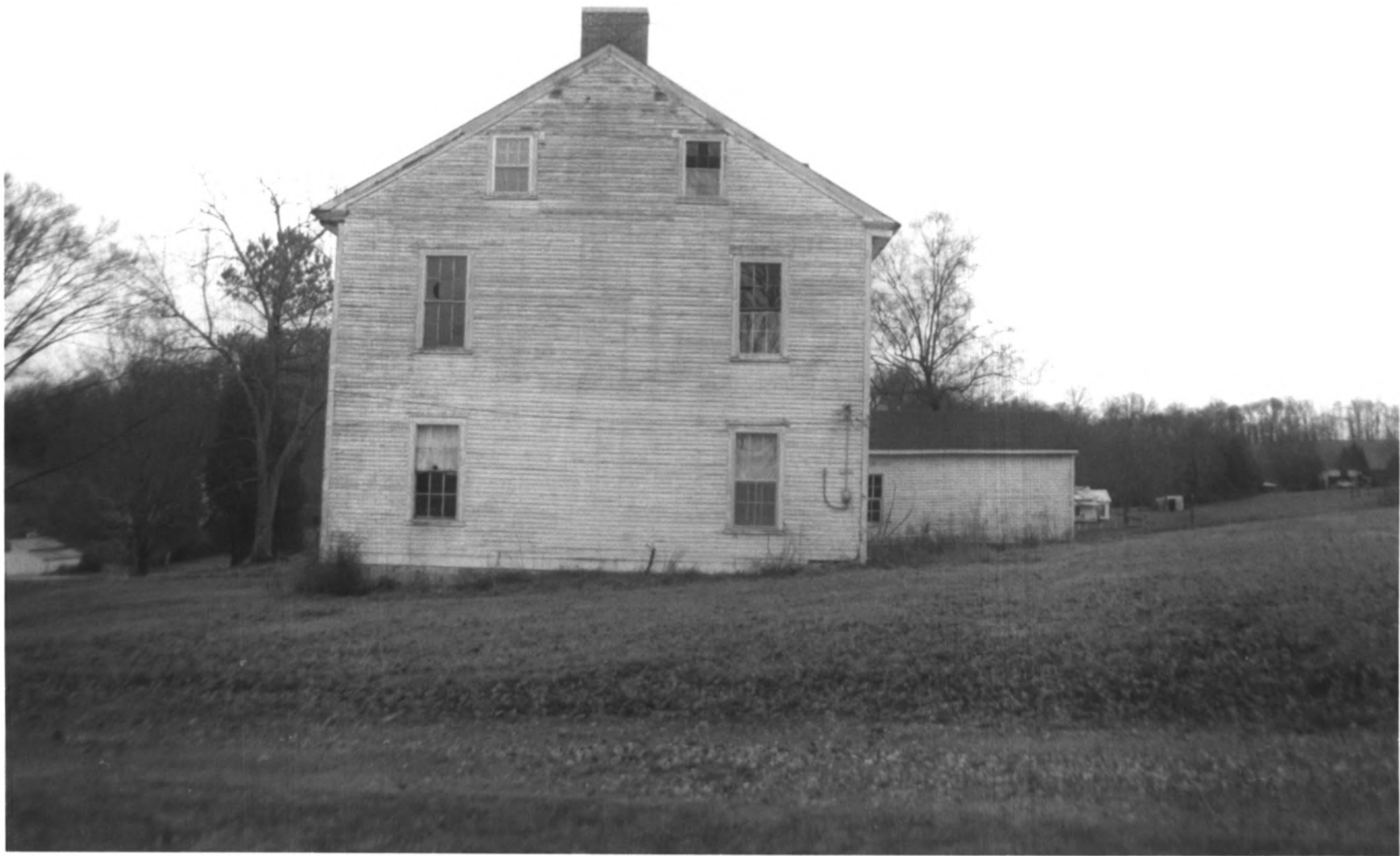
Bethany Presbyterian Church Complex Giles County TN
