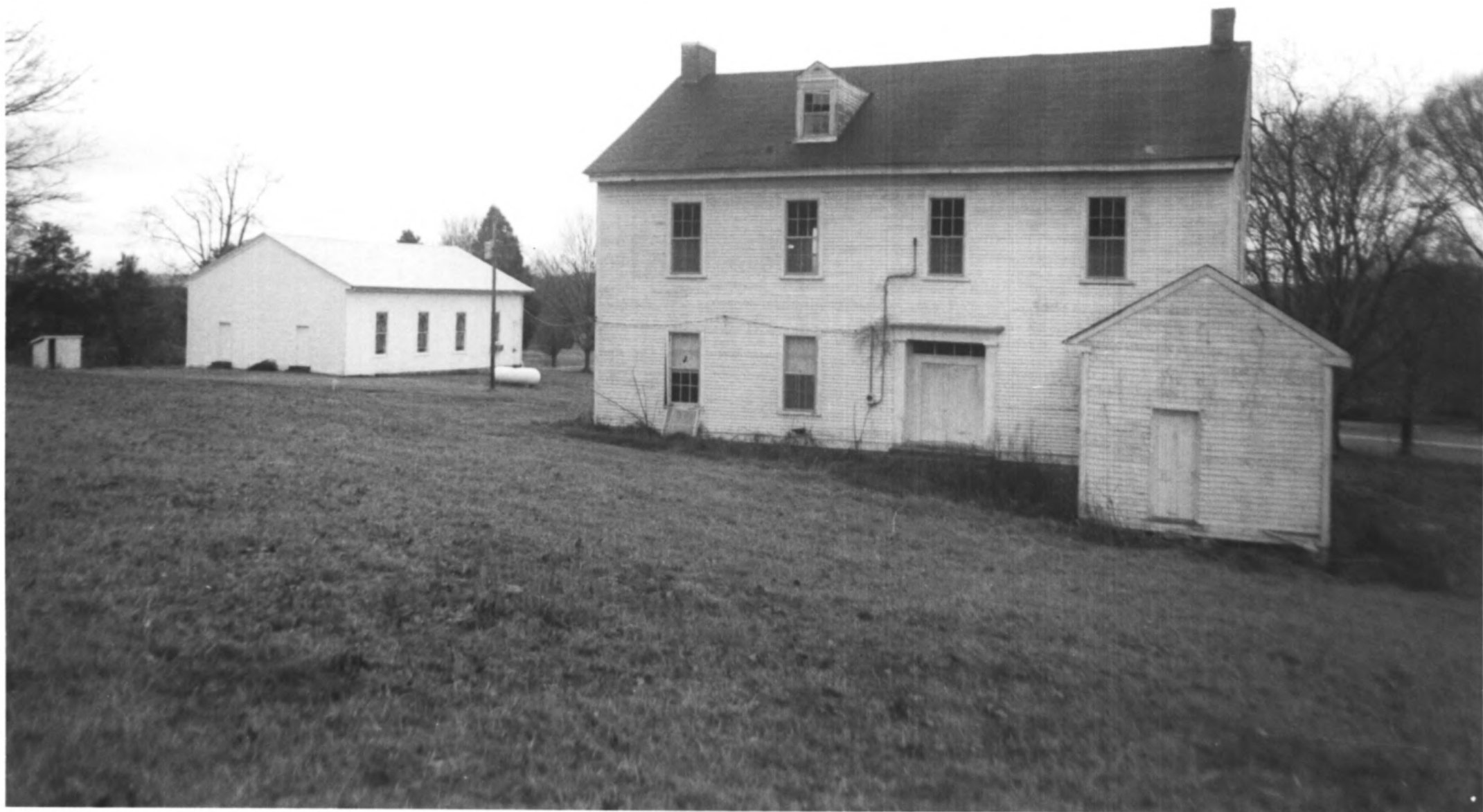
Bethany Presbyterian Church Complex Giles County TN
