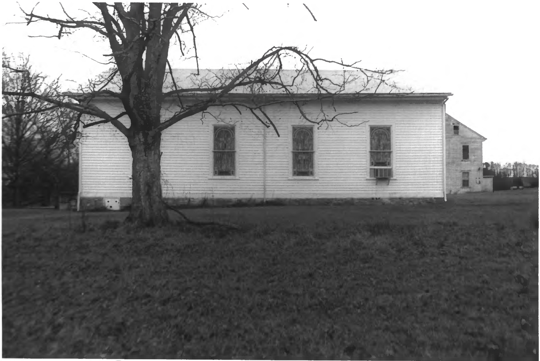
Bethany Presbyterian Church Complex Giles County TN
