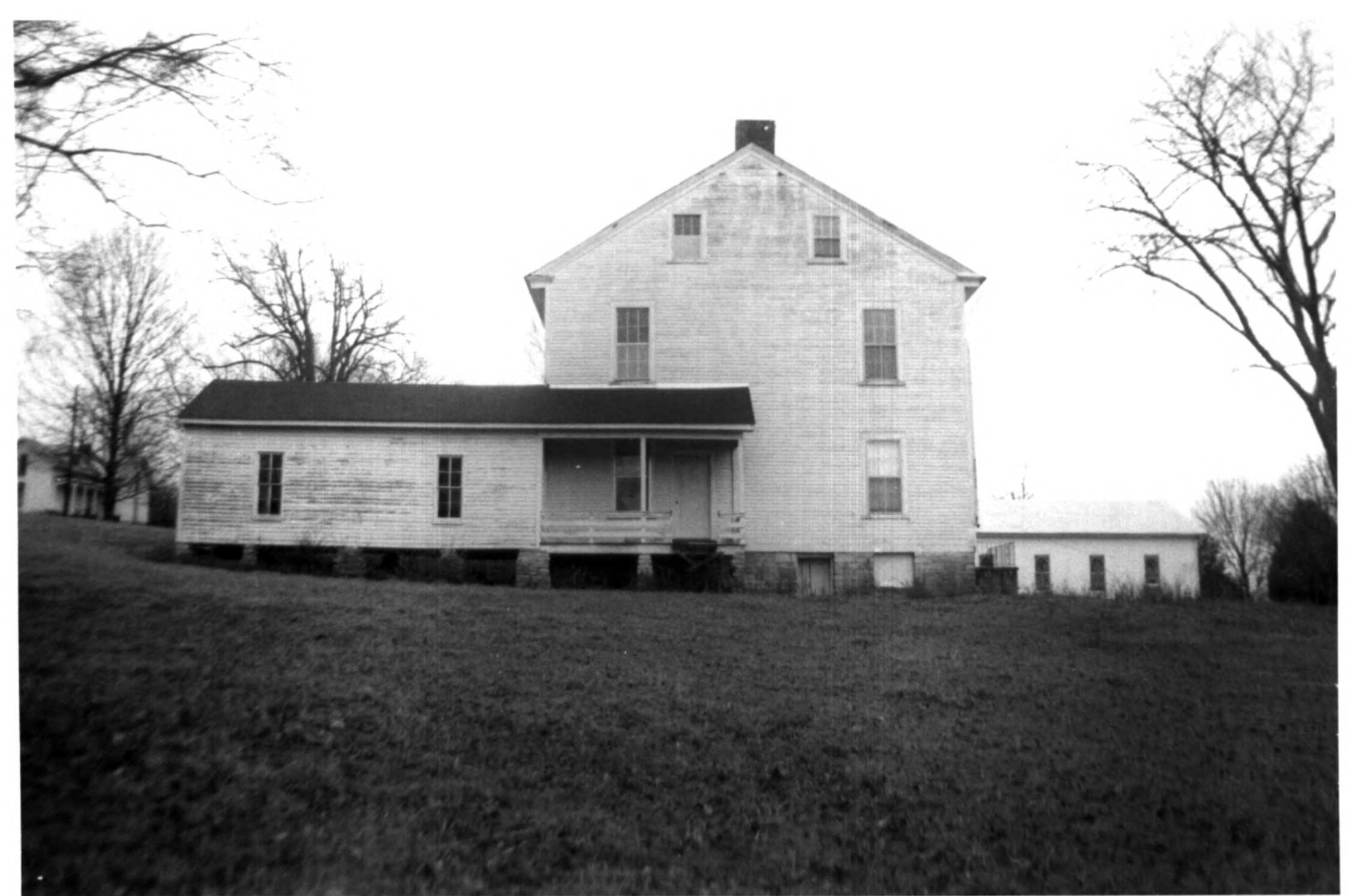
Bethany Presbyterian Church complex Giles County TN
