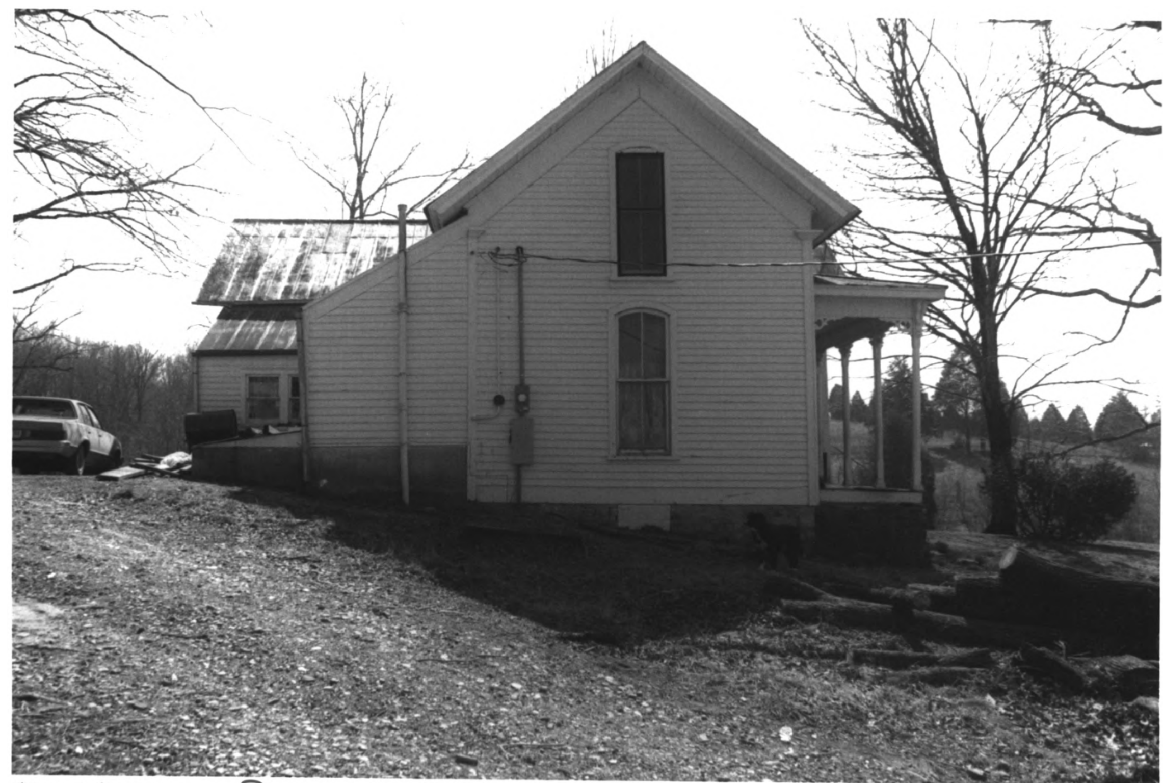
Bethany Presbyterian Church Complex Giles County TN
