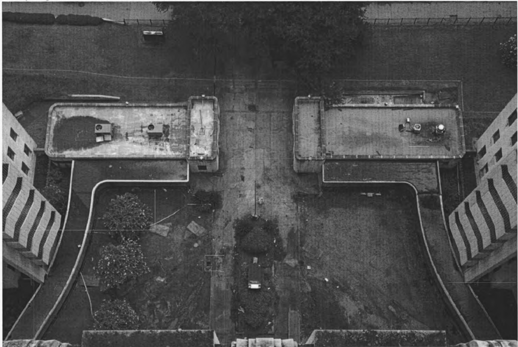
Figure 12. Charity Hospital, Courtyard with waiting rooms and breezeways (Robert Tucher, July 2009).
