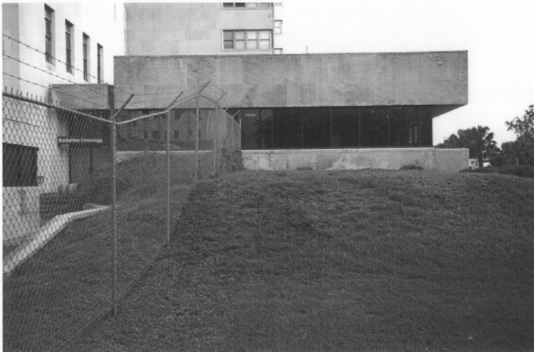
Figure 47. Charity Hospital, Radiation and Oncology addition, side elevation. Early 1980s (Robert Tucher, July 2009).
