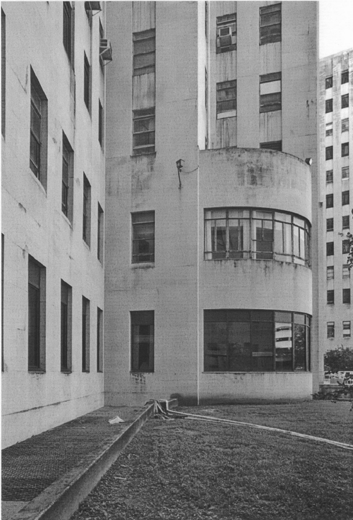
Figure 23. Charity Hospital, The elliptical wall viewed from the courtyard (Earth Search, Inc., July 2009).
