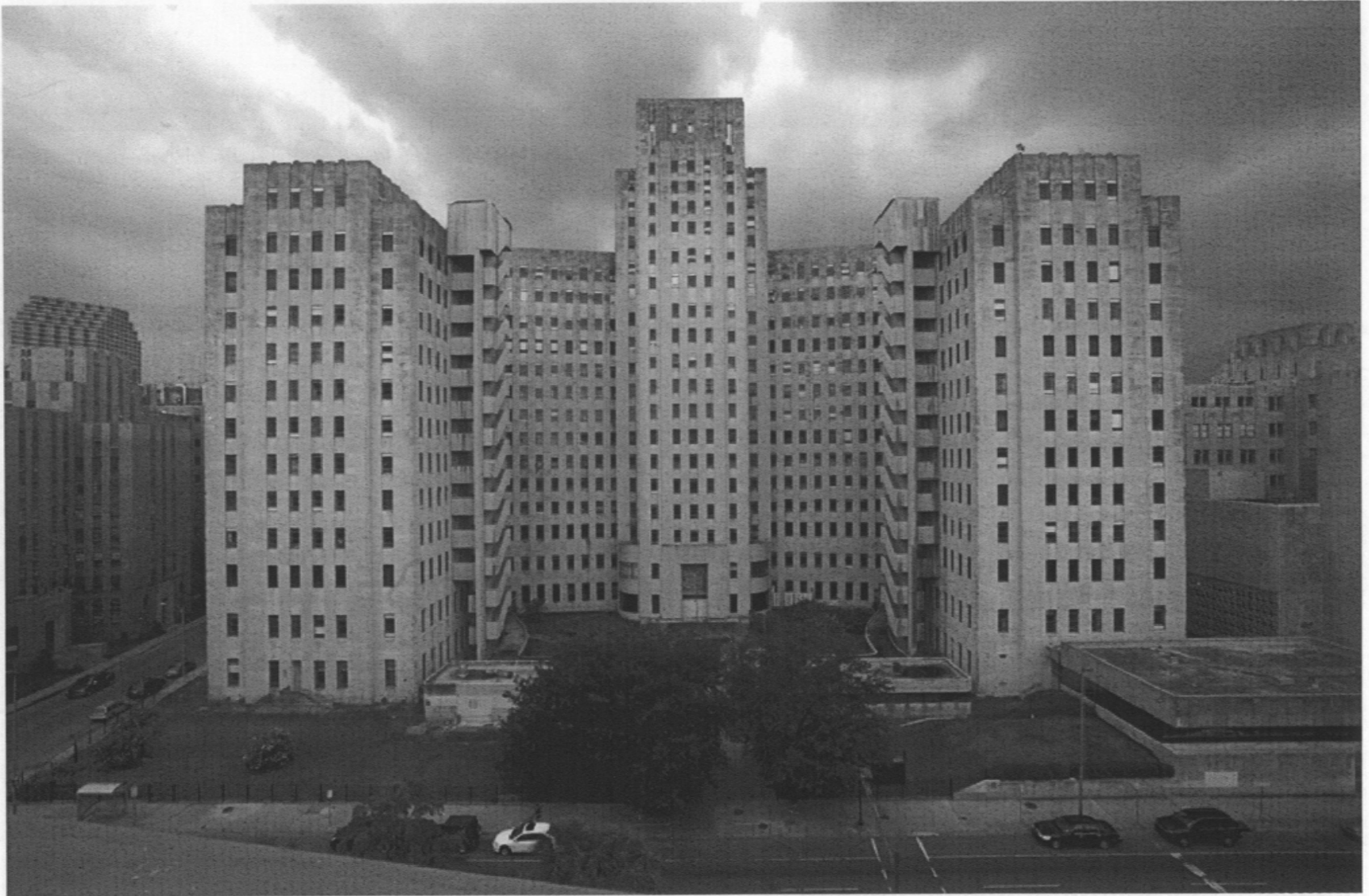
Figure 6. Charity Hospital, Tulane Avenue façade (Robert Tucher, photographer, July 2009).
