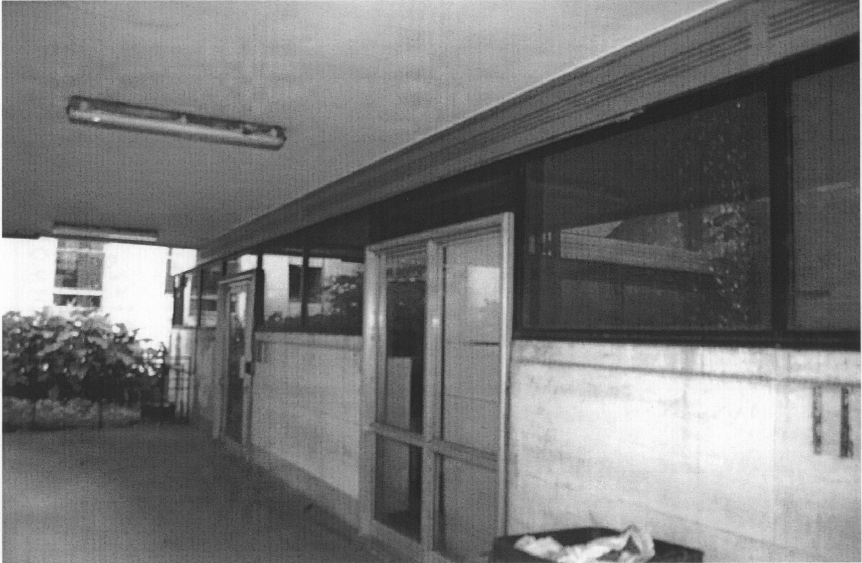
Figure 15. Charity Hospital, Waiting room, Inner courtyard elevation (Earth Search, Inc., July 2009).
