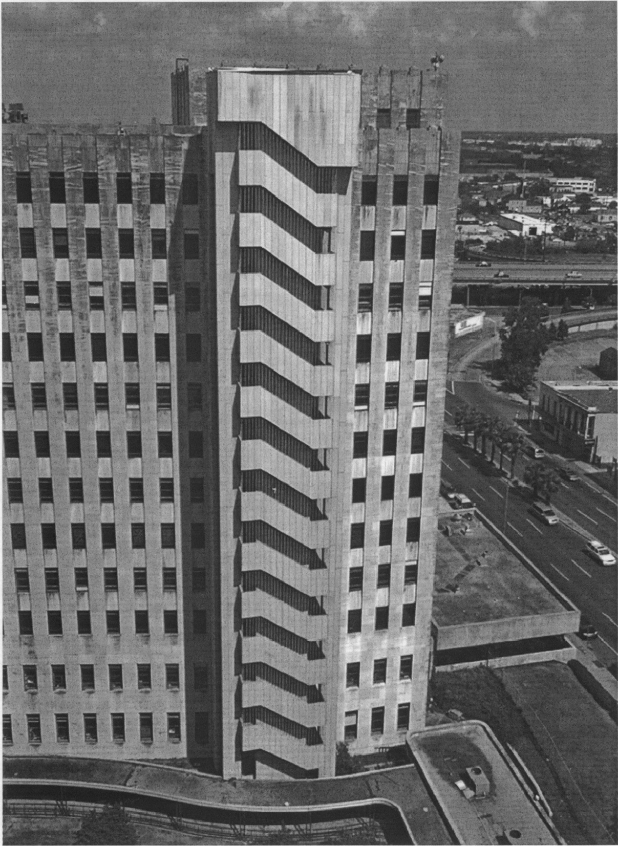
Figure 24. Charity Hospital, An emergency staircase located in the front courtyard (FEMA).
