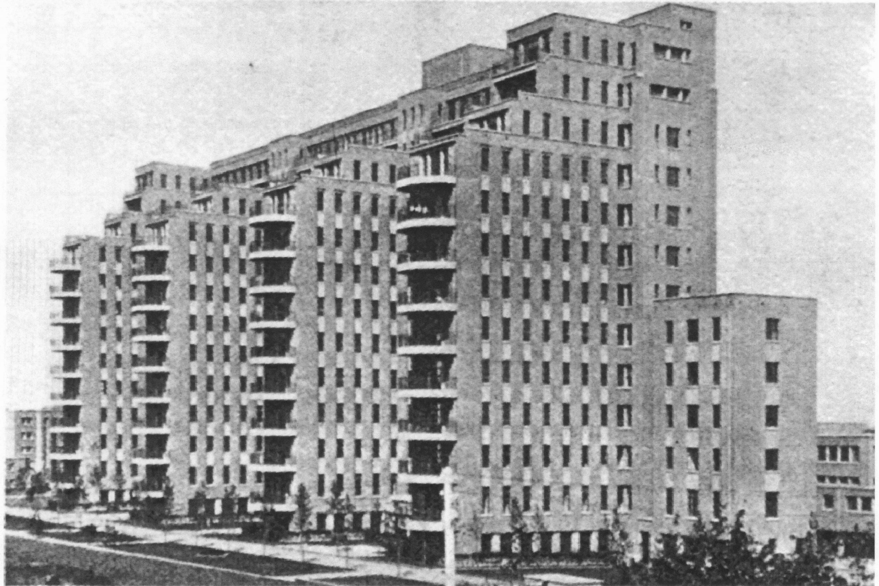
Figure 63. Beaujon Hospital, Clichy, France (Thompson and Goldin: 1975: 197).
