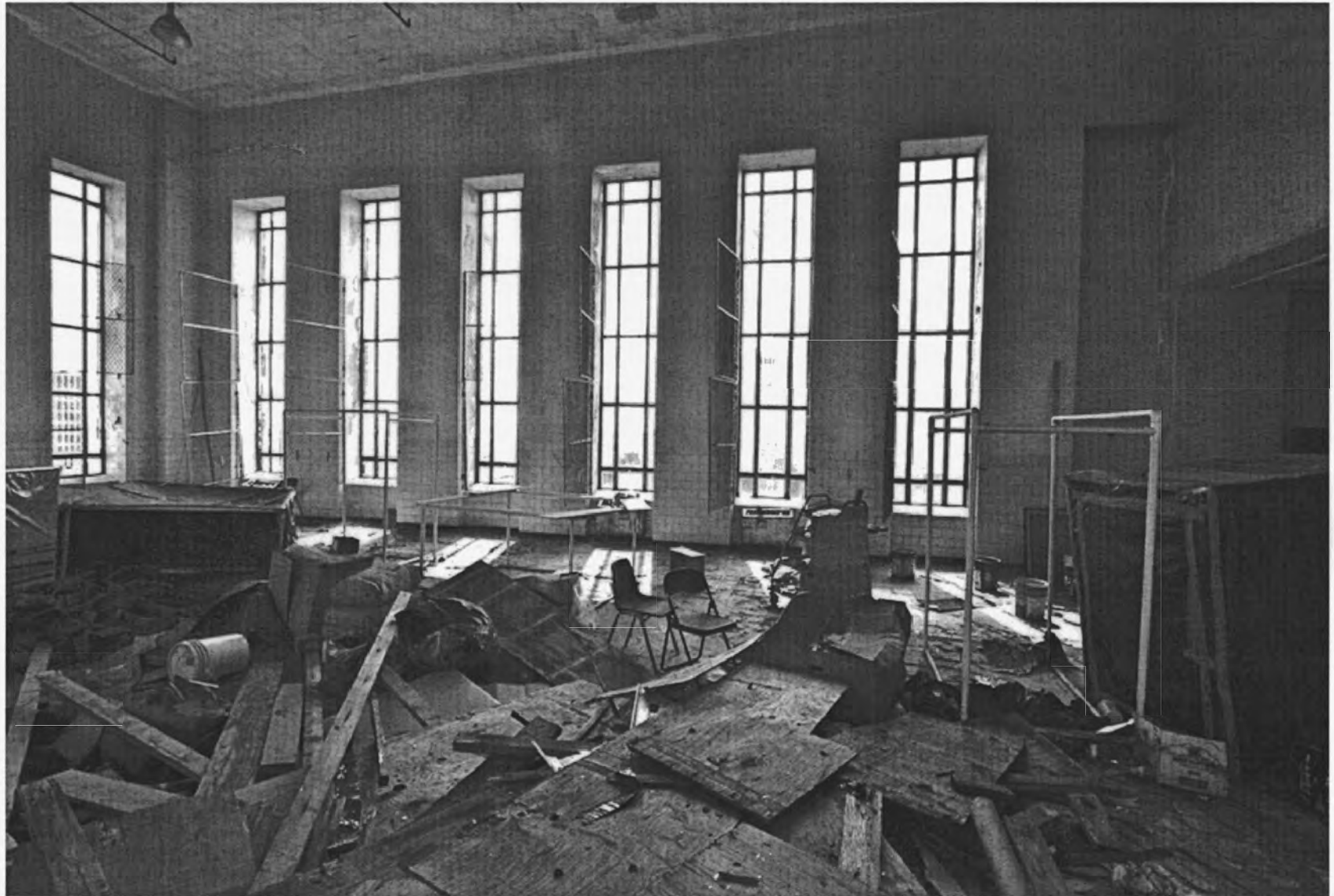
Figure 21. Charity Hospital, Gymnasium windows (Charity Hospital Engineering and Drafting Department).
