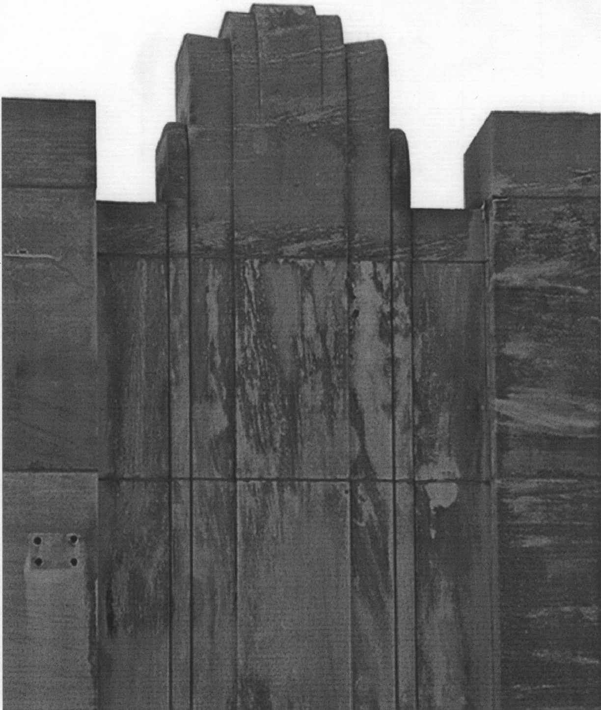
Figure 20. Charity Hospital, Limestone merlon capping on the parapet (FEMA).
