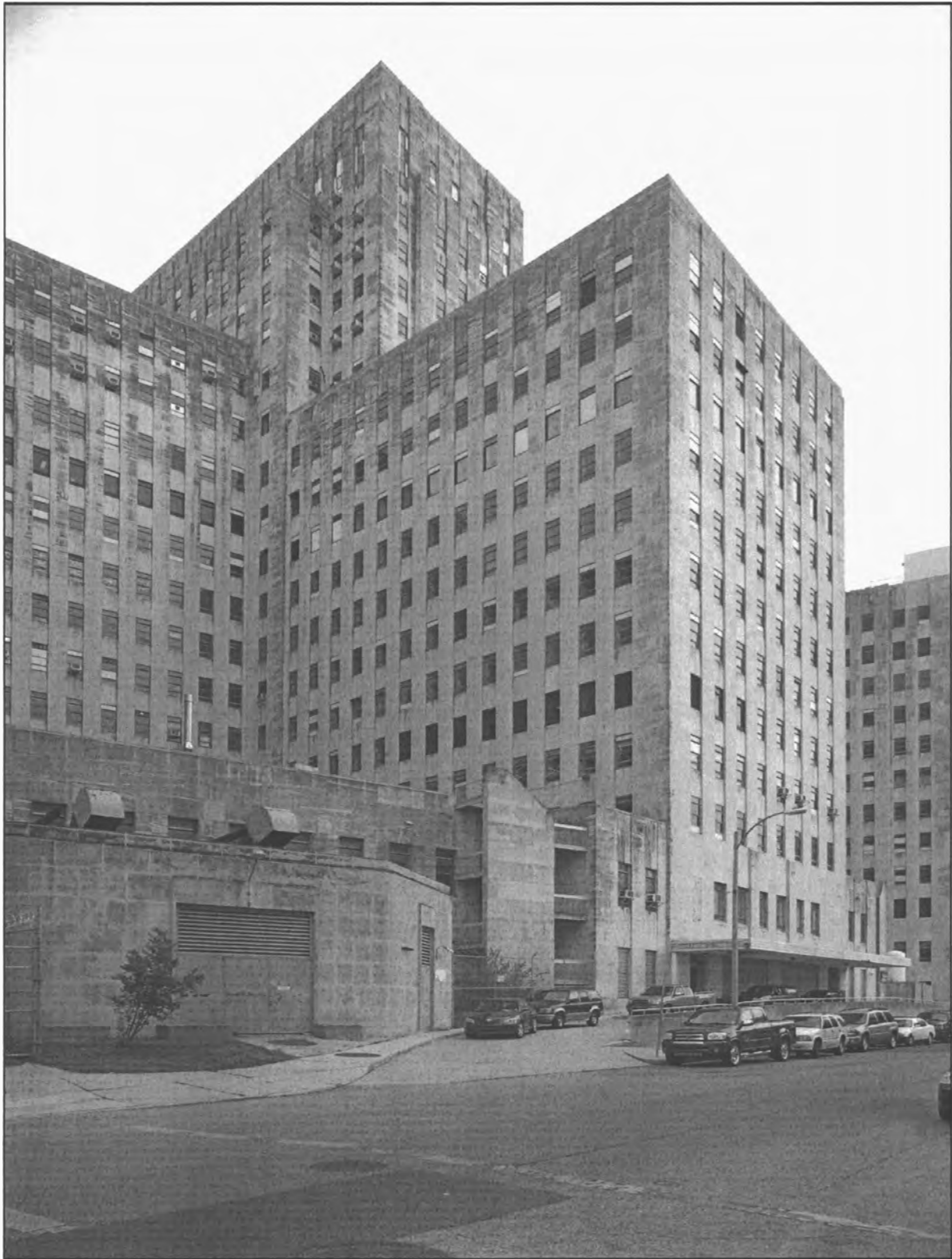
Figure 26. Charity Hospital, Rear elevation at Gravier Street (Robert Tucher, July 2009).
