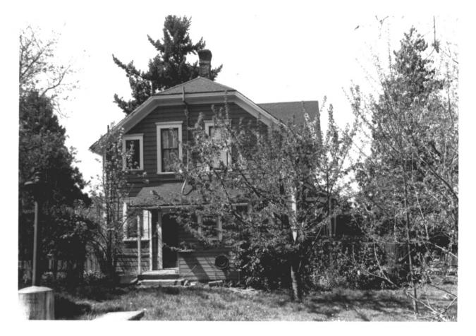
6 of 14 Southeast (rear) elevation showing clipped gable, original, corbelled chimney stack, simple, shed-roofed porch.
