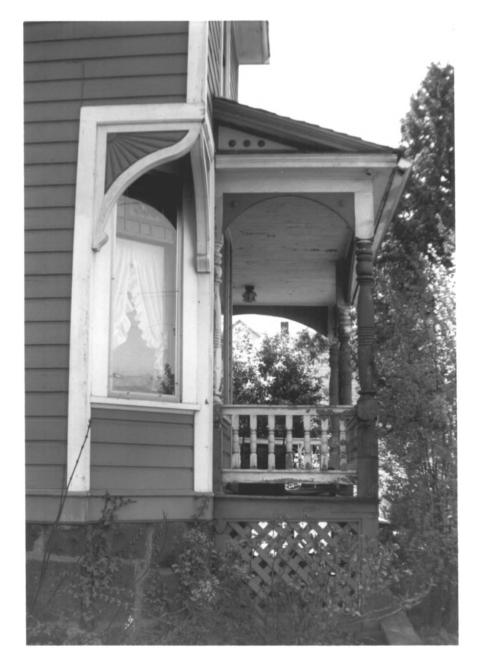
3 of 14 End view of front porch from the Northeast showing beveled window with canopy of solid S-curve brackets.
