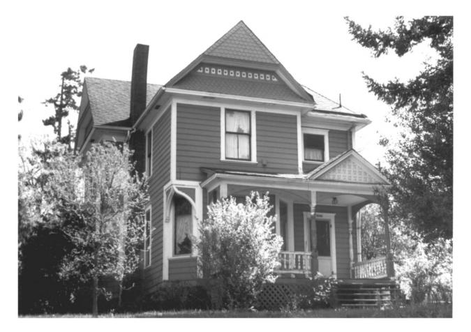
l of 14 Northwest (front) elevation, showing fish-scale shingle siding with in gable end and relief pattern in porch pediment which are typical of the
