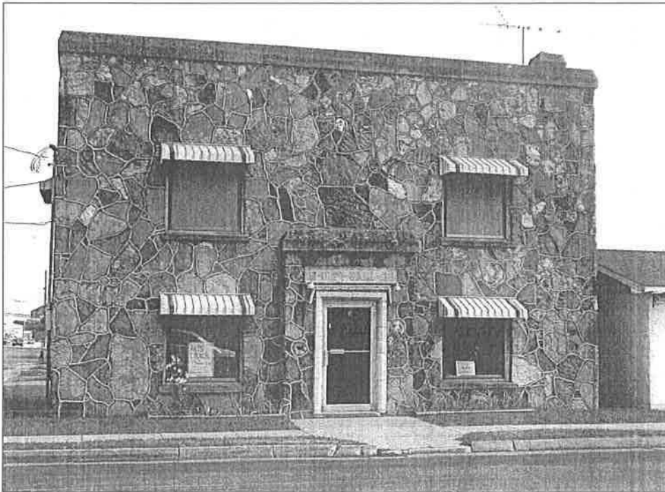
Figure 14: Photograph. Mountain Grove City Hall, Mountain Grove, MO. Constructed in 1938 as a WPA Project, it is a representative example of Ozark Rock Masonry architecture in a public government building. 2010. Source: Missouri State Historic Preservation Office (Jefferson City, MO)
