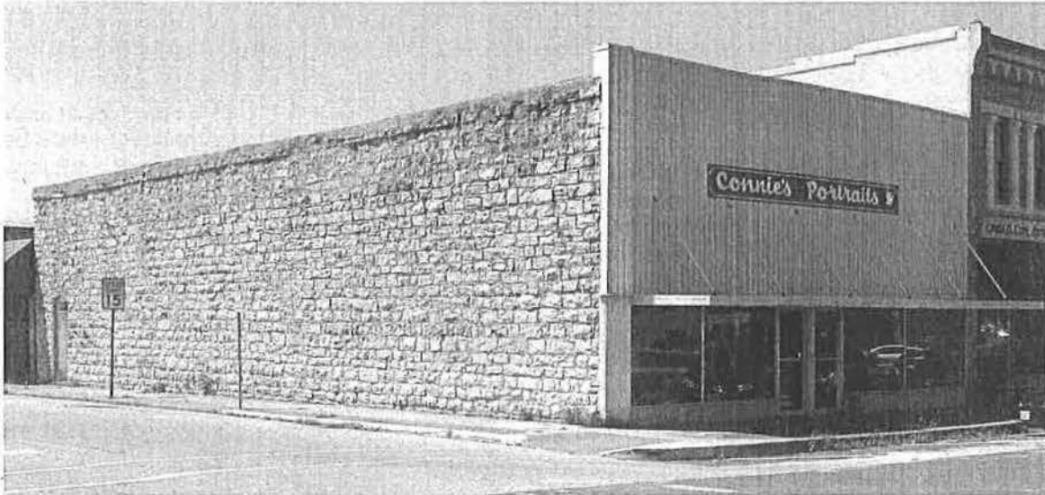
Figure 16: Photograph. Coarsed Rock Building, Marshfield, MO. Located at 108 East Madison Street. August 14, 2013. Richard Lee Burton.
