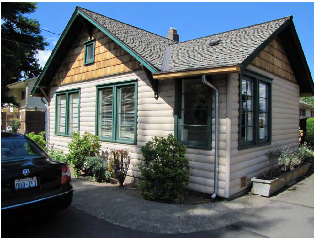
Si View Park – Caretaker's Residence 5 of 12
