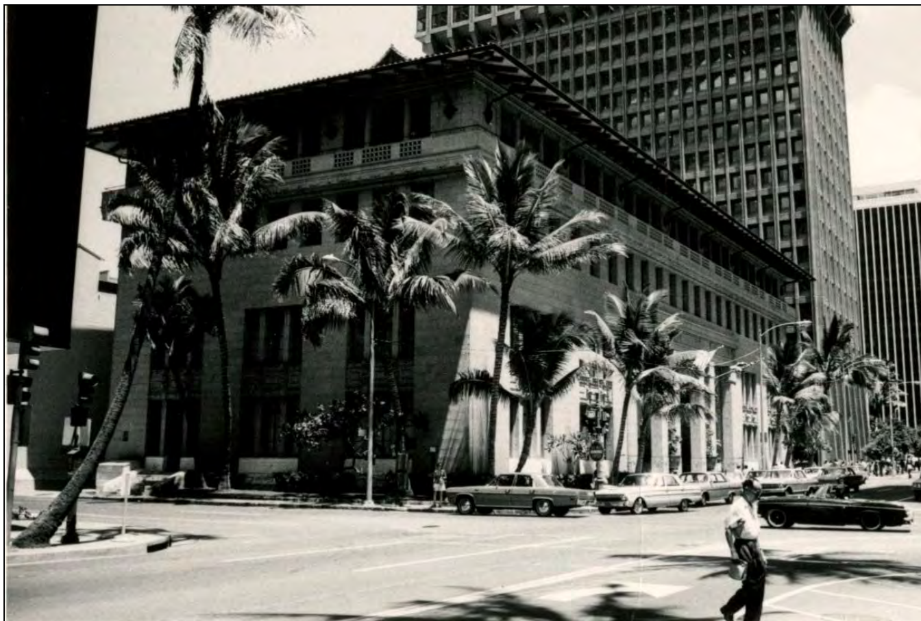
Figure 8-13. Photograph of the Alexander and Baldwin Building in downtown Honolulu, designed by C. W. Dickey in 1929. Source: Historic Hawai'i Foundation.
