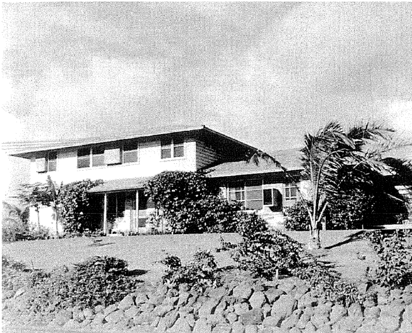
Figure 7-14. Photograph of Facility 77, ca. 1941. Note the retaining wall constructed of local rock. Source: Archives of NAVFAC Hawai'i, Joint Base Pearl Harbor-Hickam, Honolulu, Hawai'i, crediting the Archives of the USS Arizona Memorial, Honolulu, Hawai'i.
