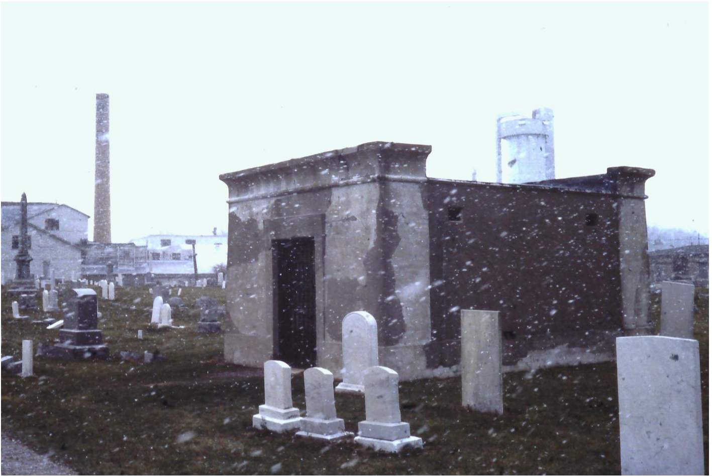
Vault prior to removal, ca. 1989
