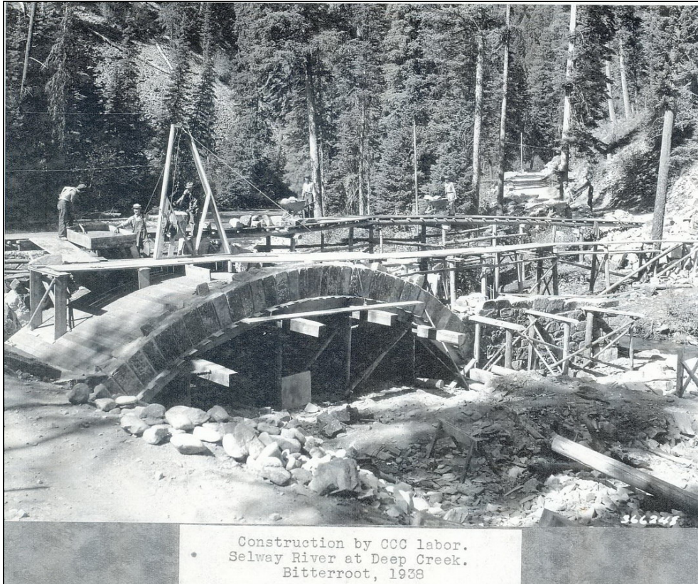
1938 photo of the Deep Creek Bridge under construction. (HF BNF)
