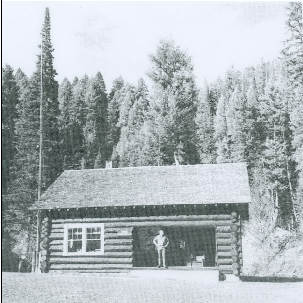
1963 photo of the east (front) wall of the combination building. Note the recessed loading dock, which should have been at the rear of the building. (HF BNF)
