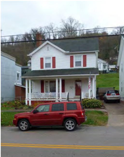
Colonial Revival infill
