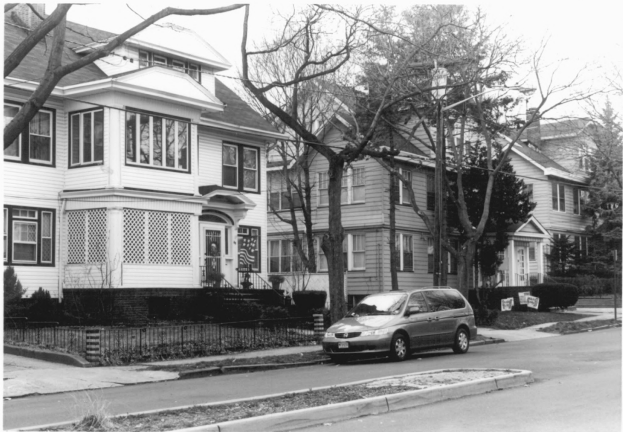
PHOTO 22 OF 76: WEEQUAMC PARK HISTORIC DISTRICT, NEWARK, ESSEX CITY, NJ
