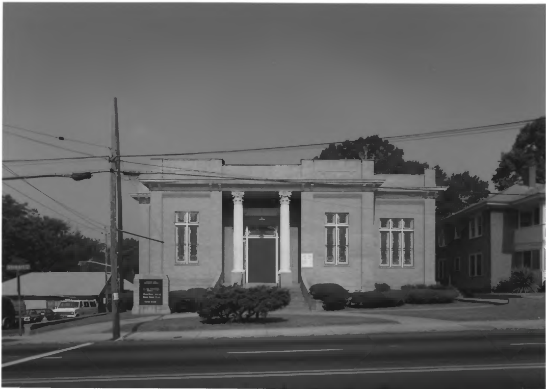
STEWART AVENUE Methodist Church Atlanta, Fulton County, Georgia # 1 of 7
