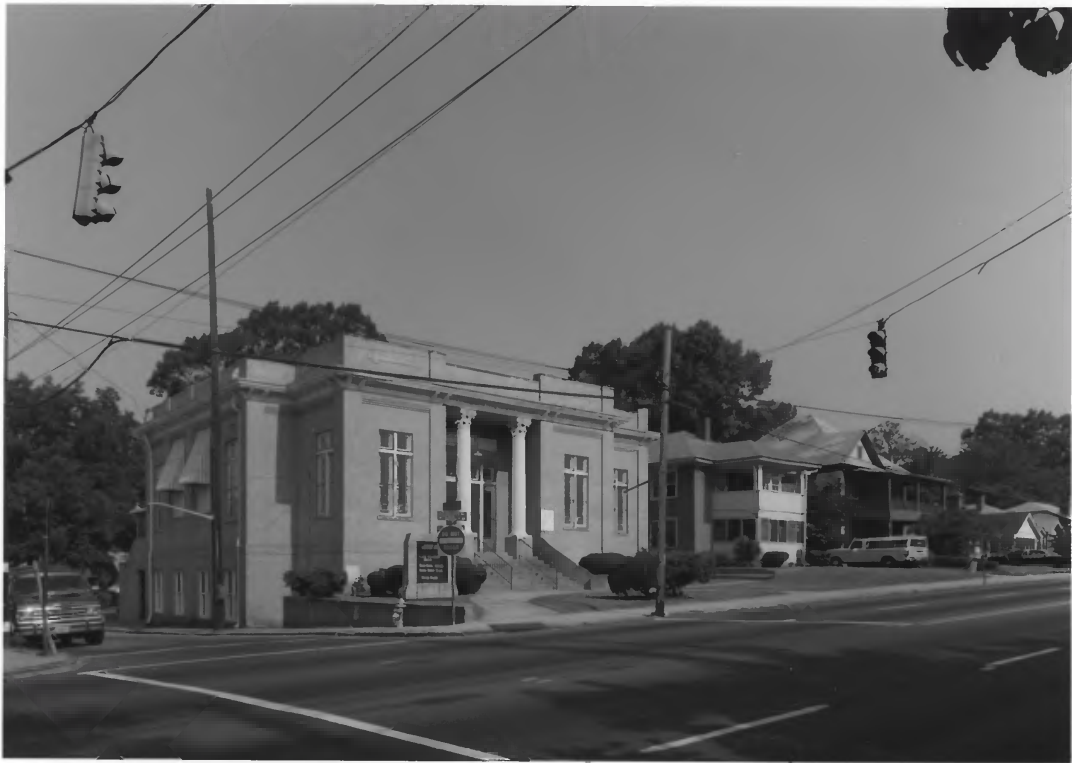
Stewart Avenue Methodist Church Atlanta, Fulton County, Georgia #2 of 7
