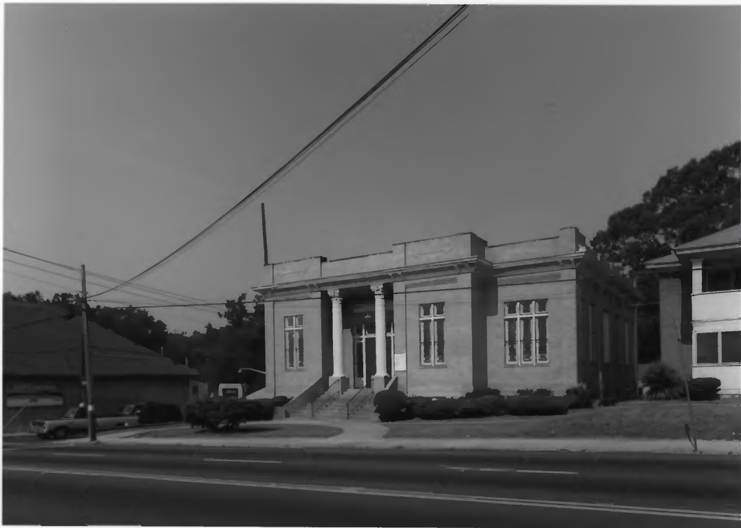
Stewart Avenue Methodist Church Atlanta, Fulton County, Georgia #3 of 7
