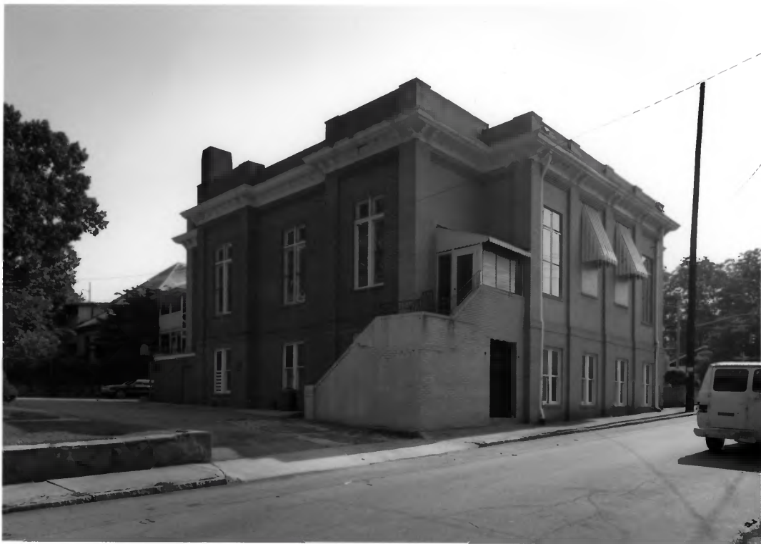
Stewart Avenue Methodist Church Atlanta, Fulton County, Georgia #4 of 7
