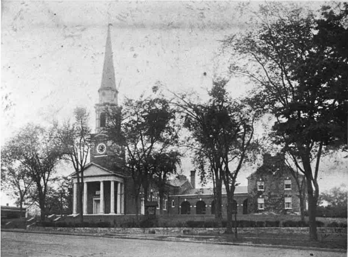
Historic Photo 1 – 1923 view of church complex, view to the west from Washington Street. This view most clearly shows the relationship of the three components of the Carrère and Hastings design: the main church sanctuary at left, the social hall/chapel in the center (with arched openings that have since been glassed in) and the administrative offices to the right. This view has since become obscured by vegetation between Washington Street and the church buildings. (Wellesley Congregational Church Archives)
