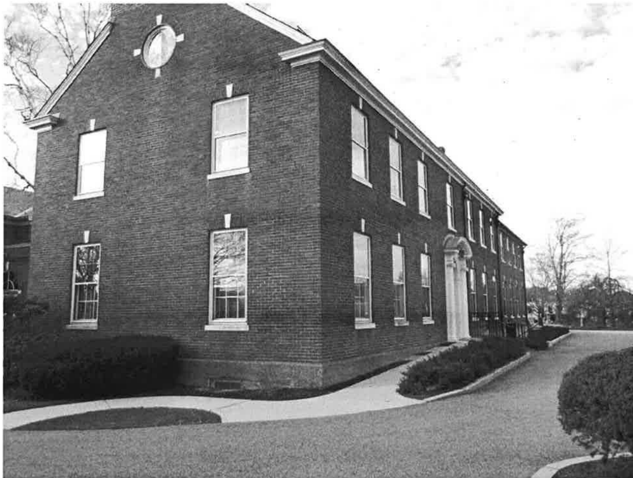
Photo 1 – Administrative offices from NE corner, view to the west, 2012.
