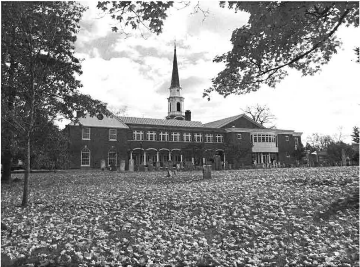
Photo 4 – Cemetery in foreground, Parish Hall in background, view to the east, 2012.
