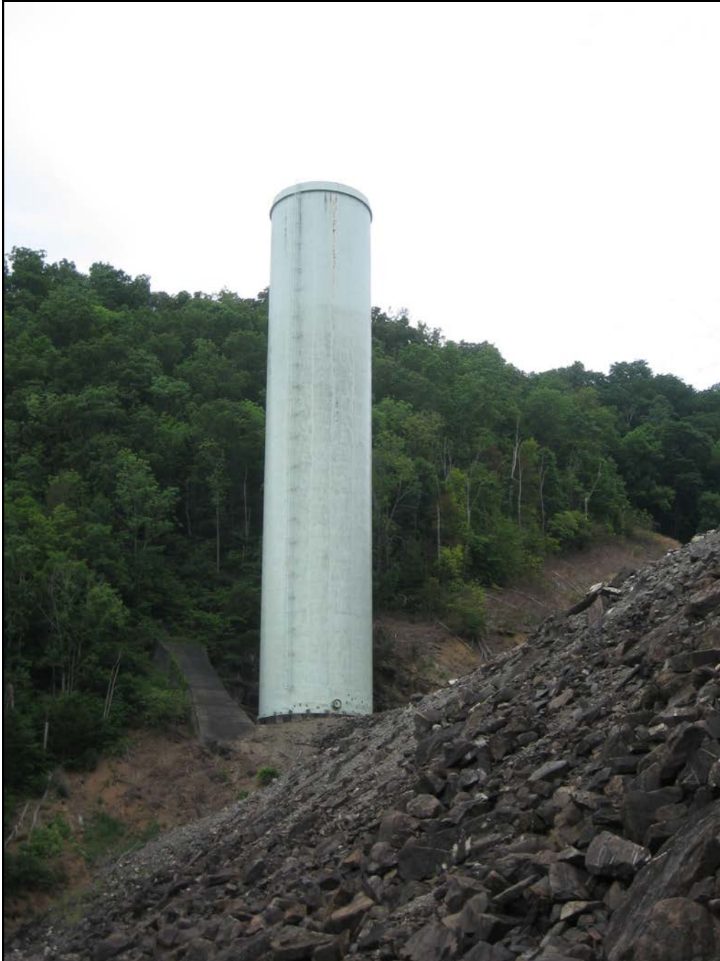
Figure 58: Surge tank at the South Holston project.
