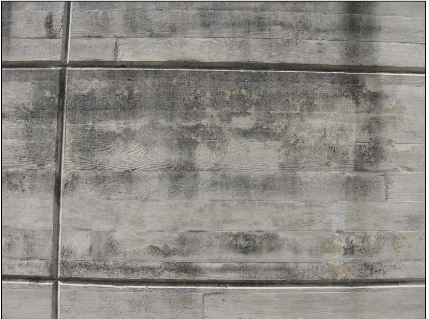
Figure 40: Board-form concrete exterior of the Chatuge Powerhouse.
