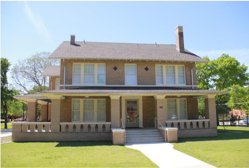
Photo 1 – North elevation, camera facing south porch (April 7, 2017)
