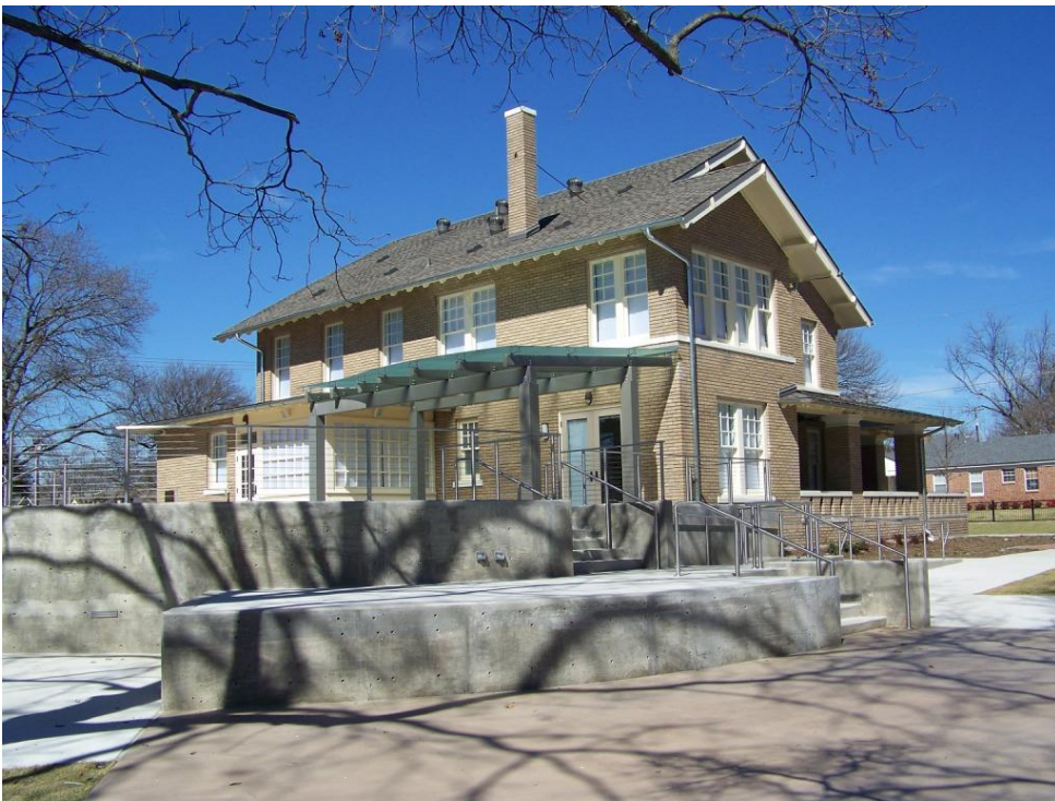
Photo 4 - Oblique view after renovation, showing south and east elevations, new canopy and new rear deck. Camera facing northwest. (February 22, 2017)
