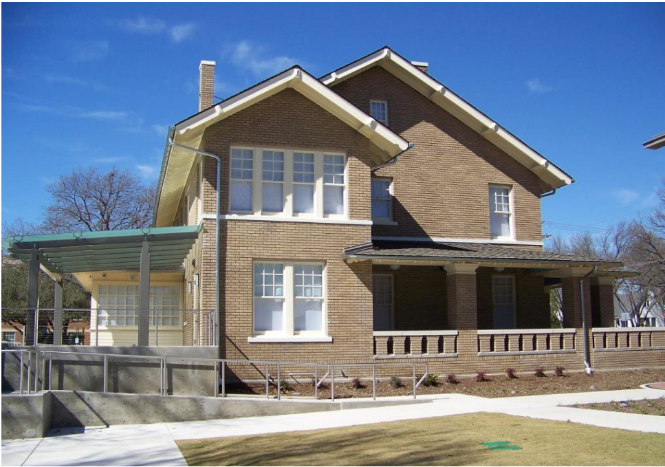
Photo 3 - East elevation after renovation, with restored side porch, new canopy and new rear deck. Camera facing west. (February 22, 2017)
