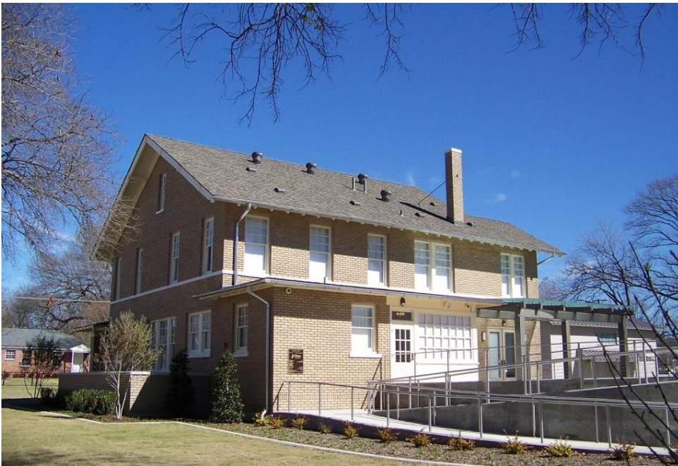
Photo 6 - Oblique view after renovation, showing west and south elevations, with new deck, new canopy and new screen wall for mechanical yard. Camera facing northeast. (February 22, 2017)
