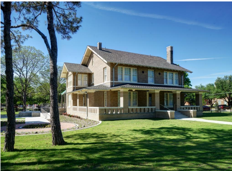
Photo 2 - Oblique view of front (north) and east elevations, with reconstructed front porch and and restored side porch. Camera facing southwest. (April 26, 2017)
