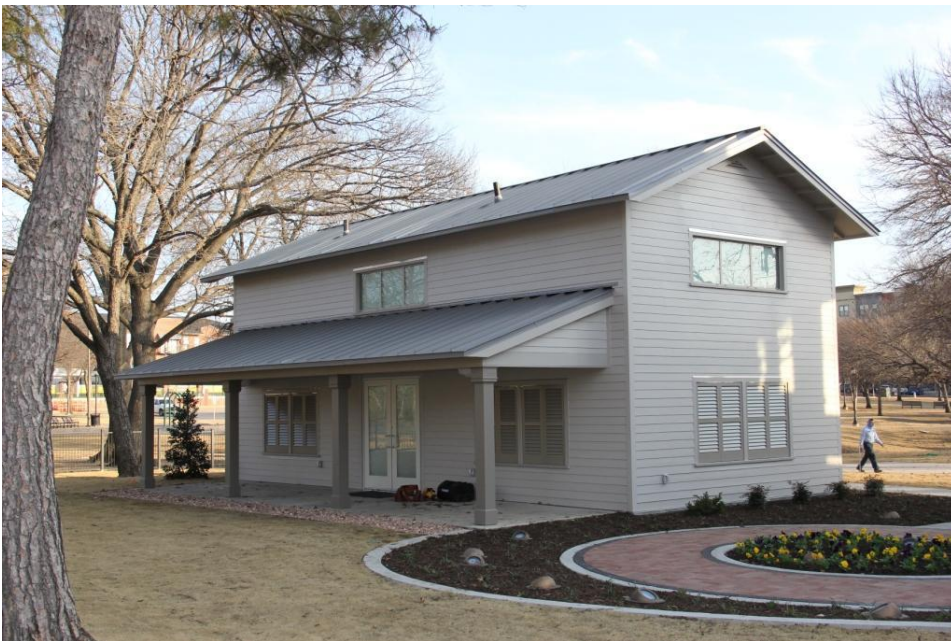
Photo 21 - Oblique view of the restroom building, showing front (north) and west elevations, and sculpture garden. Camera facing southeast. (February 22, 2017)
