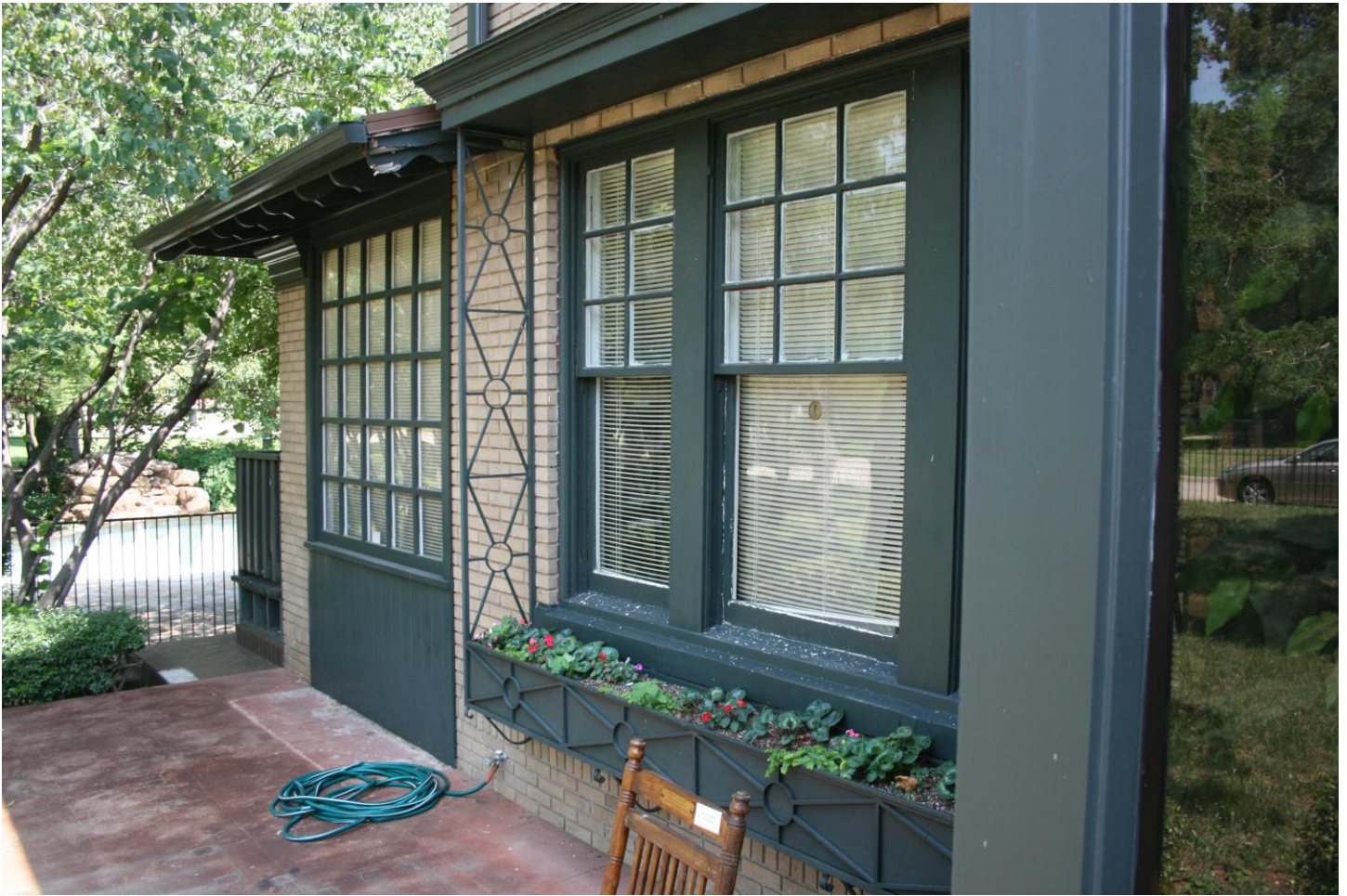
Figure 5 - Saigling House front elevation prior to recent renovation, showing enclosed side porch and front window box (June 2012).
