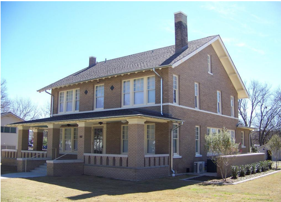
Photo 8 - Oblique view after renovation, with reconstructed front porch and new screen wall for mechanical yard. Camera facing southeast. (February 22, 2017)
