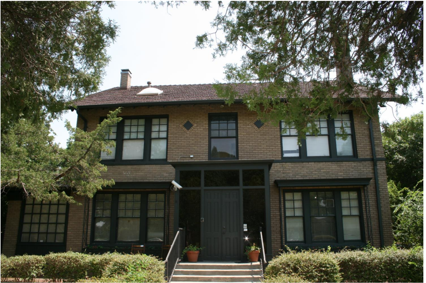
Figure 4 - Saigling House front elevation prior to recent renovation, showing the entrance vestibule and front window boxes (June 2012).
