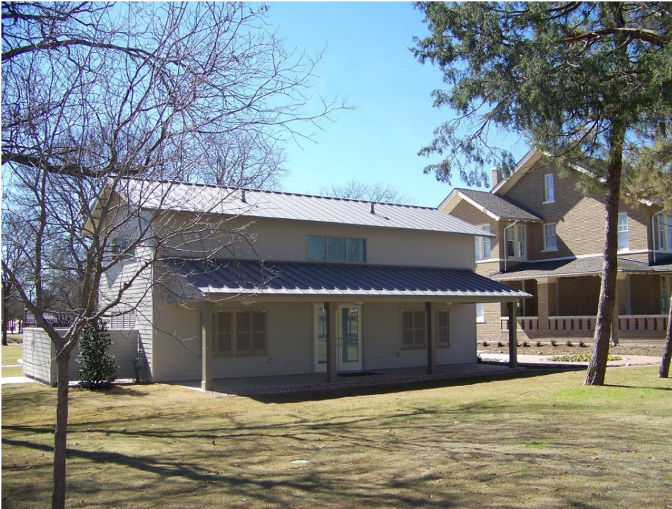
Photo 22 - Oblique view of the restroom building, showing front (north) and east elevations, with the Saigling House in the background. Camera facing southwest. (February 22, 2017)
