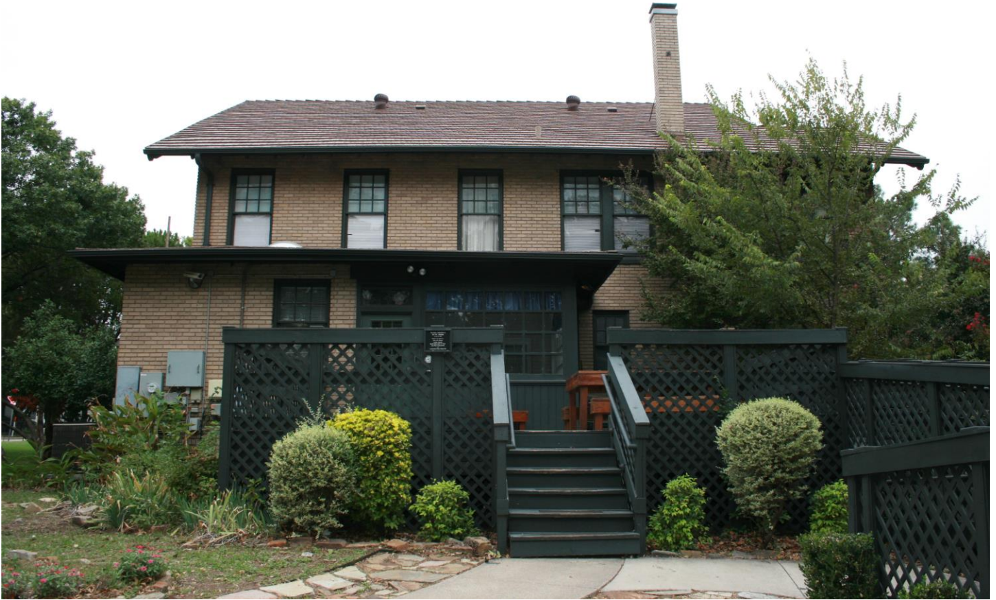
Figure 6 - Saigling House rear elevation prior to recent renovation, showing prior wood rear deck addition, and enclosed original rear (service) porch (October 2012).
