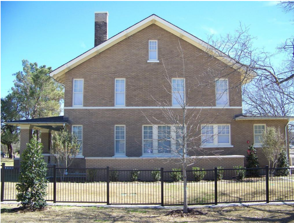
Photo 7 - West elevation after renovation, showing new screen wall for mechanical yard. Camera facing east. (February 22, 2017)
