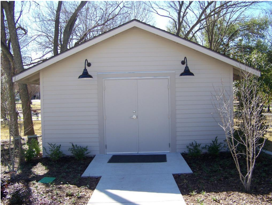
Photo 20 - Front (north) elevation of the storage building. Camera facing south. (February 22, 2017)
