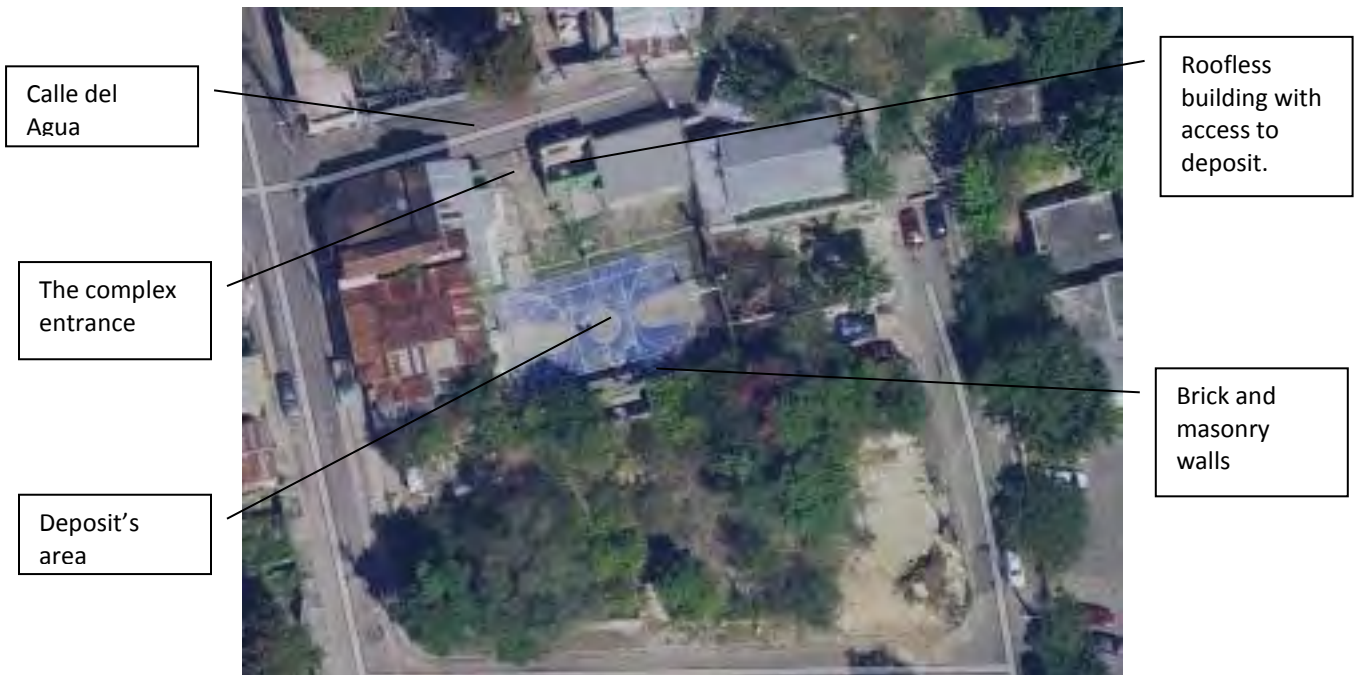
Figure 5. Aerial view of the deposit's area: the basketball court, the brick and masonry roofless building with sealed-off access to the deposit and the brick and masonry wall that surrounds most of the area.
