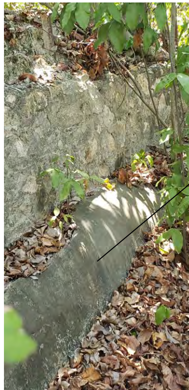
Figure 7. Photos show sections of the conduit channel showing construction material: brick, stone and hydraulic concrete for the outer shell, with the interior vault made of brick with a hydraulic cement grout. The conduit channel in the pictures below still retains parts of its outer fabric horseshoe vaulted component. (Juan Llanes, 2019)
