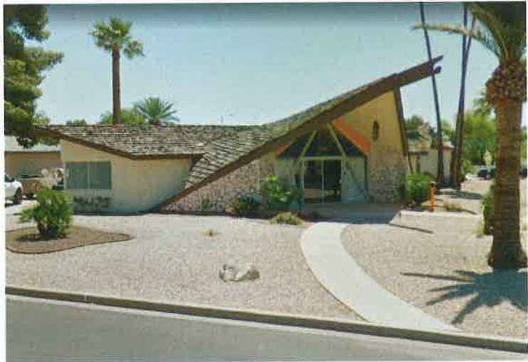
Figure 17. This home at the southeast corner of Pueblo and Saranac avenues was the sales office for the ACCE. The distinctive roofline was a feature of the then popular Polynesian styling, which also occurs in a simpler form on the home next door to the Ponderosa II (see Fig. 4).
