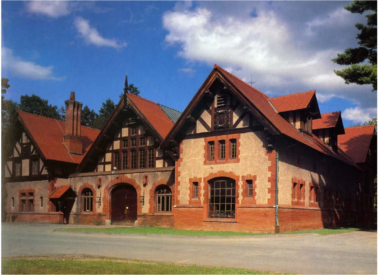
Supplemental Photo 13. Carriage house/garage, Frederick Vanderbilt National Historic Site, Hyde Park, New York, circa 1896. (Hewitt, The Architect and the American Country House ).
