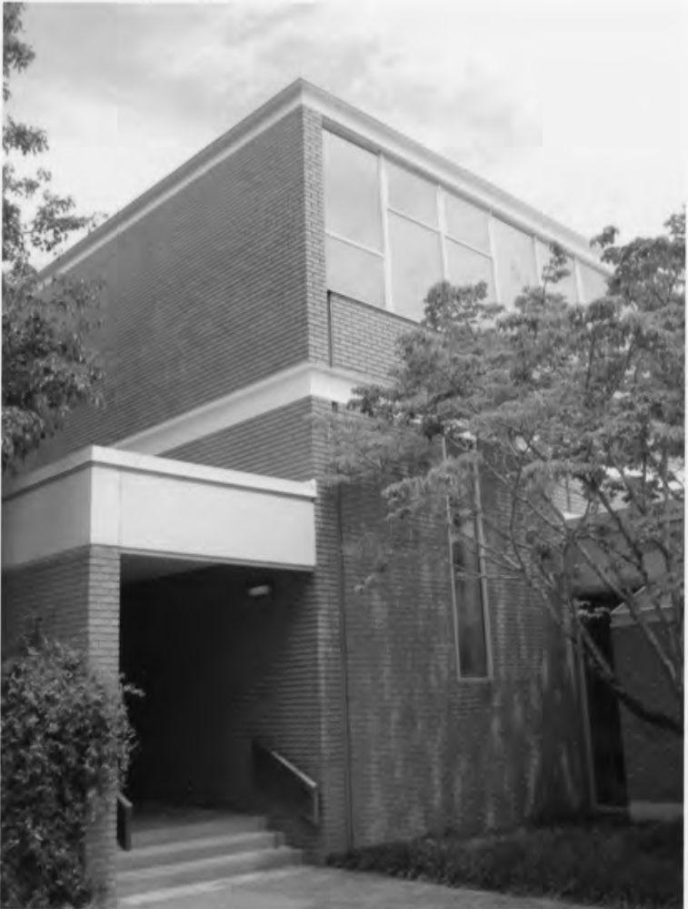
South Wall of 1991 Tower Addition
