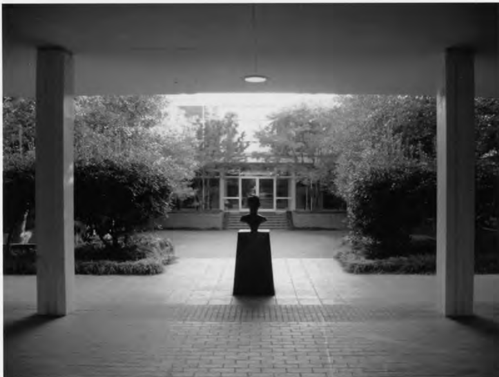
R03. Structural Science Building (Lee Hall / Lowry Hall) Clemson University Pickens County, S.C.
