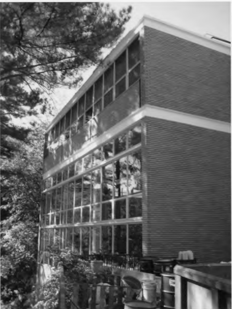
Lowry Hall, East Elevation, Civil Engineering Laboratory Wing
