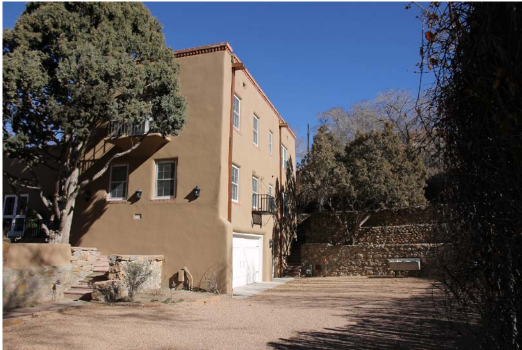
12 of 22. Main and East Facades, photographer facing northeast.
