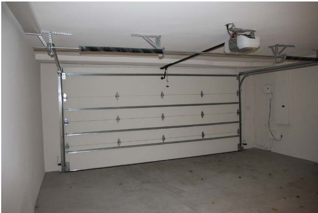
20 of 22. Garage in Basement Level, photographer facing southeast.
