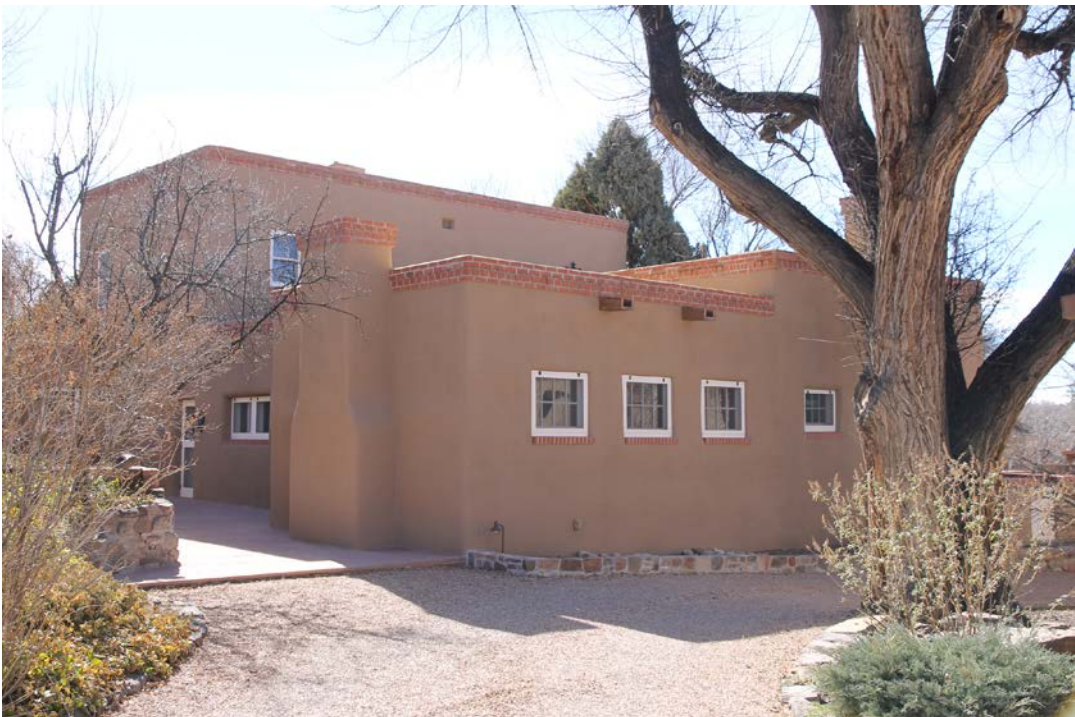
8 of 22. West and Rear facades, photographer facing southeast.
