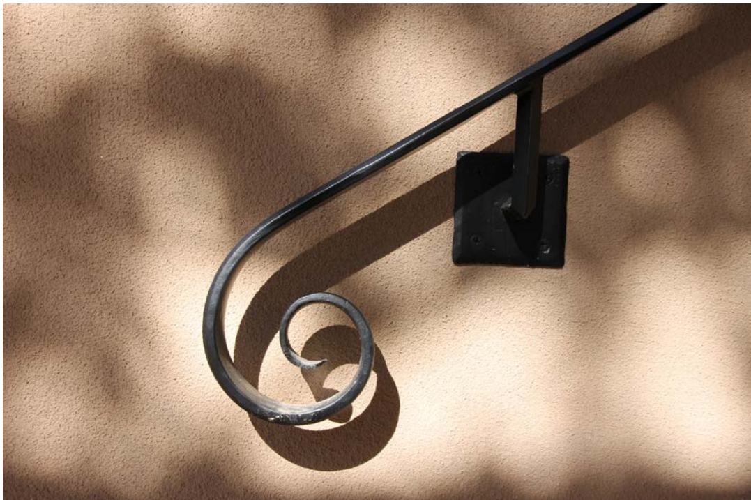
14 of 22. Detail of Iron Handrail on East Facade, photographer facing west.
