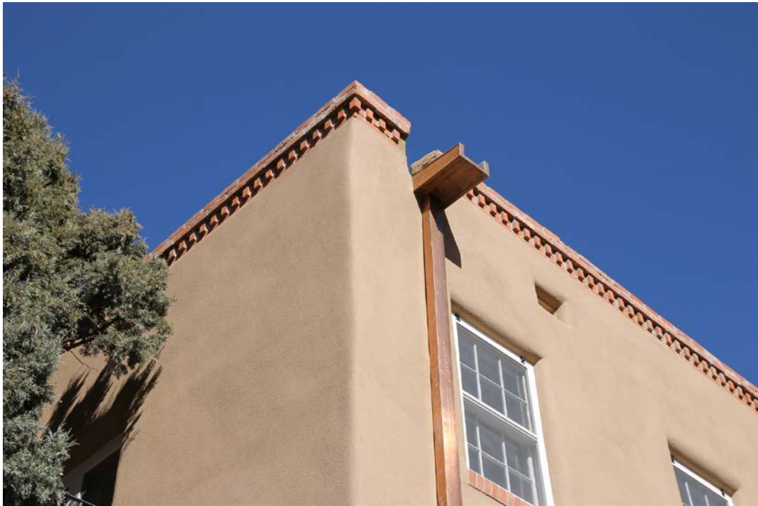
13 of 22. Detail of Brick Dentil Cornice, photographer facing northwest.
