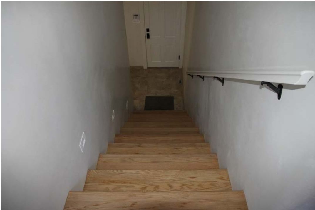
19 of 22. Stairs to Basement Level and Garage, photographer facing south.
