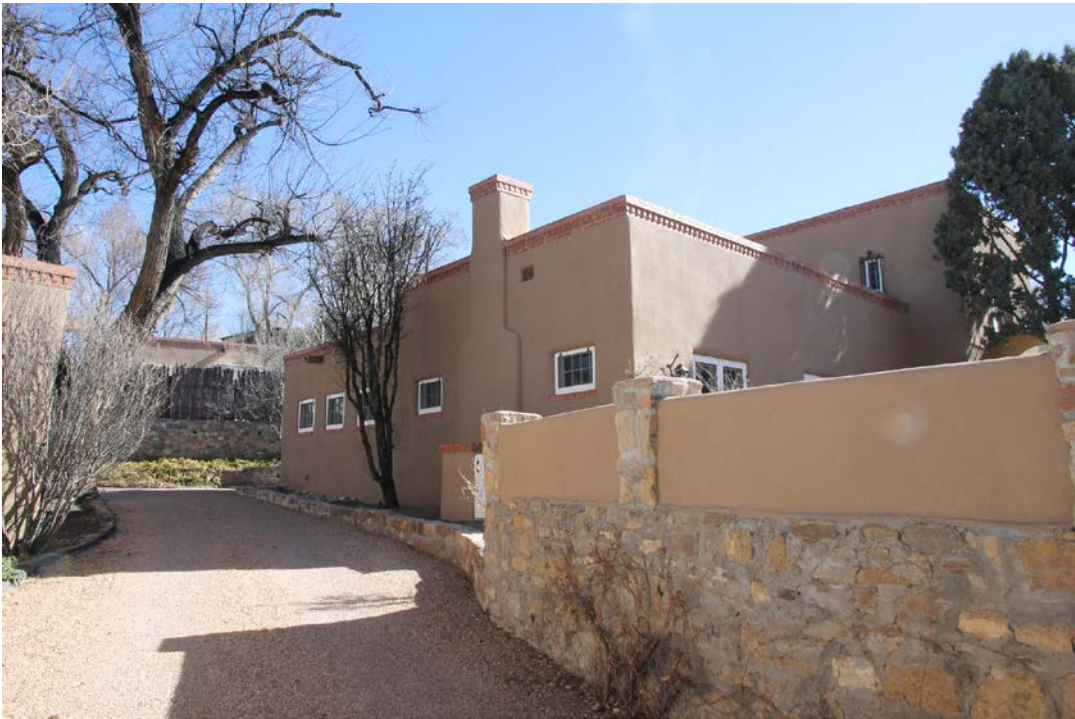
7 of 22. West and Main Facades, photographer facing northeast.
