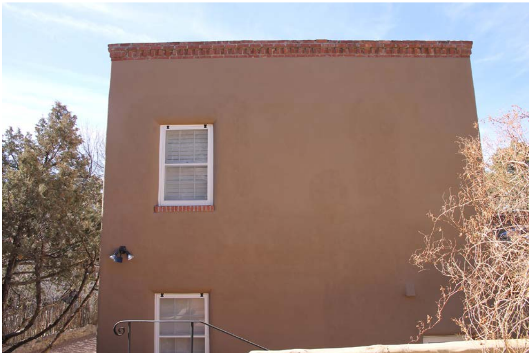
10 of 22. Rear façade of Bedroom Block from atop Guest Apartment, facing south.
