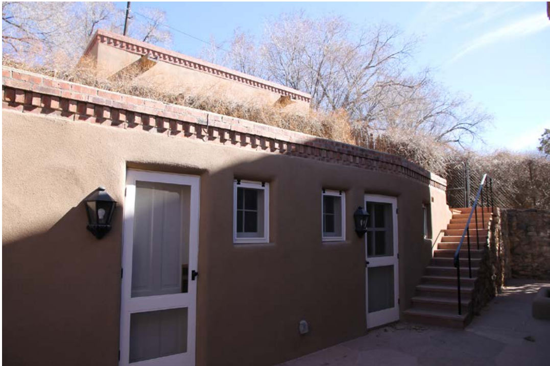
9 of 22. Guest Apartment north of the main house, photographer facing northeast.
