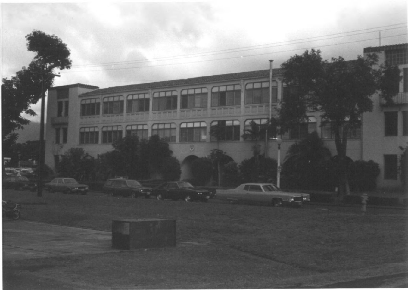
Enlisted men's barracks, Wheeler Air Force Base, 1983.
