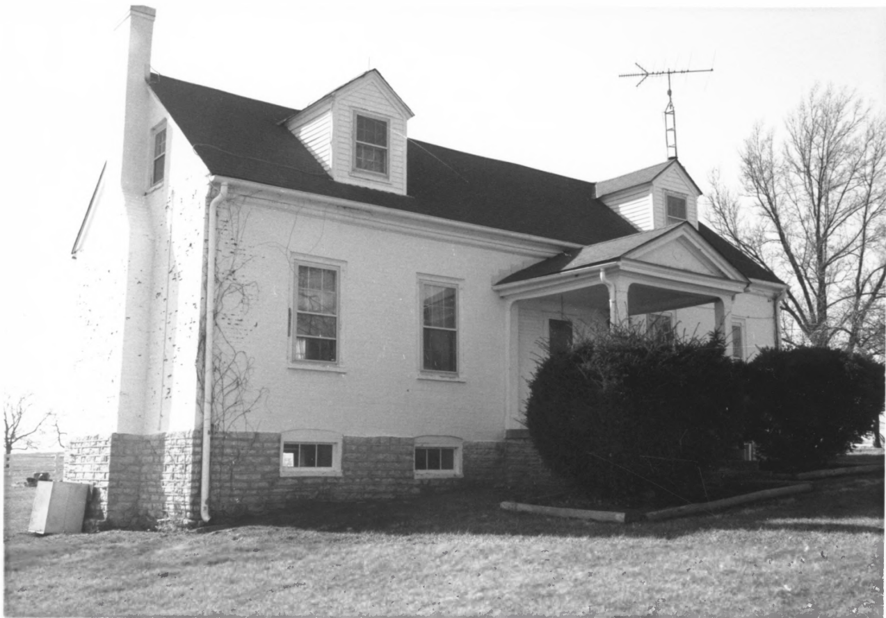
WEST FAYETTE COUNTY RURAL HISTORIC DISTRICT, KY. PHOTO 13
