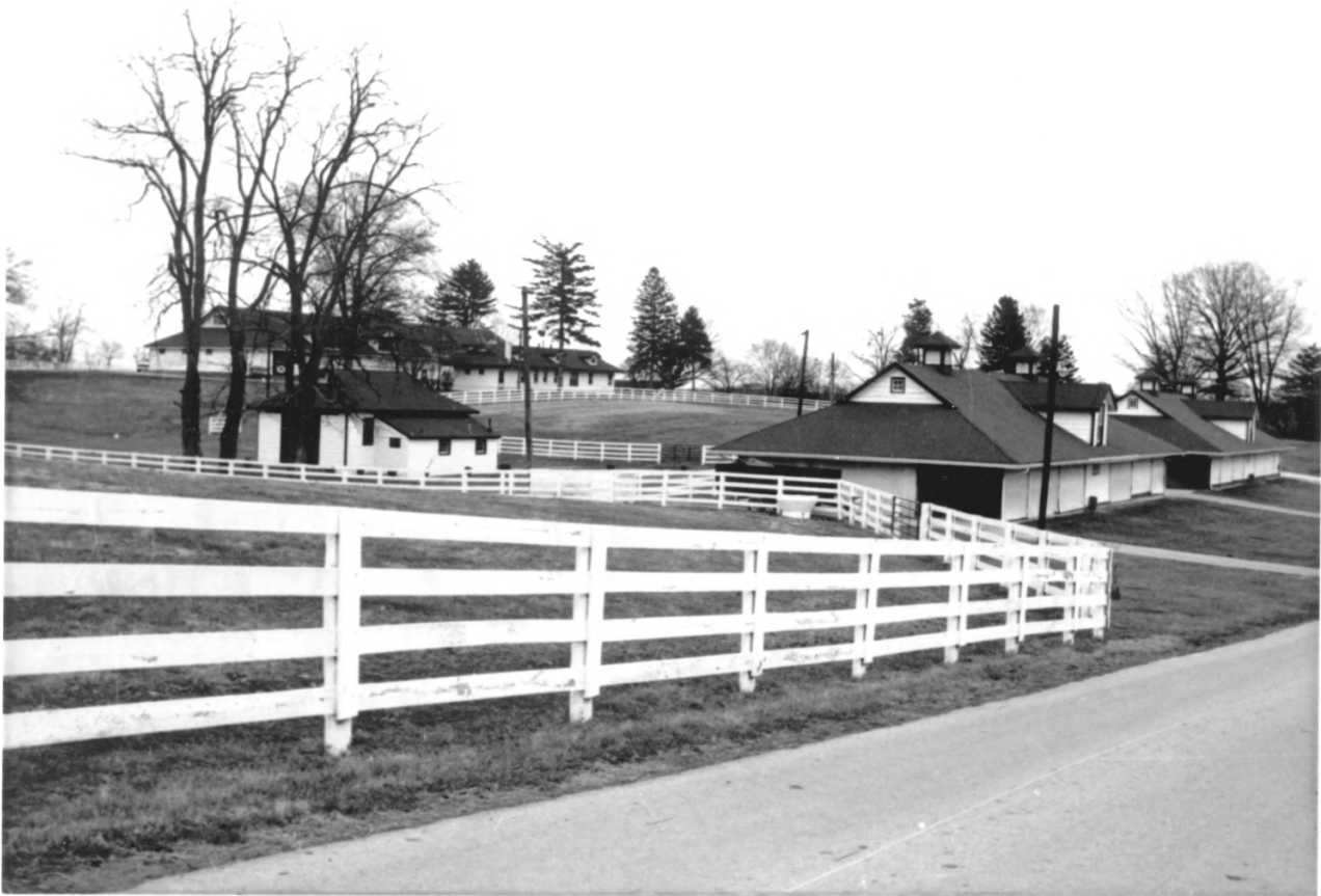
WEST FAYETTE COUNTY RURAL HISTORIC DISTRICT , KY.
