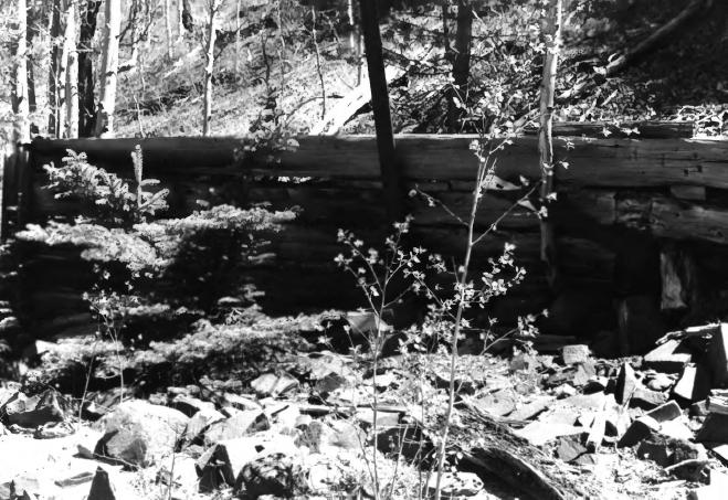
Figure 2: Feature 2, the wood retaining wall. This view was made south of the wall looking north. In the foreground is a portion of the rock foundation.
