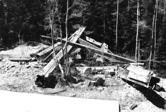
Figure 5: Feature 5, the collapsed hoist tower. At the far end of the long beam is the pulley and cable which cannot be seen in this picture. The view was made on top of the tailings pile, looking south with part of the slab over the shaft seen in the foreground.
