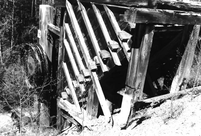
Figure 9: Feature 8, the stamp mill, as seen from the road above the mill. This shows the large hopper which stands above the machinery. The large wheel on the east side of the mill is seen and above and to the right of the wheel are the long iron rods to which the pistons are attached. This view is looking in a southeasterly direction.
