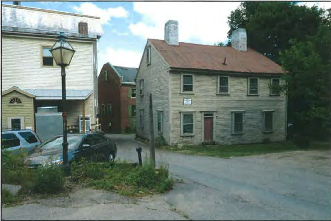
Photo 3: View southeast at north and west elevations of Dummer House from Dummer Lane. SCC, June 2017.
