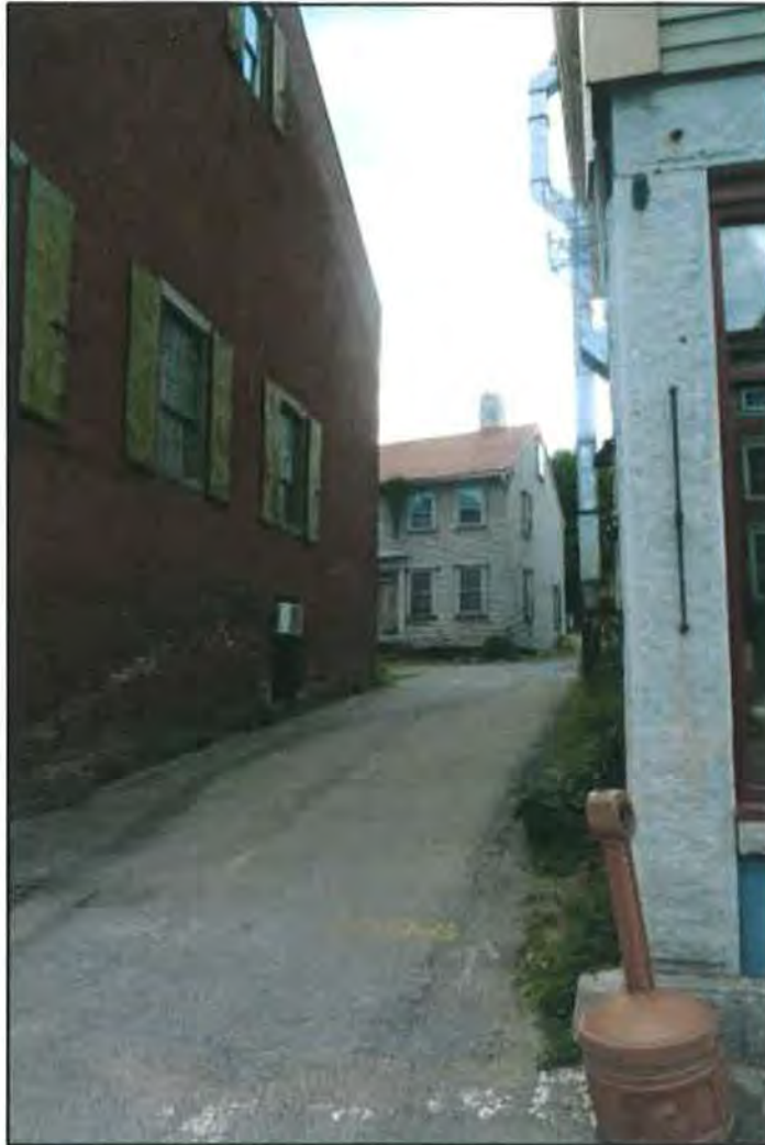
Photo 7: View of Dummer House from Water Street. SCC, June 2017.
