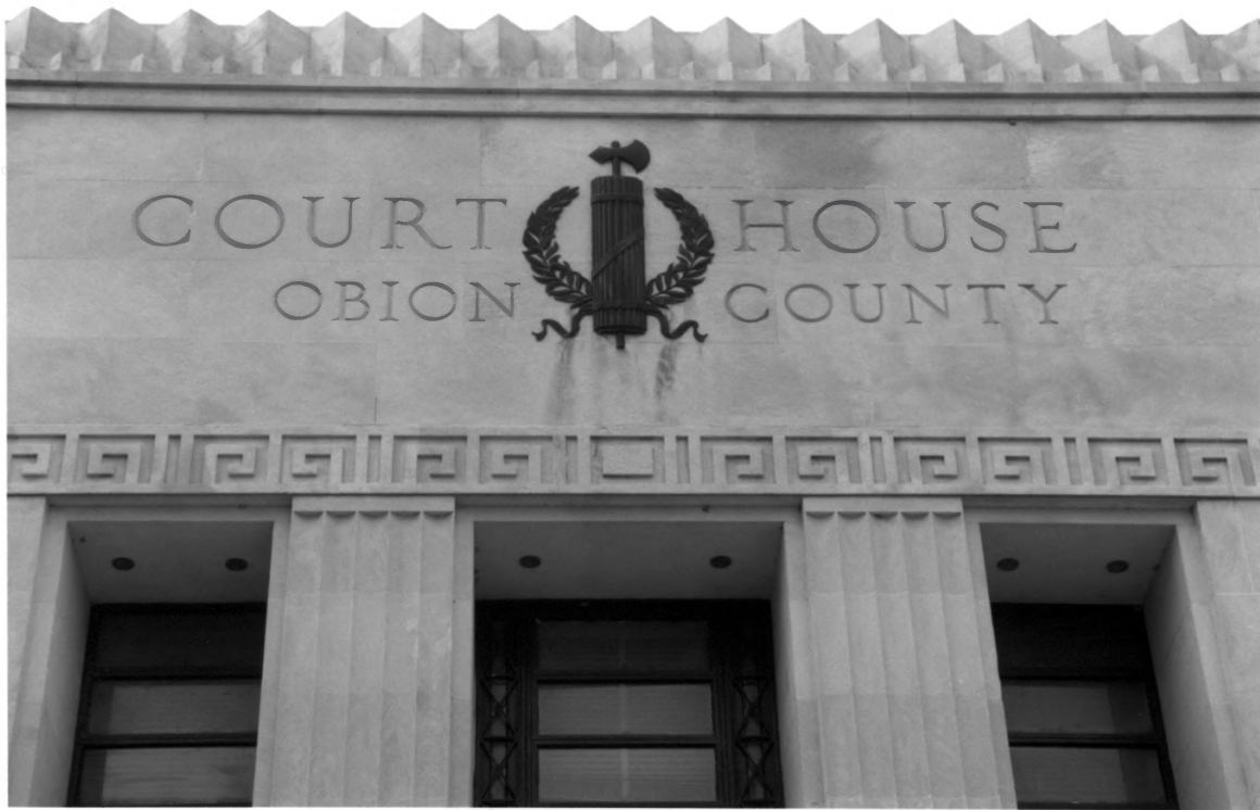
OBION COUNTY COURTHOUSE OBION COUNTY TN
