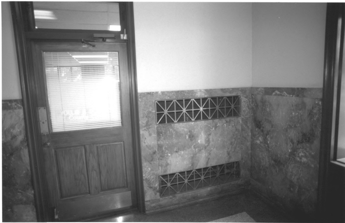
OBION COUNTY COURTHOUSE OBION COUNTY TN
