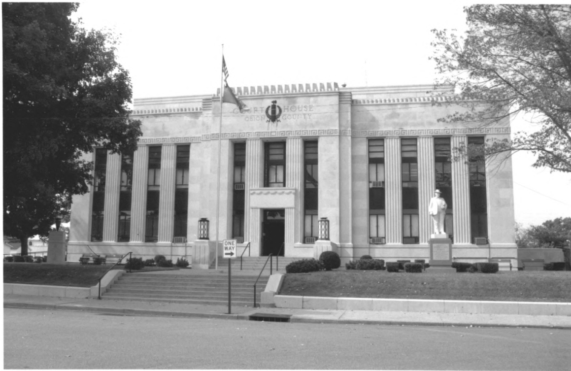
OBION COUNTY COURTHOUSE OBION COUNTY TN
