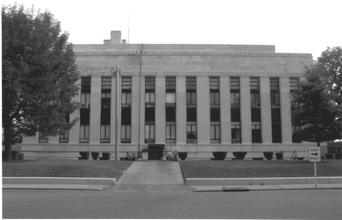
OBION COUNTY COURTHOUSE OBION COUNTY TN
