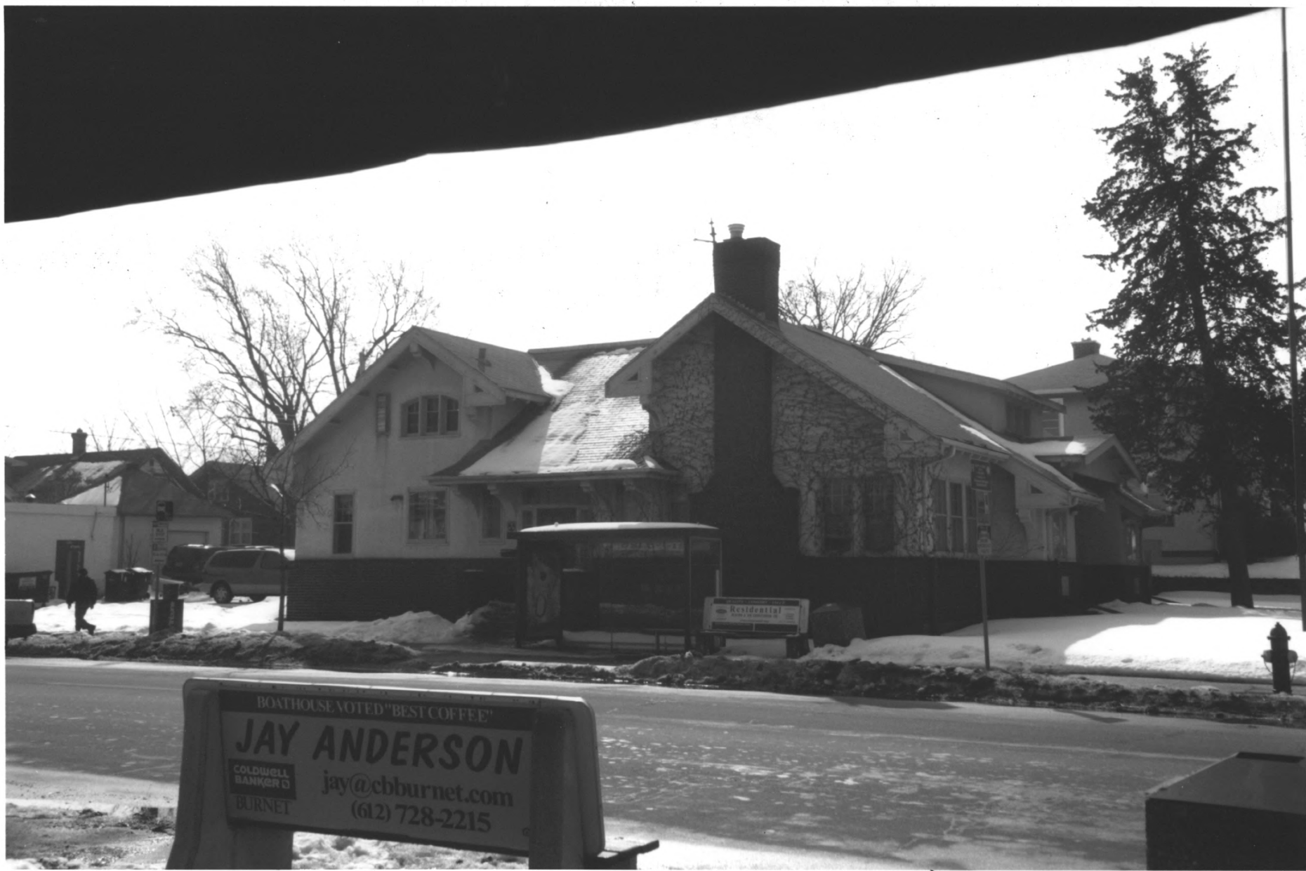
Station 13 Minneapolis Fire Department (MFD) Henne pin Co., Mn 014559-36A
