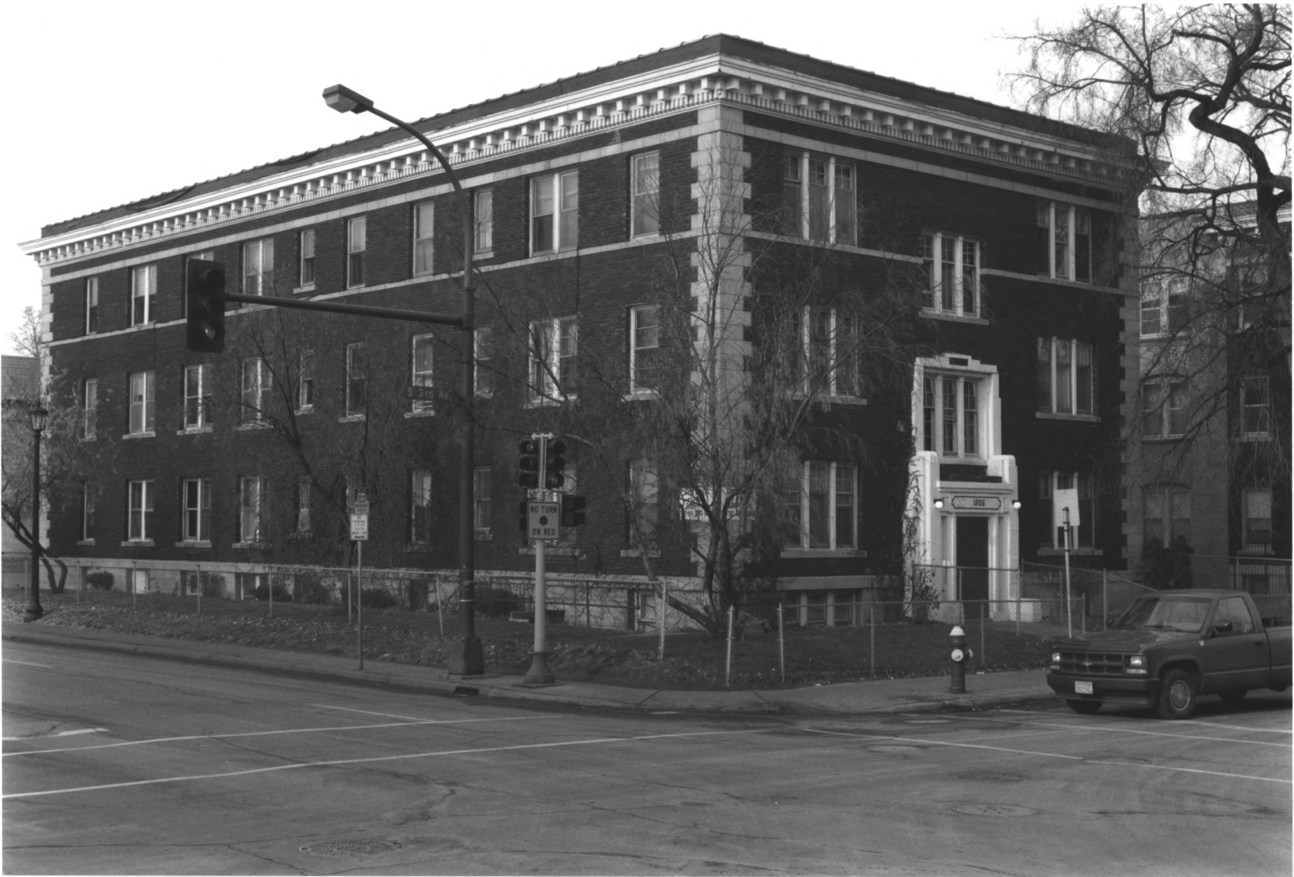
1926 3RD AVE. S. STEVENS SQUARE HISTORIC DISTRICT MINNEAPOLIS, HENNEPIN CO., MINNESOTA #011516-22A
