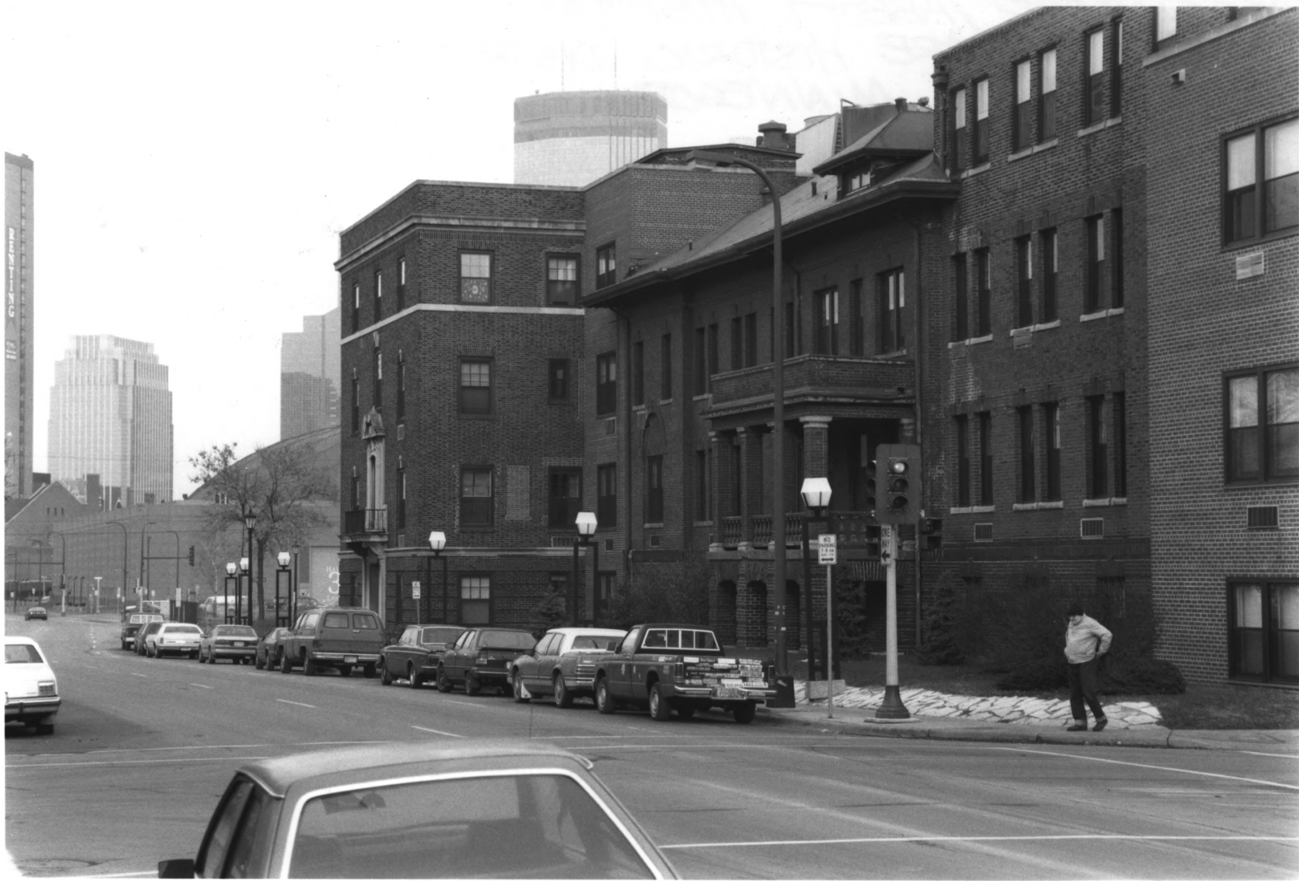
STREETSCAPE/ABBOTT HOSPITAL/1ST AVE. S. STEVENS SQUARE HISTORIC DISTRICT MINNEAPOLIS, HENNEPIN CO., MINNESOTA #011514-7
