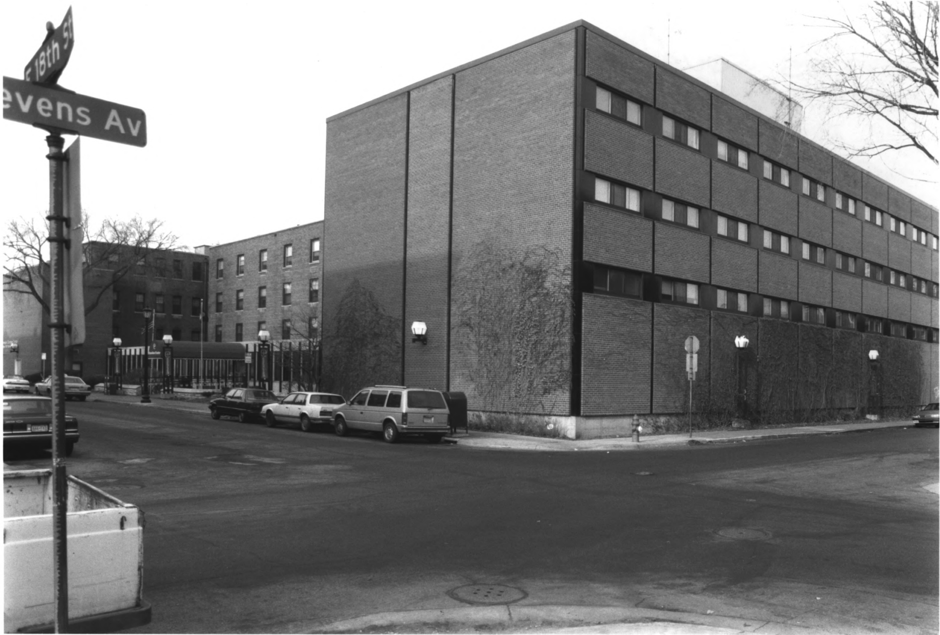
ABBOTT HOSPITAL- 1711-25 1ST AVE. S. STEVENS SQUARE HISTORIC DISTRICT MINNEAPOLIS, HENNEPIN CO., MINNESOTA #011499-19
