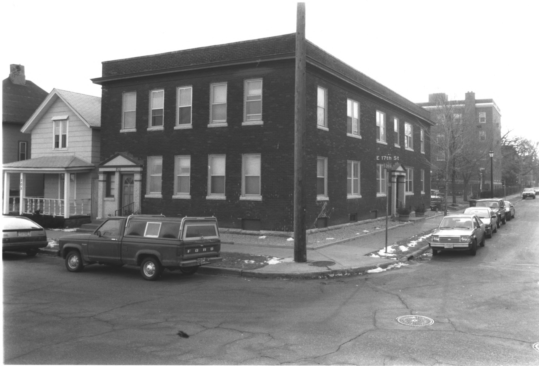
203 E. 17TH ST. STEVENS SQUARE HISTORIC DISTRICT MINNEAPOLIS, HENNEPIN CO., MINNESOTA # 511516-0A
