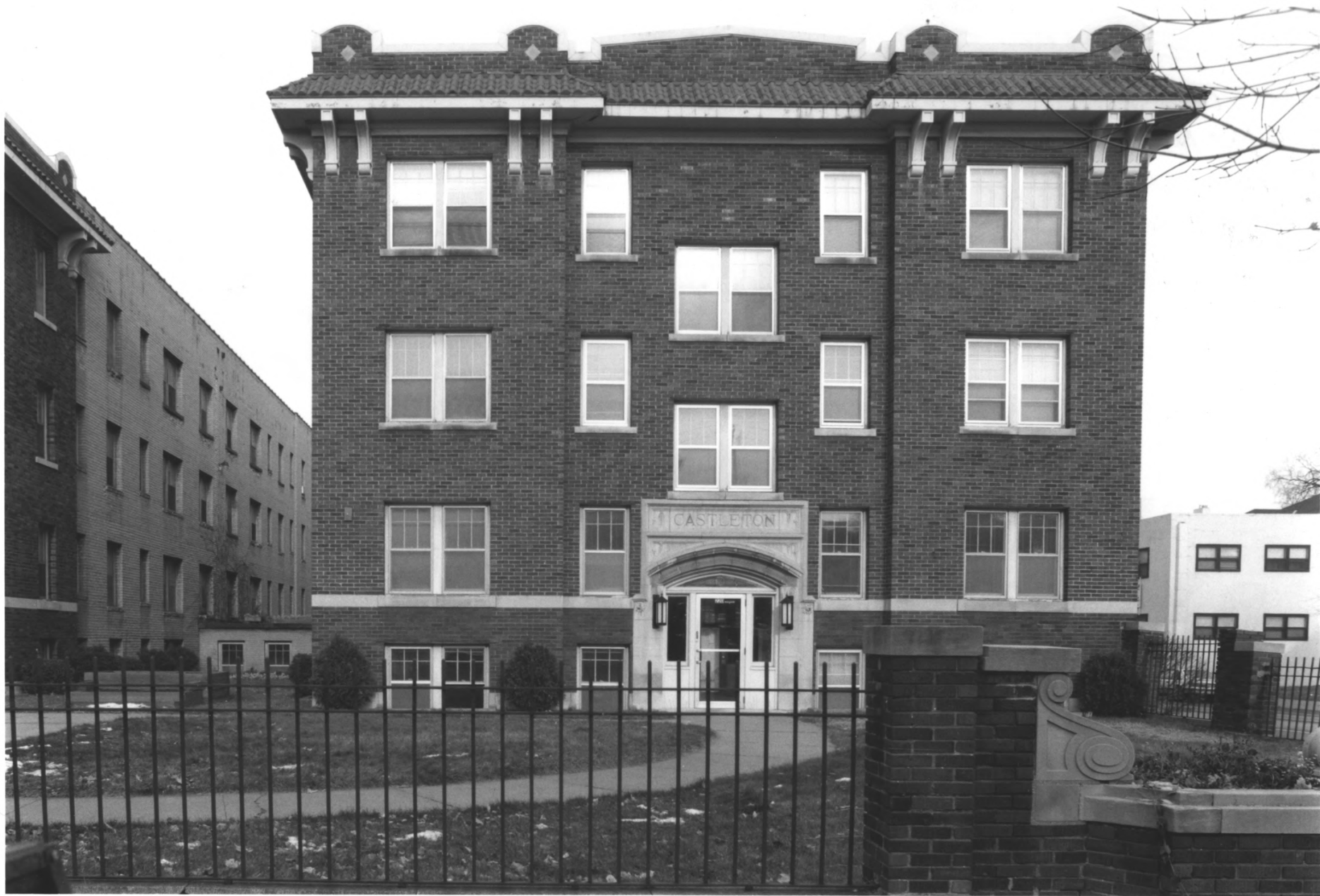
THE CASTLETON - 220 E. 19 TH ST. STEVENS SQUARE HISTORIC DISTRICT MINNEAPOLIS, HENNEPIN CO., MINNESOTA #011516 - 11A
