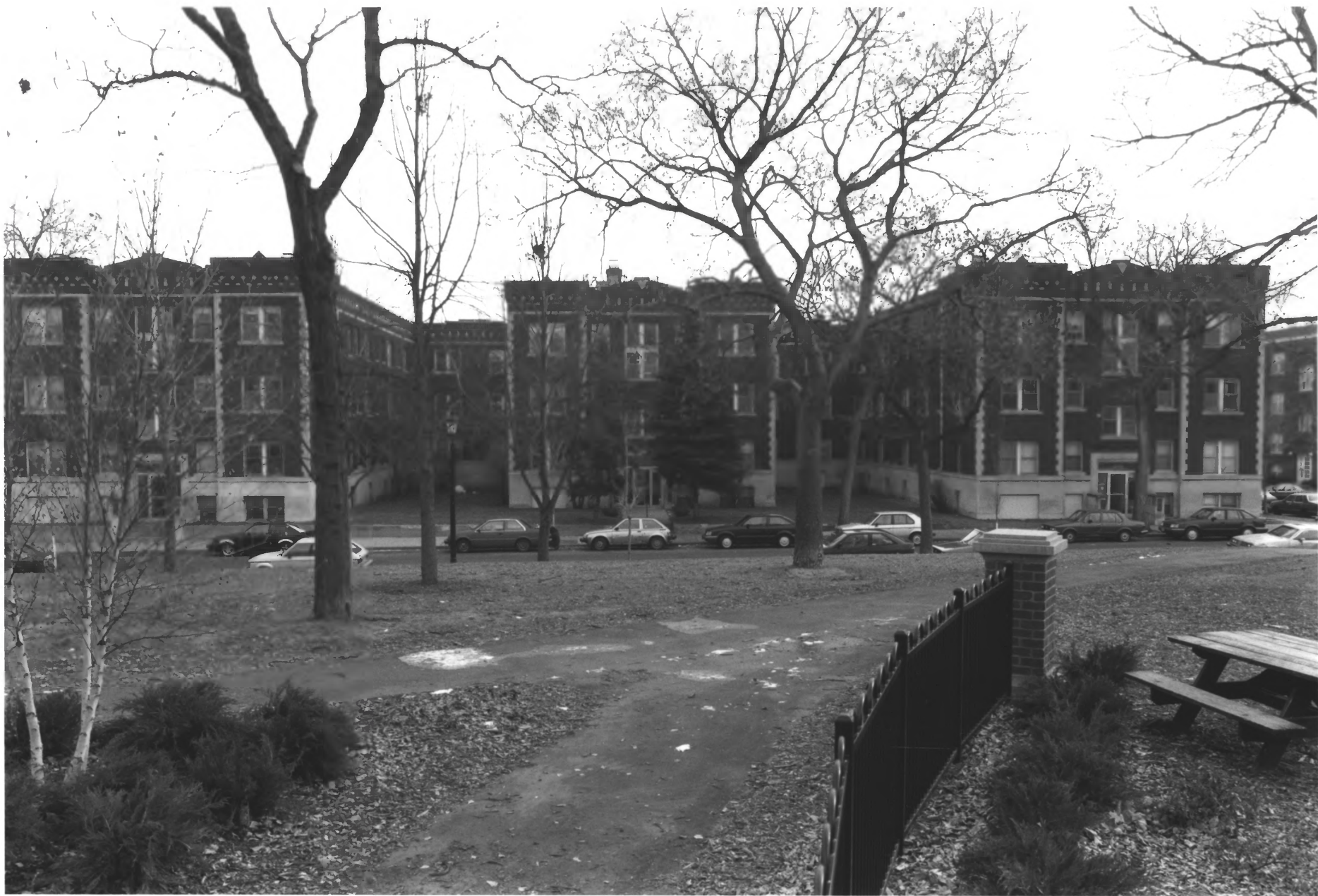
THE VESTA - 1817-25-31 2ND AVE. S. STEVENS SQUARE HISTORIC DISTRICT MINNEAPOLIS, HENNEPIN CO., MINNESOTA #011515-12
