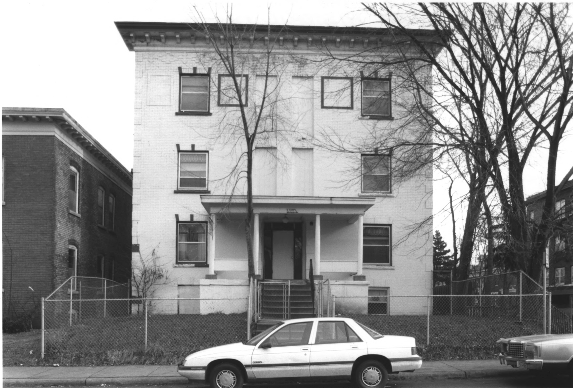
THE SHERWOOD FLATS - 1915 1 ST AVE. S. STEVENS SQUARE HISTORIC DISTRICT MINNEAPOLIS, HENNEPIN CO., MINNESOTA #011513-5A
