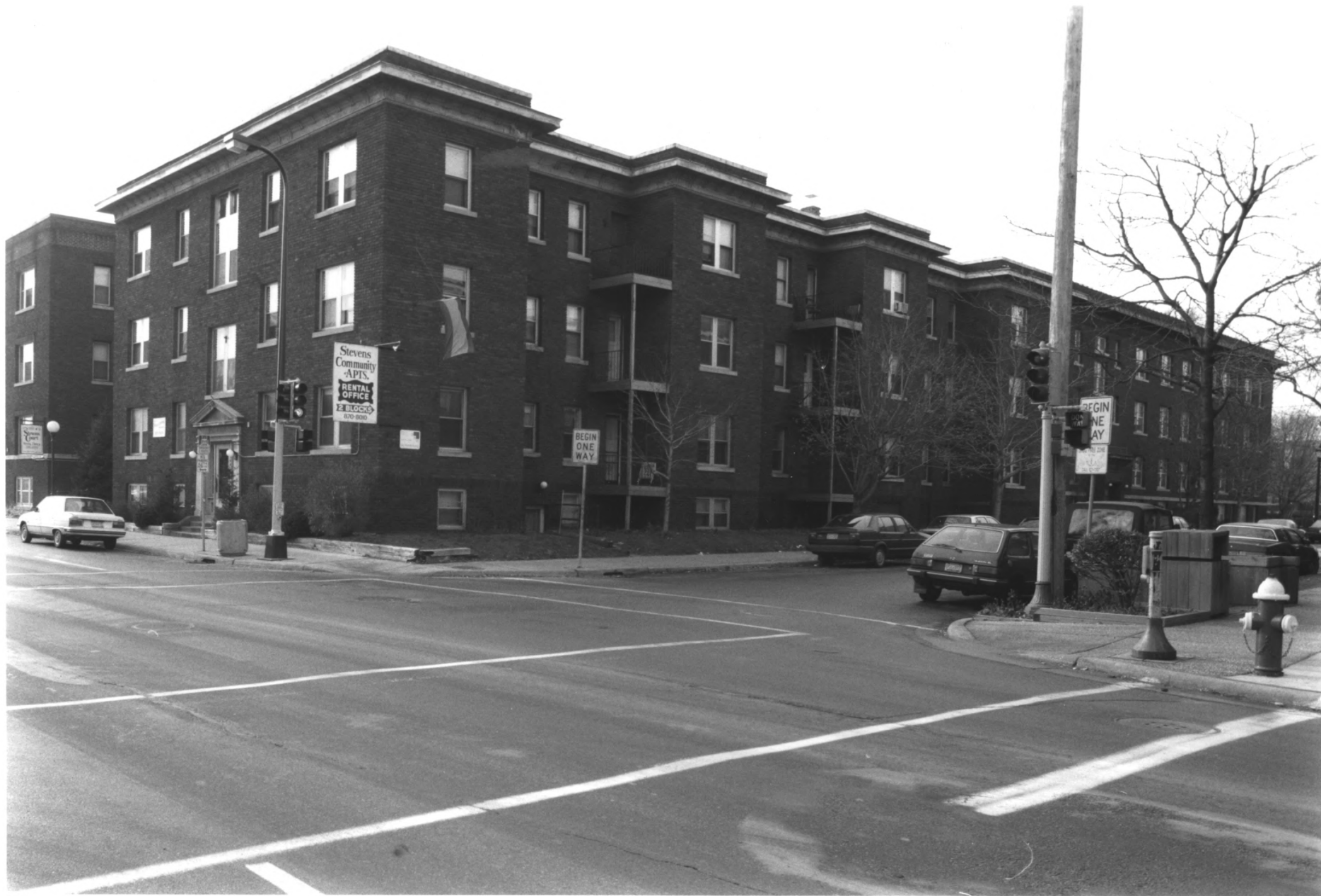
THE REXOR-1800 3RD AVE. S. STEVENS SQUARE HISTORIC DISTRICT MINNEAPOLIS, HENNEPIN CO., MINNESOTA #011516-6A
