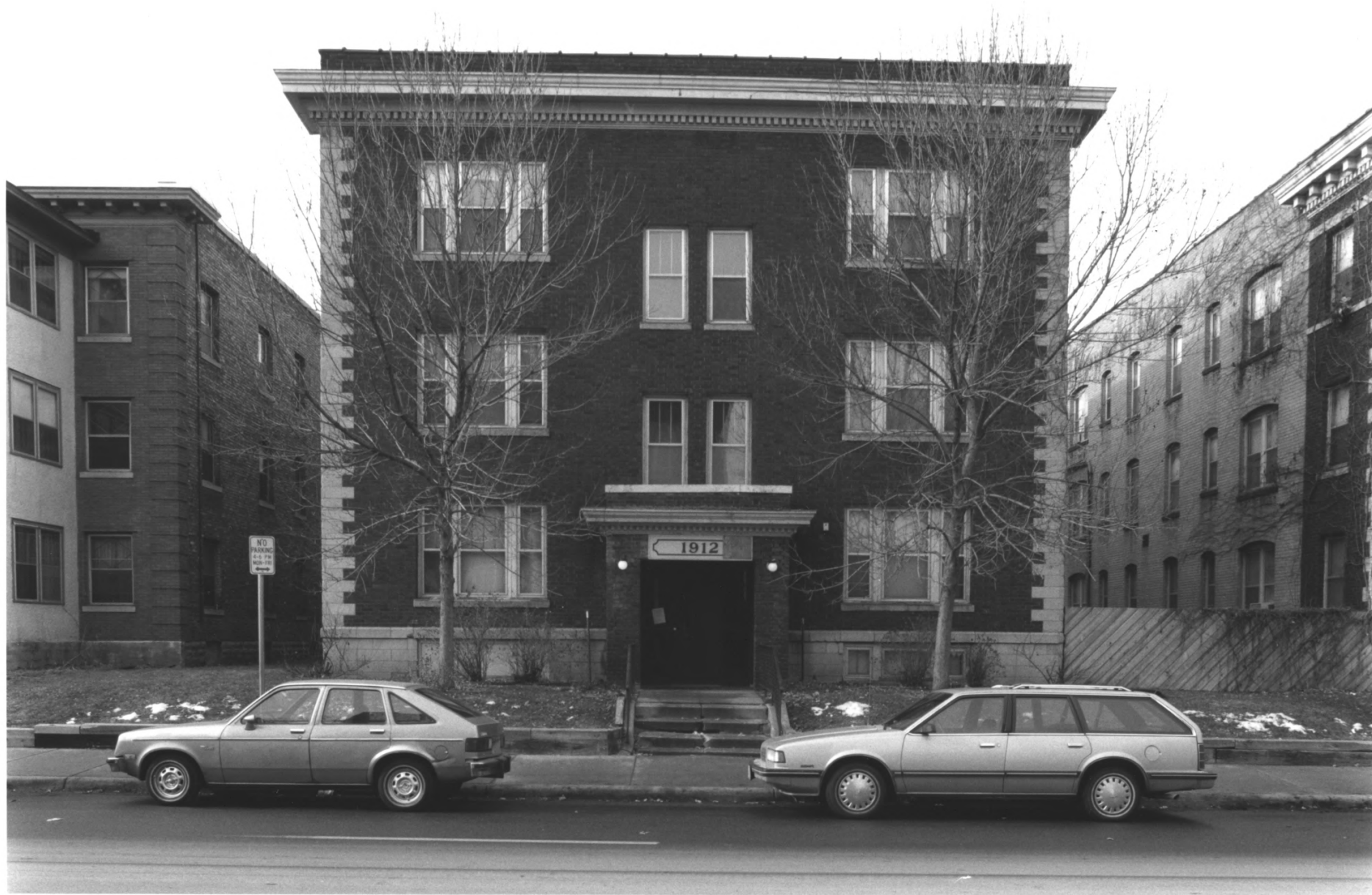
1912 3RD AVE. S. STEVENS SQUARE HISTORIC DISTRICT MINNEAPOLIS, HENNEPIN CO., MINNESOTA # 011516-17A
