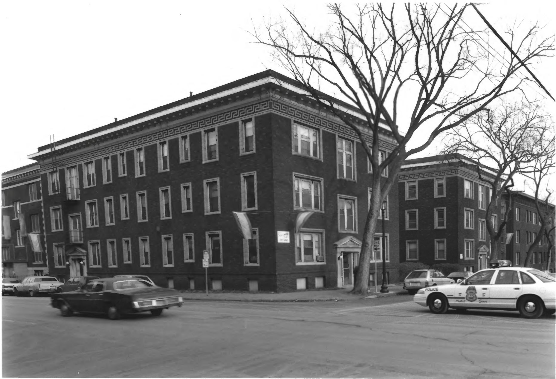
STREETSCAPE - E. 19TH ST. STEVENS SQUARE HISTORIC DISTRICT MINNEAPOLIS, HENNEPIN CO., MINNESOTA #011513-10A
