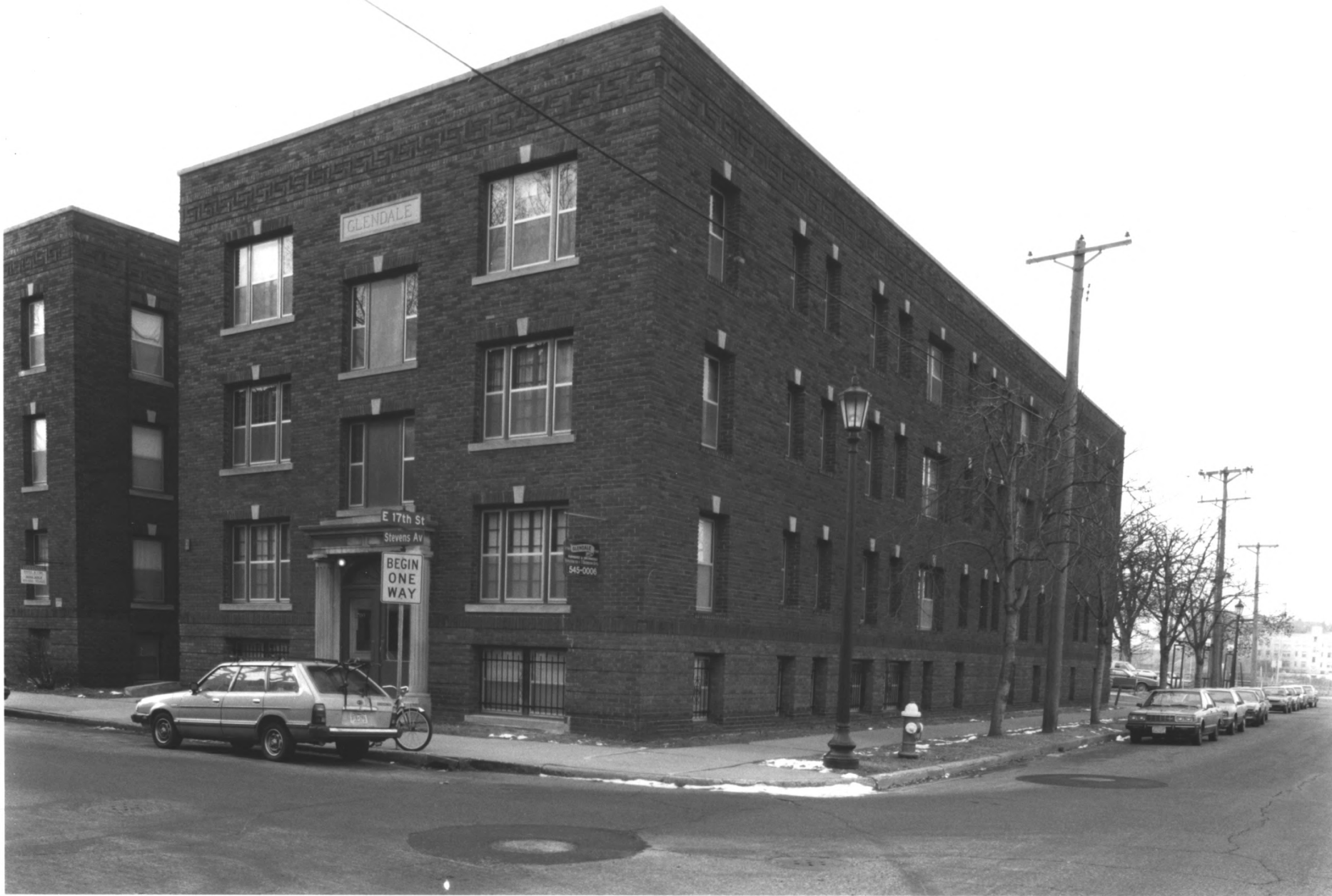
THE GLENDALE - 1700 STEVENS AVE. STEVENS SQUARE HISTORIC DISTRICT MINNEAPOLIS, HENNEPIN CO., MINNESOTA # 011499-11
