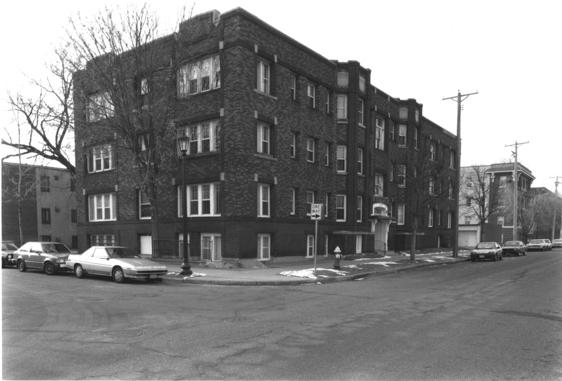
ST. GEORGE APTS. - 137-147 E. 17TH ST. STEVENS SQUARE HISTORIC DISTRICT MINNEAPOLIS, HENNEPIN CO., MINNESOTA #011499-2B
