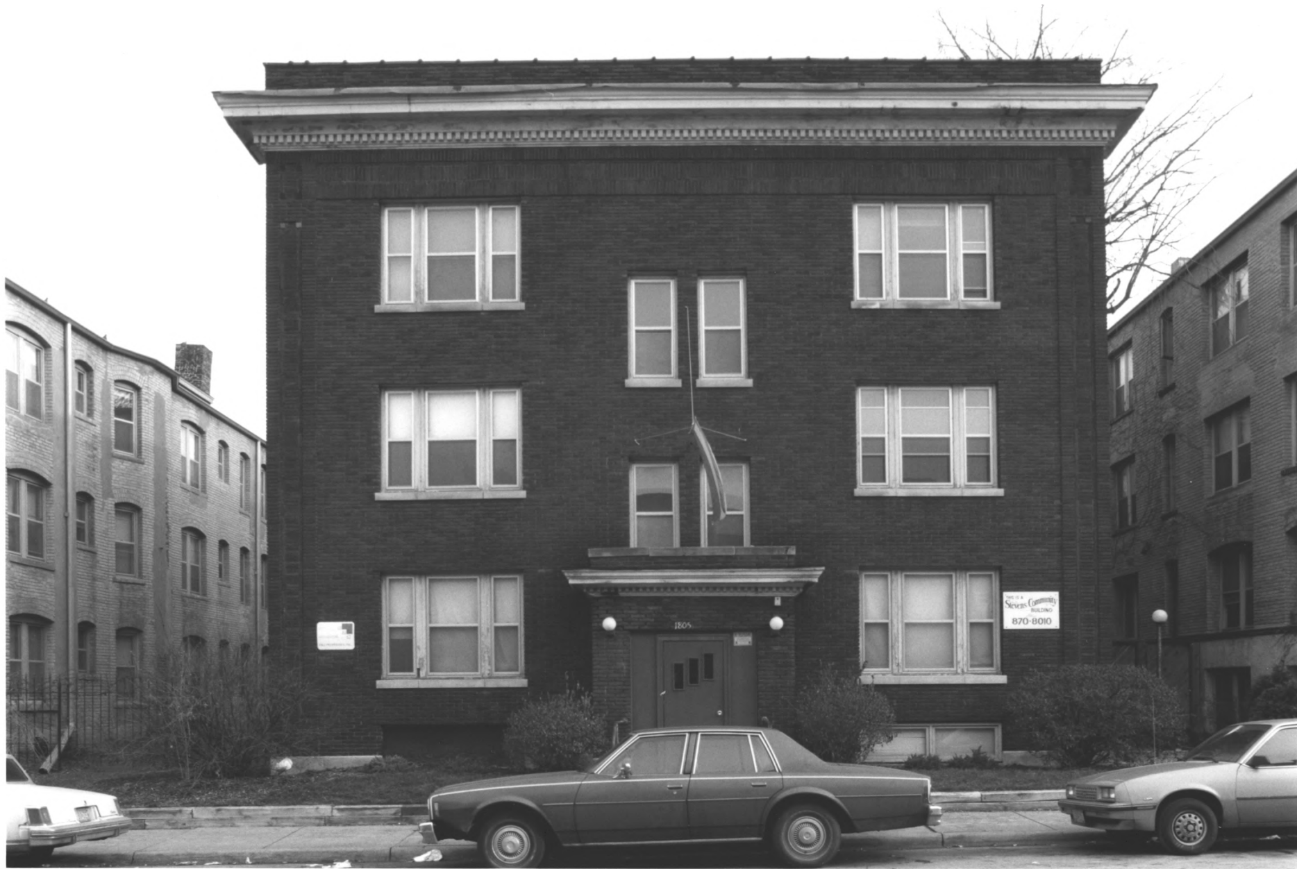
1805 1ST AVE. N. STEVENS SQUARE HISTORIC DISTRICT MINNEAPOLIS, HENNEPIN CO., MINNESOTA # 011513-22A
