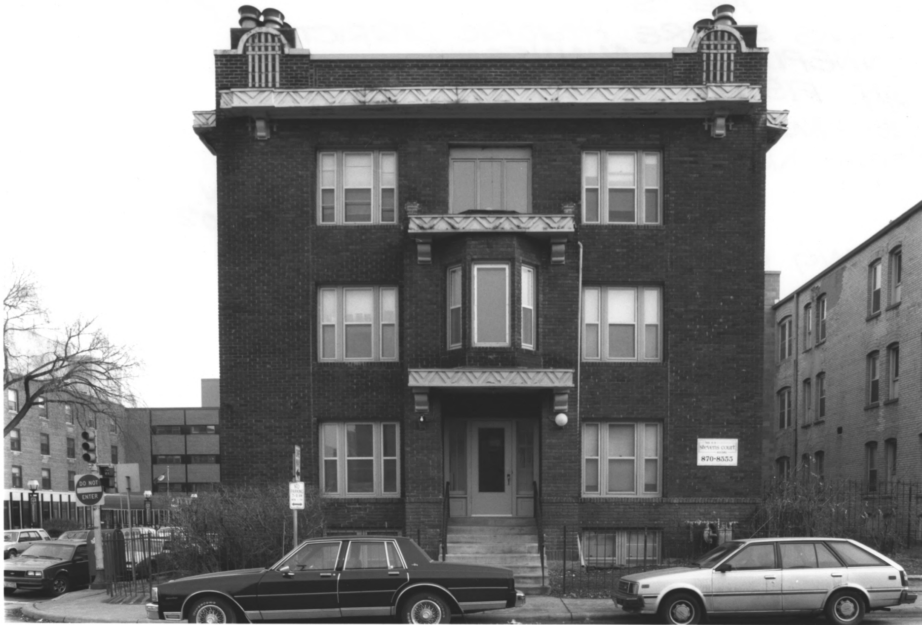
1801 1ST AVE. S. STEVENS SQUARE HISTORIC DISTRICT MINNEAPOLIS, HENNEPIN CO., MINNESOTA #011513-20A
