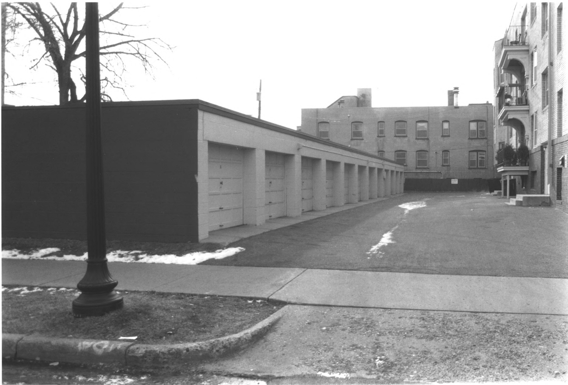
MAUNA LOA GARAGE - 1705-07 STEVENS AVE. STEVENS SQUARE HISTORIC DISTRICT MINNEAPOLIS, HENNEPIN CO., MINNESOTA # 011499-17
