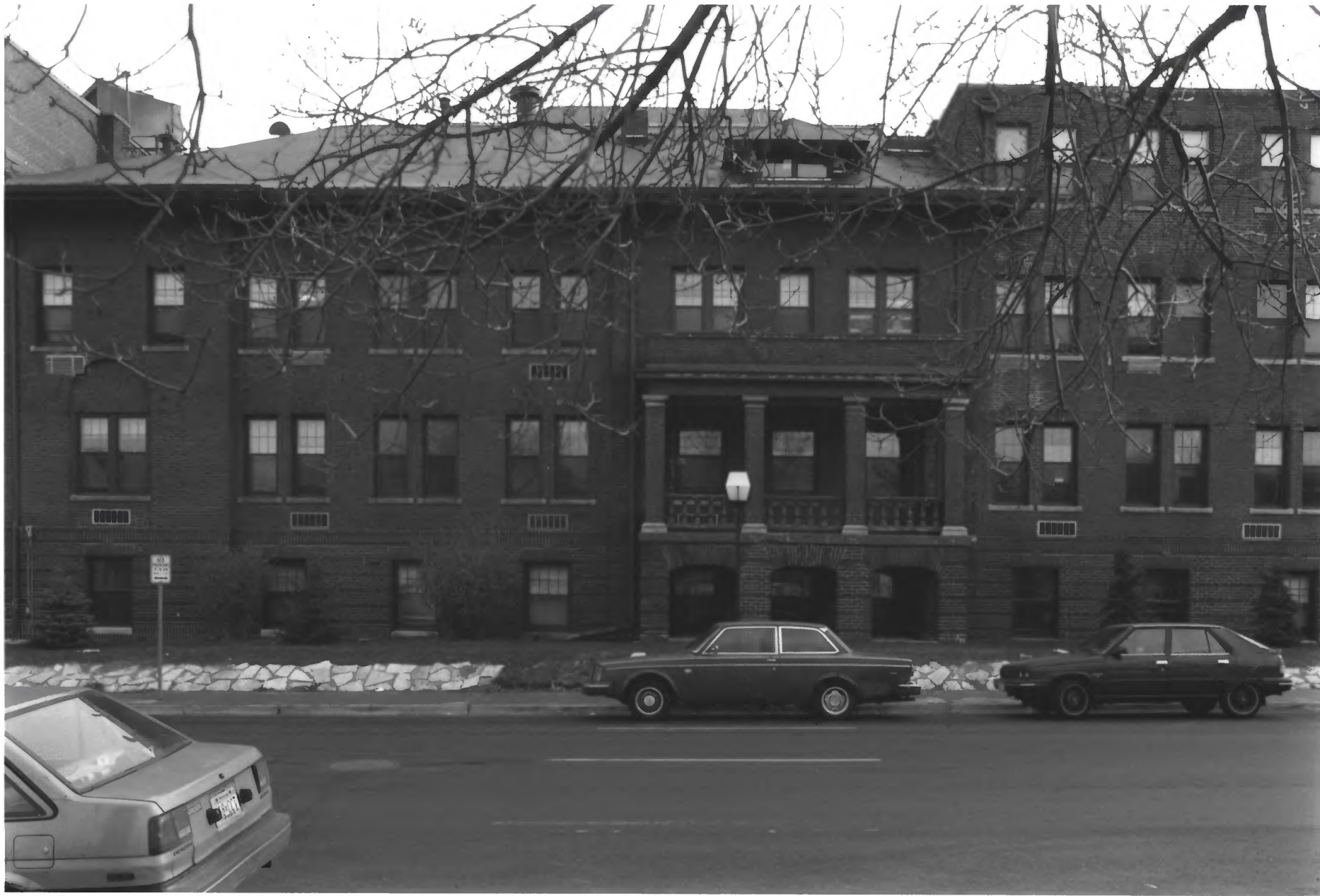
ABBOTT HOSPITAL - 1711-25 1ST AVE. S. STEVENS SQUARE HISTORIC DISTRICT MINNEAPOLIS, HENNEPIN CO., MINNESOTA #011499-8
