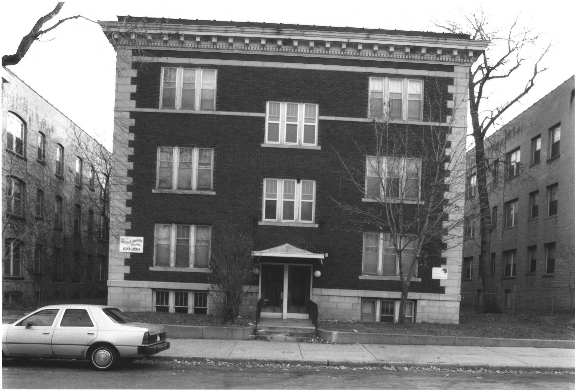
PARKHURST APTS - 1811 2ND AVE. S. STEVENS SQUARE HISTORIC DISTRICT MINNEAPOLIS, HENNEPIN CO., MINNESOTA #011515-9
