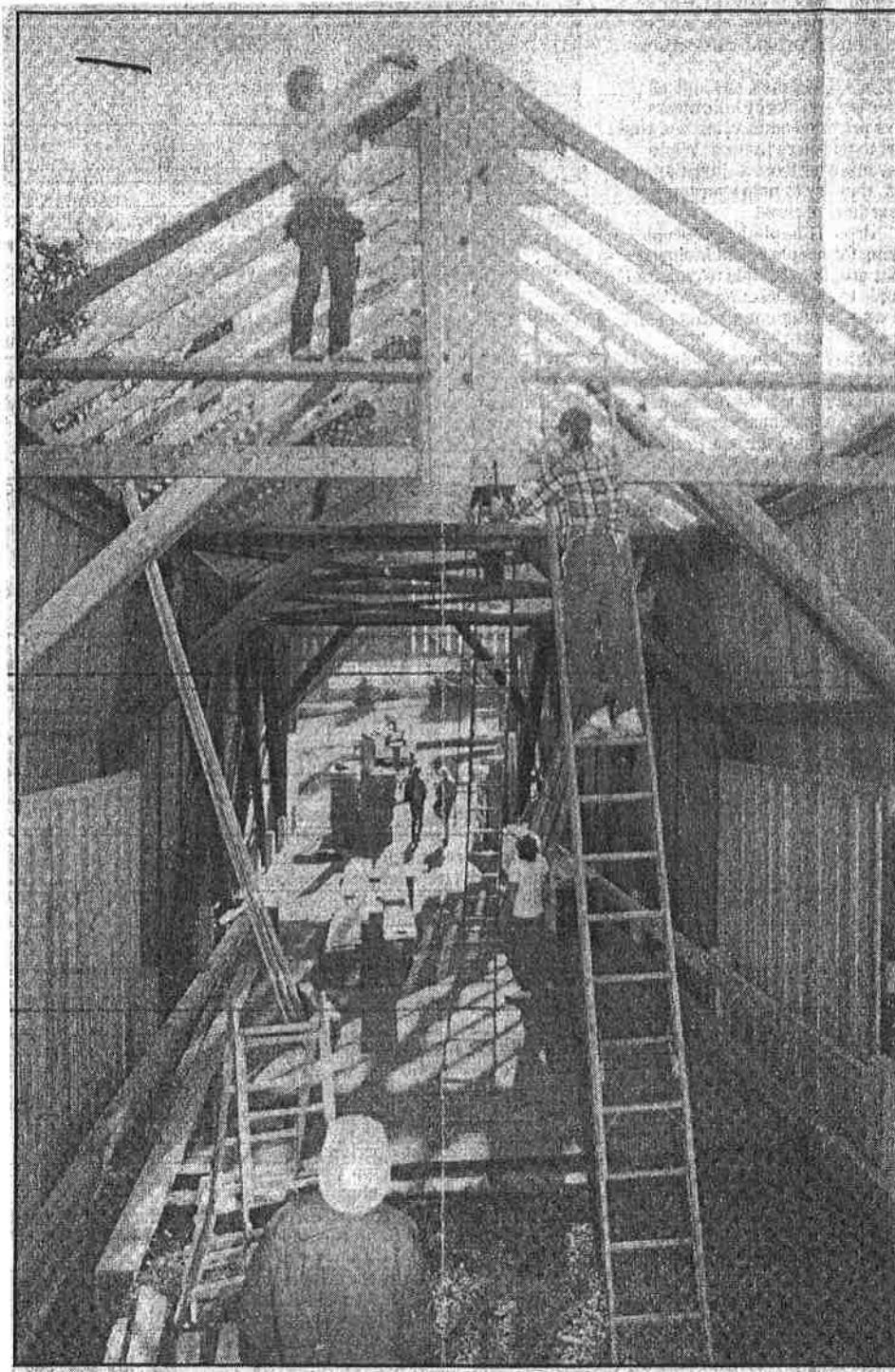
Figure 5: Irish Bend Covered Bridge, Reassembly Process ( Oregonian , 7-Nov-1989)
