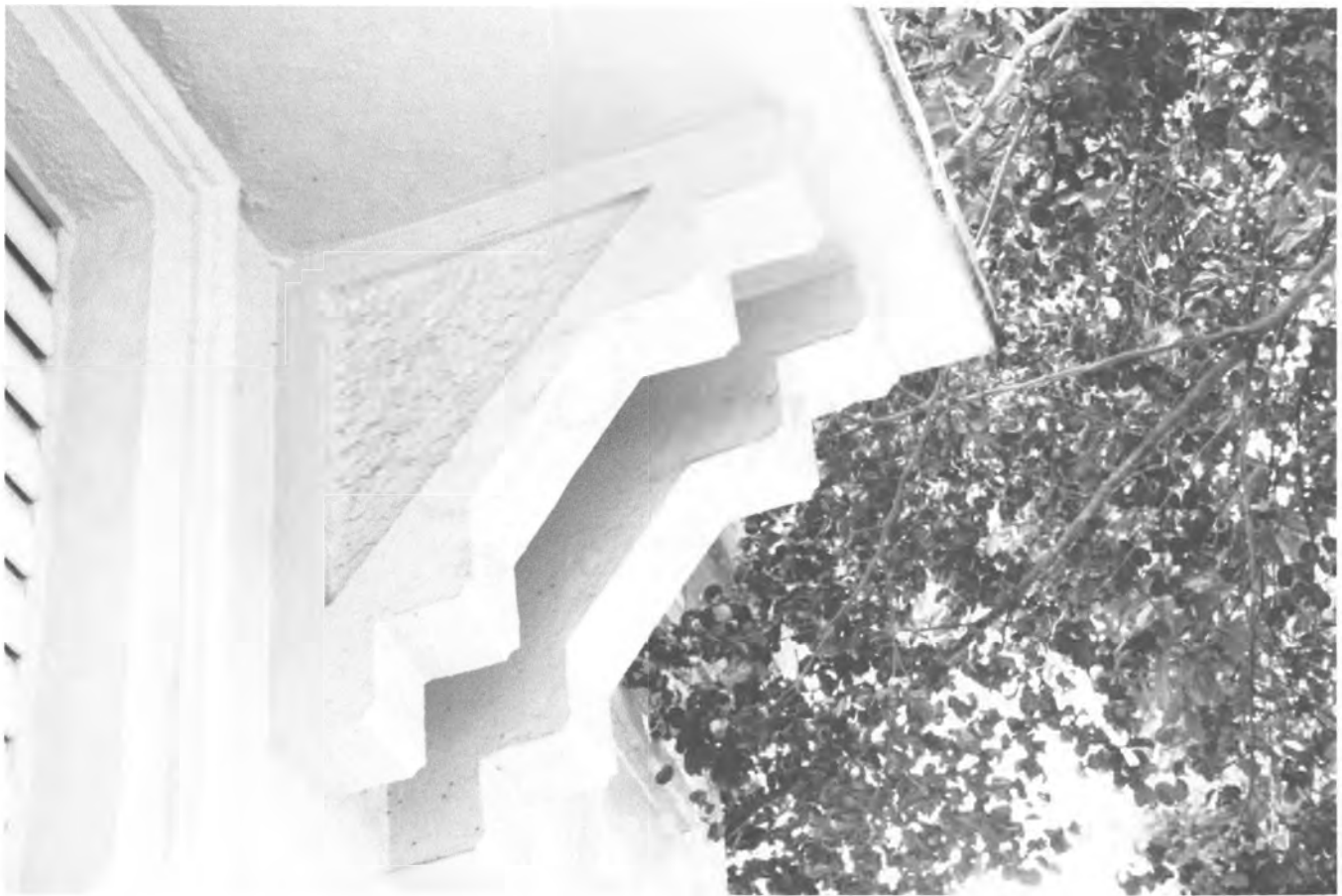
FIG. 13: Mc Kown Jones School closeup detail view, looking southeast, in Villalba, Puerto Rico. Above the window opening, flanking each side, are located two pairs of saw tooth profile brackets. These, in turn, are adorned with triangular sunken panels bearing an exposed aggregate concrete texture. The brackets support a thin, flat concrete slab eave. Above this cantilever, three four-level sunken, tables, bearing exposed aggregate concrete texture in the inner panel appear in alignment with the windows below the awning. Photo: Guillermo Marrero, June 01, 2012. Source: Jorge Rigau Arquitectos, San Juan Puerto Rico.
