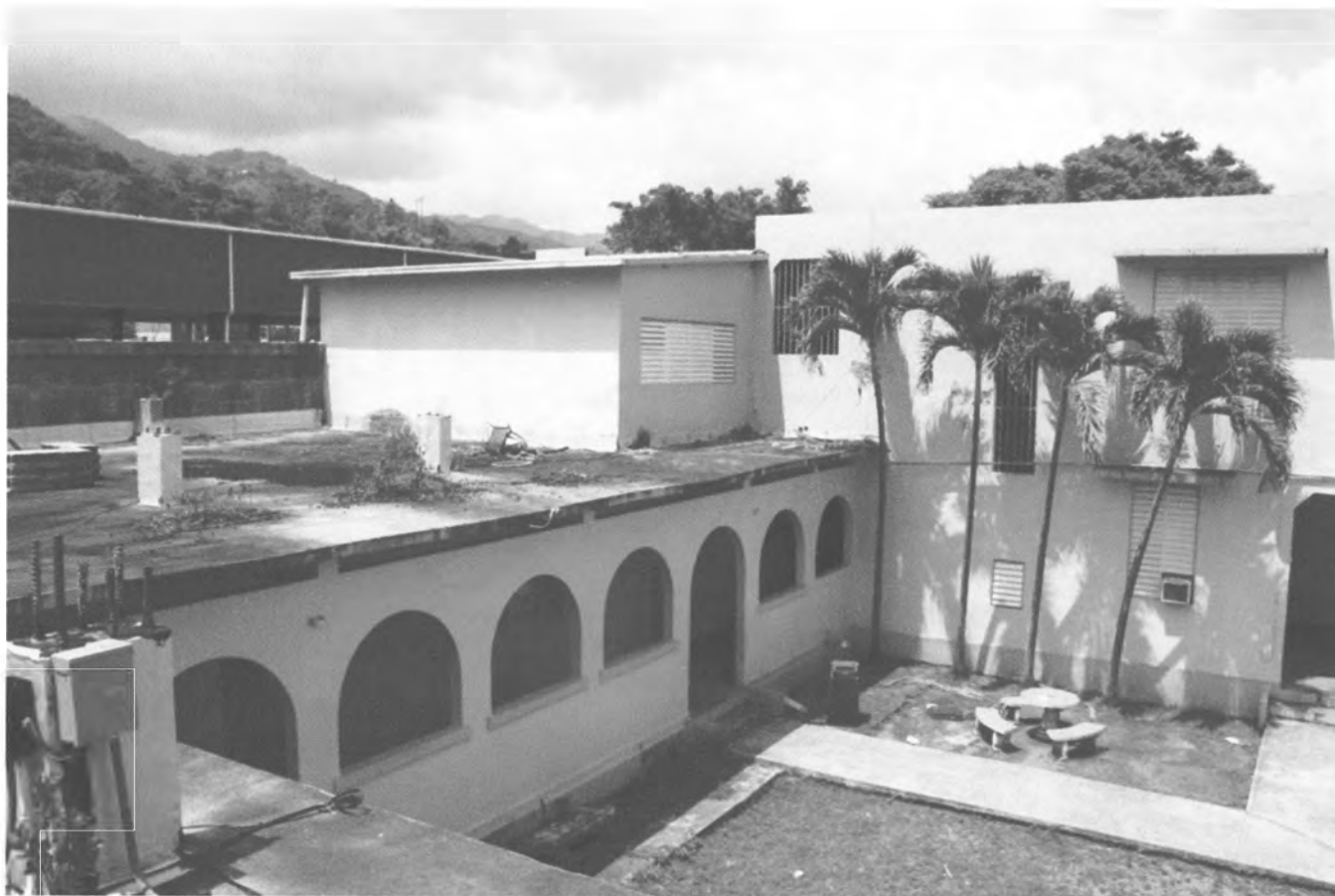
FIG. 15: Mc Kown Jones School interior elevation, looking northeast, in Villalba, Puerto Rico. Seven arches on either side have a solid concrete parapet, while an eighth one allows access to the courtyard. Photo: Guillermo Marrero, June 01, 2012. Source: Jorge Rigau Arquitectos, San Juan Puerto Rico.
