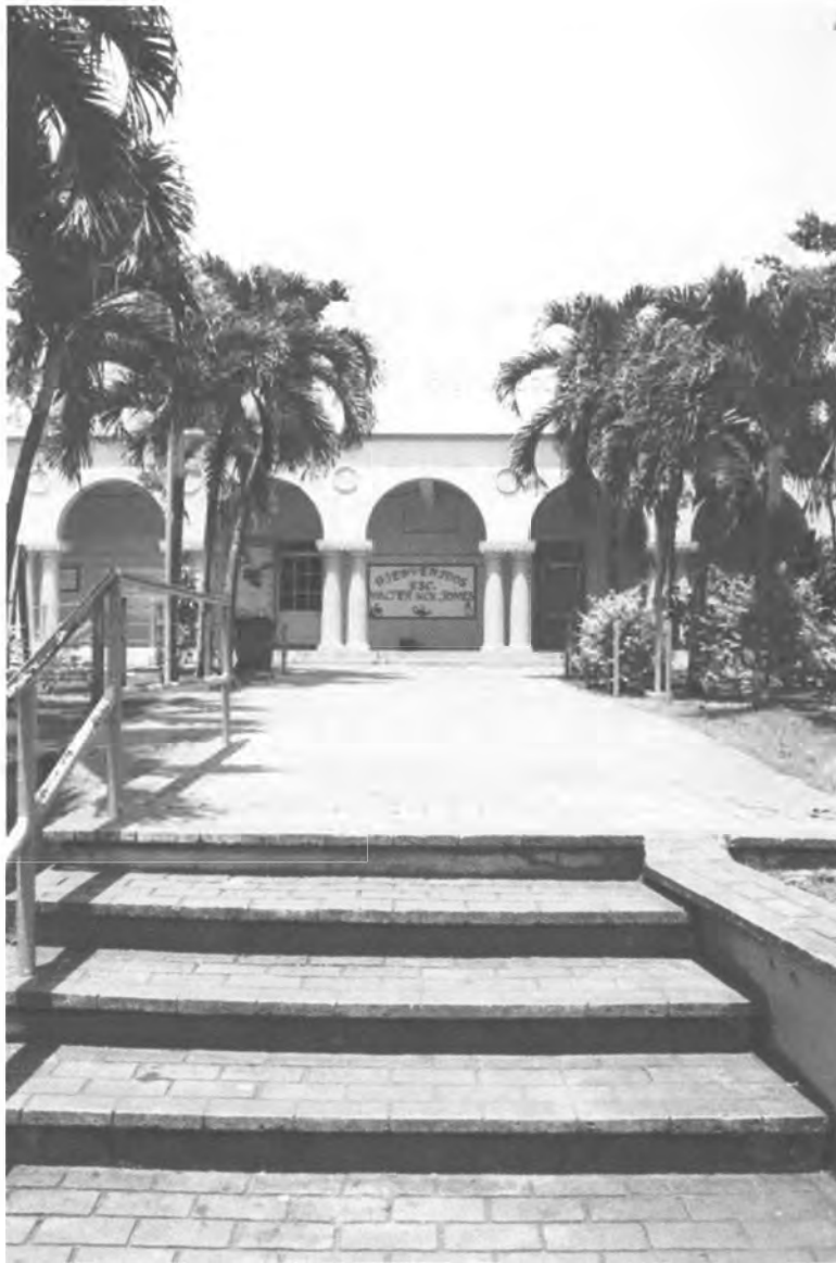
FIG. 3: Walter Mc Kown Jones School west elevation, looking east, in Villalba, Puerto Rico. The stairs are 7'-4" wide, built in reinforced concrete. Both steps and ramp mediate the height difference between the sidewalk and the School's patio. The stair risers are cement-plastered with paint while the treads, as well as the ramp and access path from entrance towards the building, are covered with concrete pavers. Photo: Guillermo Marrero, June 01, 2012. Source: Jorge Rigau Arquitectos, San Juan Puerto Rico.
