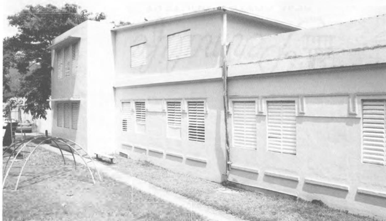
FIG. 16: Mc Kown Jones School north elevation, looking south, in Villalba, Puerto Rico. Originally, each lateral façade included eighteen (18) windows; fifteen (15) arranged in three sets of five, each group corresponding to a classroom. A single window unit provided light and ventilation to the restrooms. Two windows served the offices. At an unknown point of time, the middle opening on each classroom group was sealed up with cement masonry units. Unlike at the office windows, all openings are framed by a connecting/continuous label molding that steps back twice, once as a broad band, the other as a thin strip above the latter. Each unit is underscored by individual windowsill that projects forward twice, once as a broad band, the other as a lean strip below the wide one. On both side elevations, PVC pipes, air conditioning wall units, electrical conduits, electrical service entrance conductors, watt-hour meters and security cameras have been attached carelessly on the surface. A single classroom constructed in the 1980's stands out above the eastern end of the north wing. Photo: Guillermo Marrero, June 01, 2012. Source: Jorge Rigau Arquitectos, San Juan Puerto Rico.
